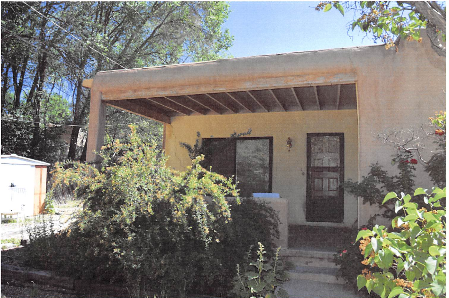
Image 1: The front entry and porch at the west end of the south elevation. The aluminum slider window dates to 1964. The wood-paneled front door dates to circa 2010.
