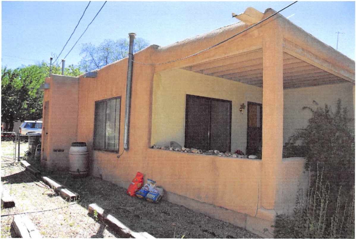
Image 2: SW corner of house and western elevation.
