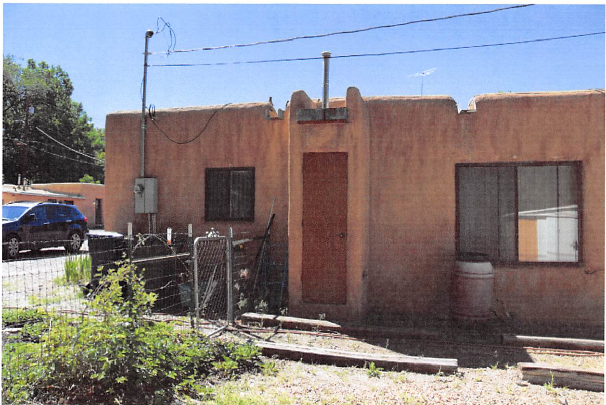
Image 3: North end of western elevation with water closet addition. Parking area at rear is visible in the background.
