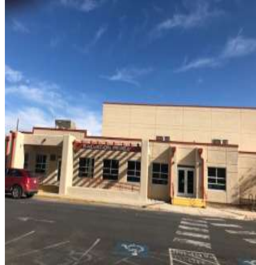
Sal Perez Roof Top Units
