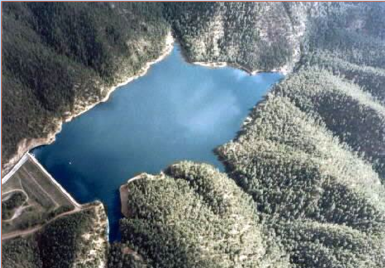
McClure Reservoir on the Santa Fe River
