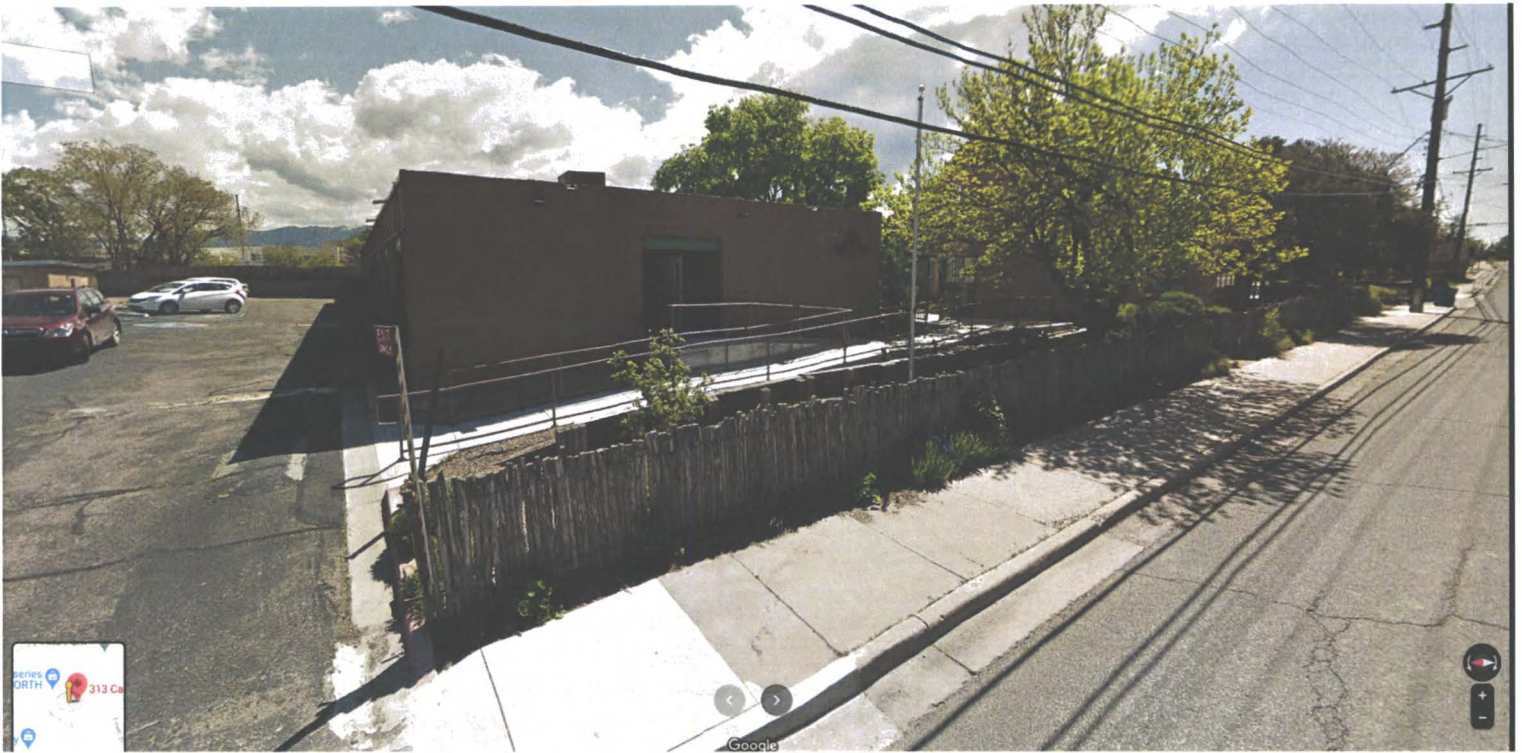
View of 313 Camino Alire from the North. Driveway to the left of the building will be the exit from the property.
