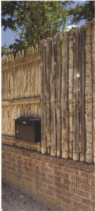
Brick at Frontage Fence
