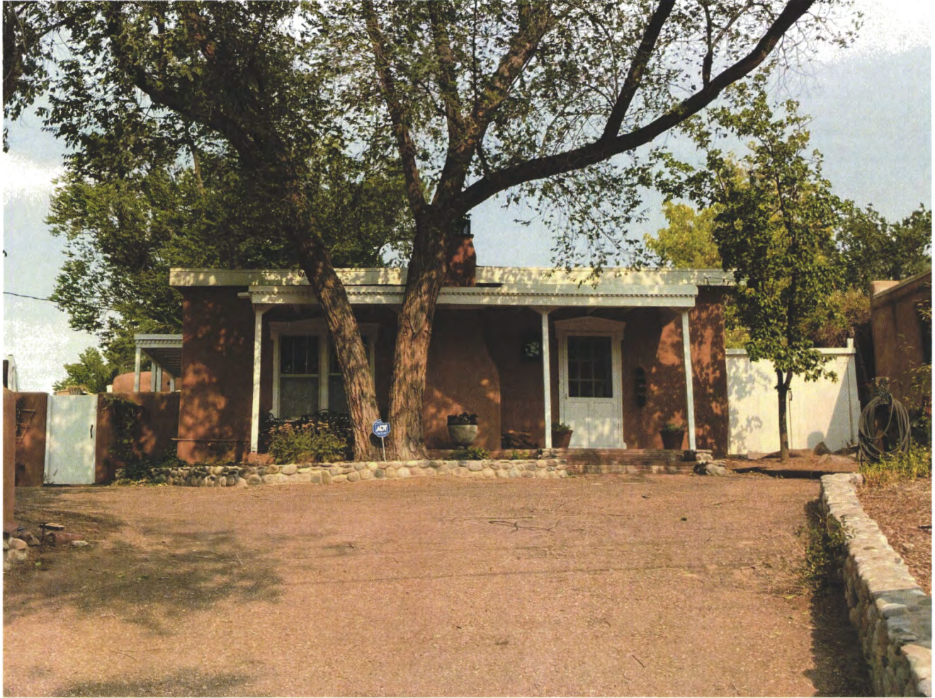
WEST FACING FAÇADE – Existing Residence; “primary façade” as designated by HDRB.
