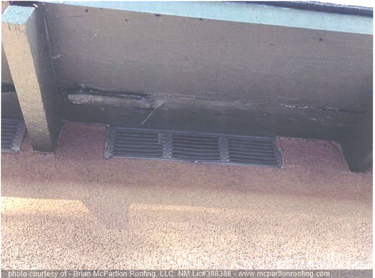
photo courtesy of - Brian McPartlon Roofing, LLC. NM Lic#388388 - www.mcpartlonroofing.com
