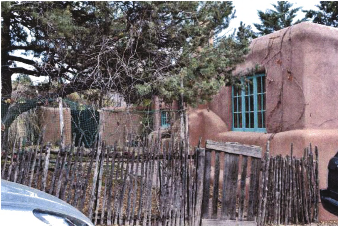
Photo 9: Coyote Fence. Camera facing southwest.
