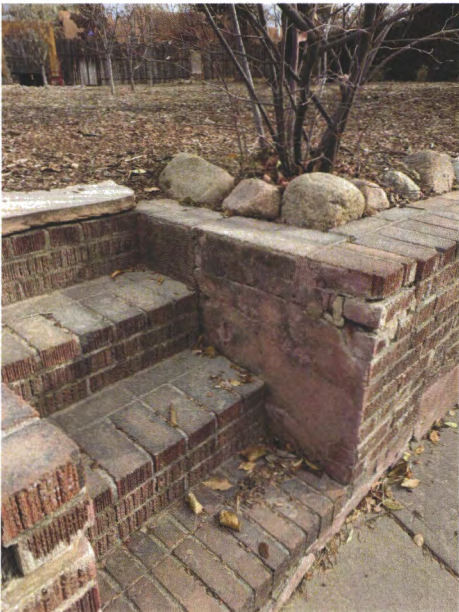
Old Stucco at Driveway Brick
