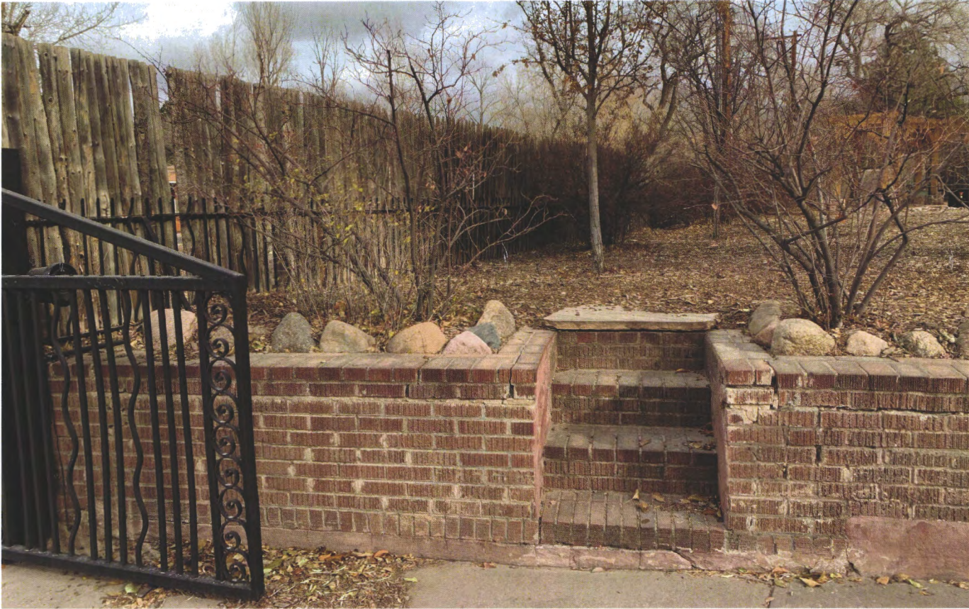
Driveway Brick Wall
