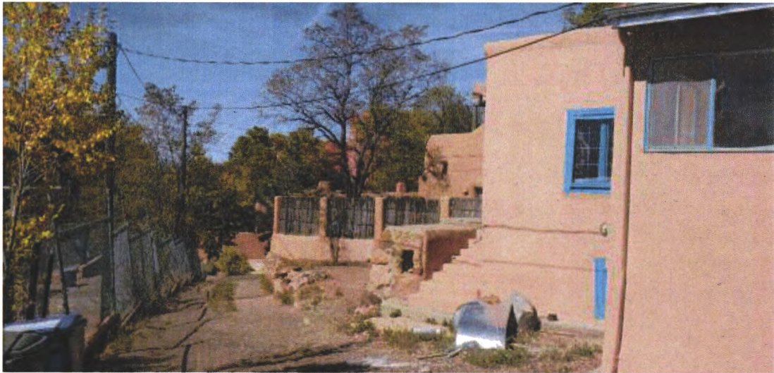
Photo 7: South elevation; 1970s bump-out at right. Camera facing northwest.
