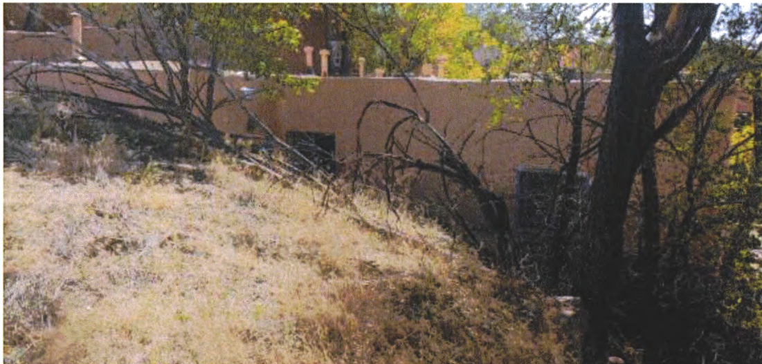
Photo 12: North elevation. Camera facing southwest.
