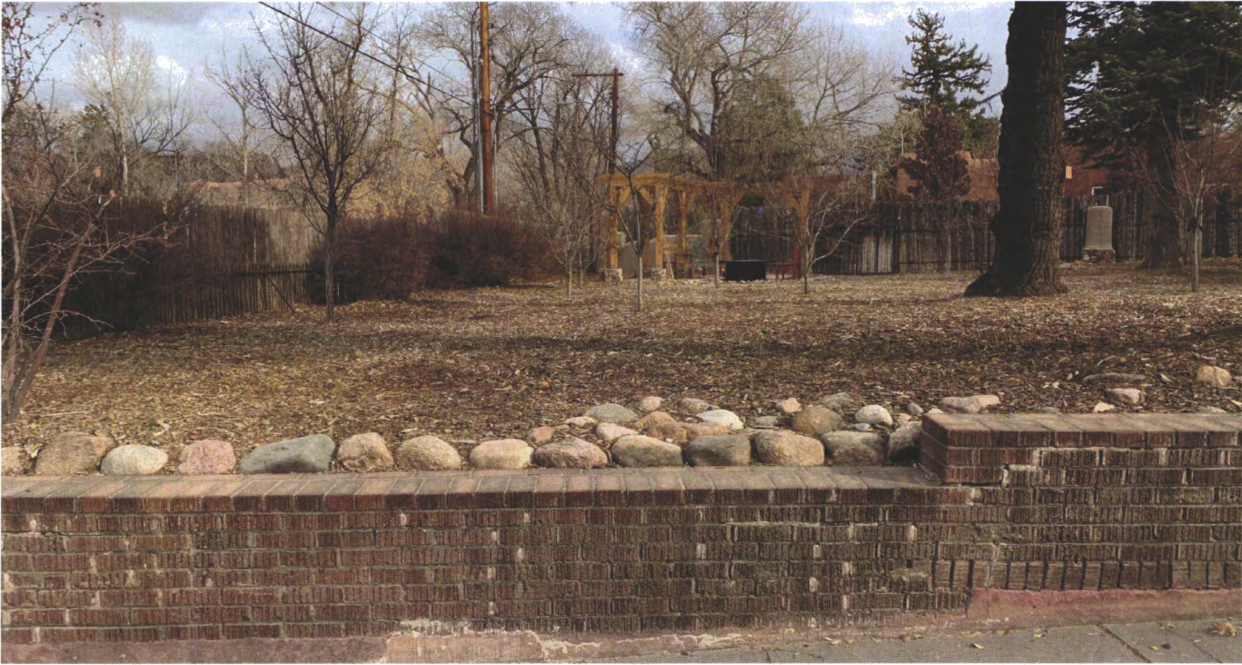
Driveway Brick Wall
