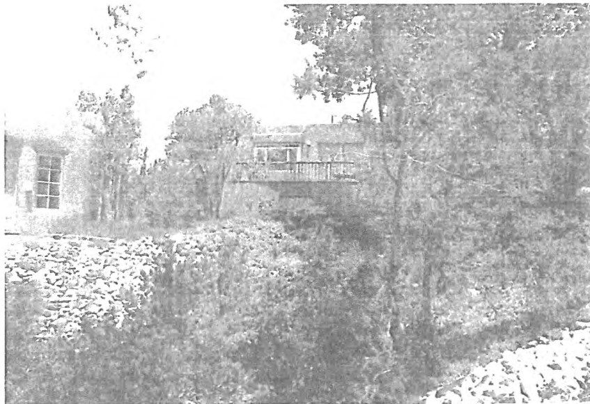
#2 south elevation, west portion
