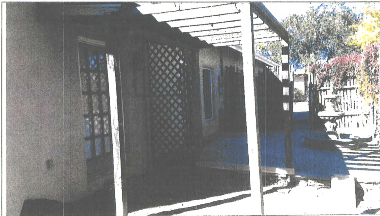
Photo 4 – East Elevation with wood trellis and awning.
