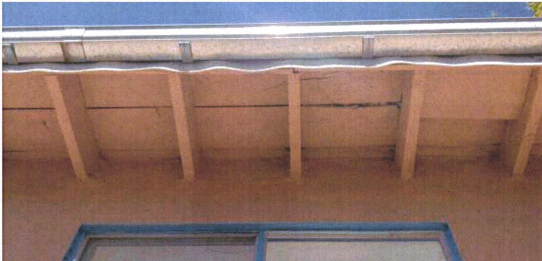
Photo 9: South elevation; 1970s bump-out overhang. Camera facing north.
