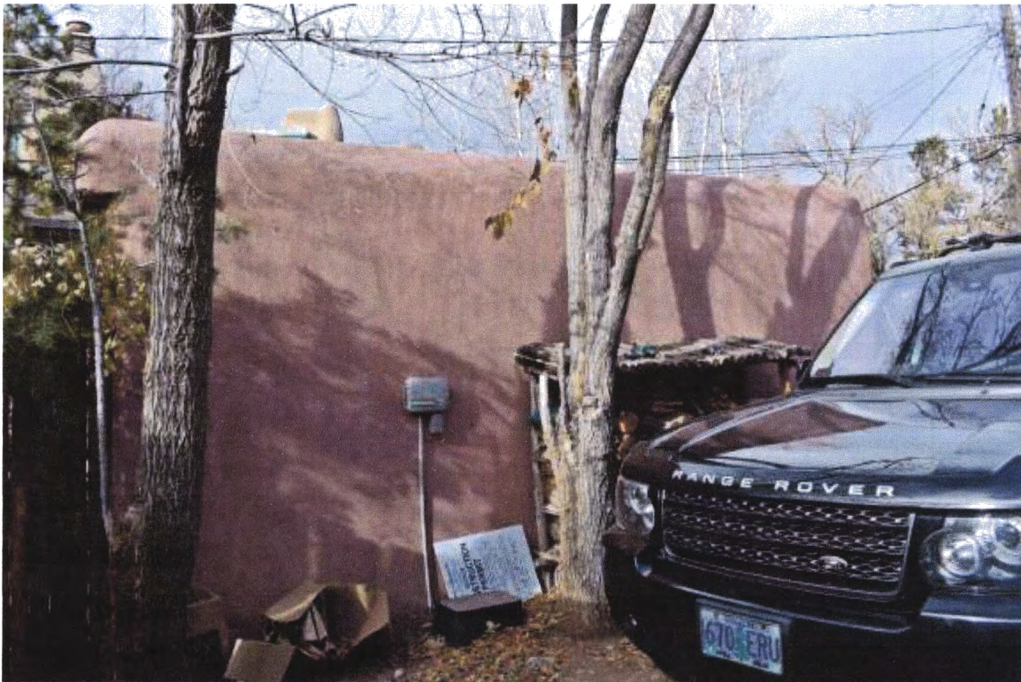
Photo 7: Garage - south elevation. Camera facing northeast.
