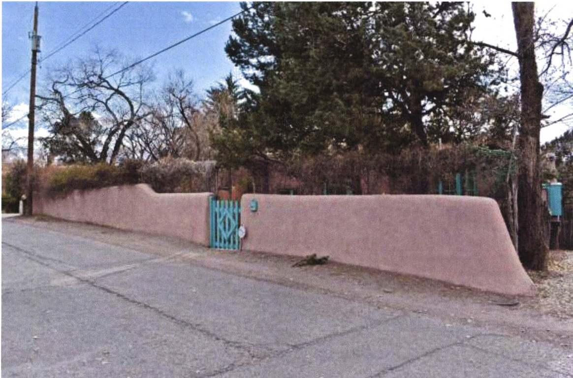
Photo 1: Street Wall. Camera facing southwest.
