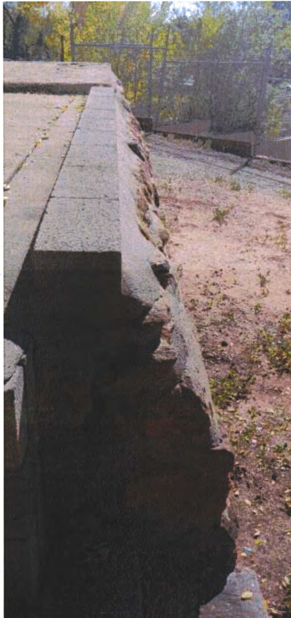
Photo 13: West (front) façade landing; stone cladding. Camera facing southeast.
