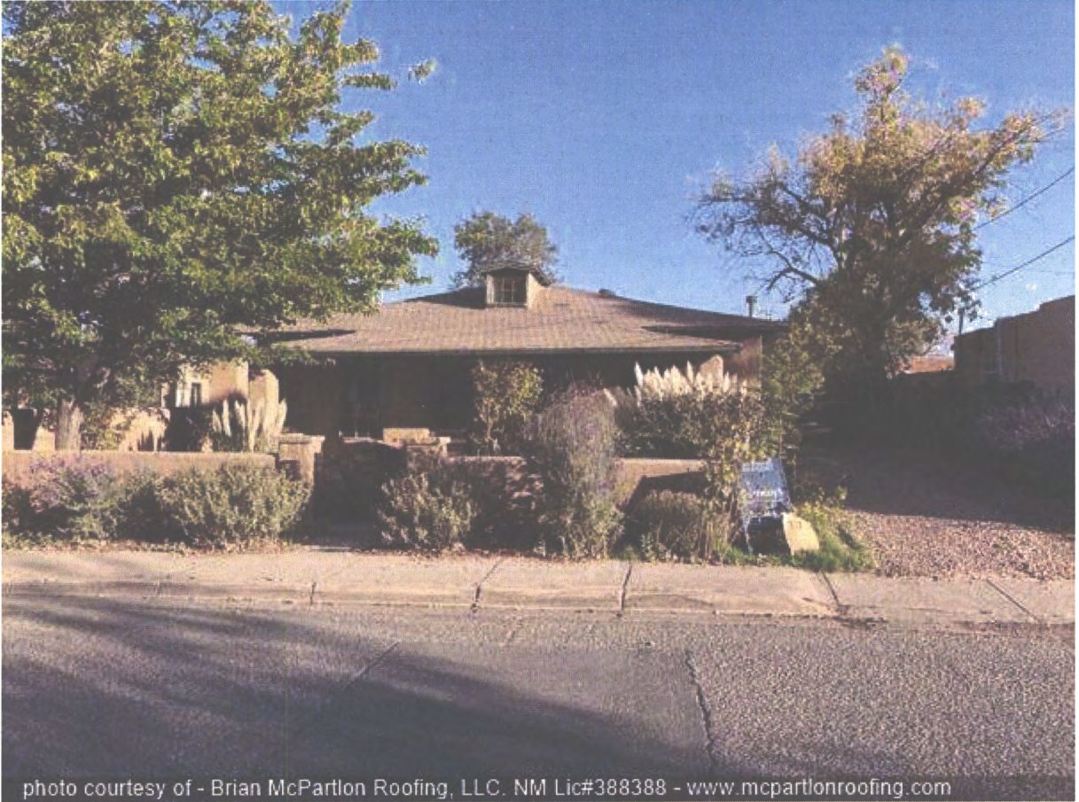
Street frontage – South elevation
