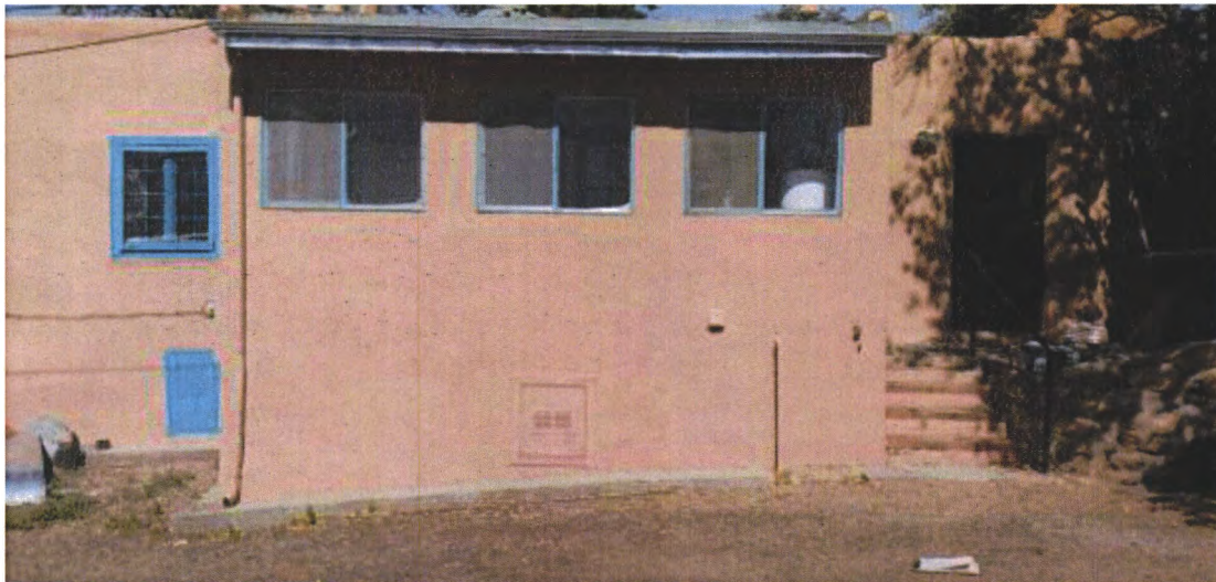
Photo 8: South elevation; 1970s bump-out at center. Camera facing north.
