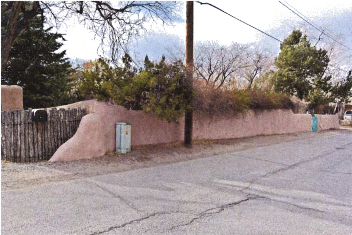
Photo 2: Street Wall. Camera facing northwest.
