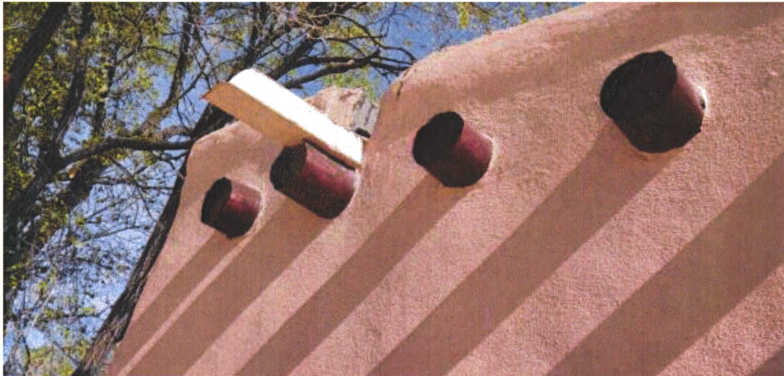
Photo 5: West (front) façade metal vigas. Camera facing northeast.
