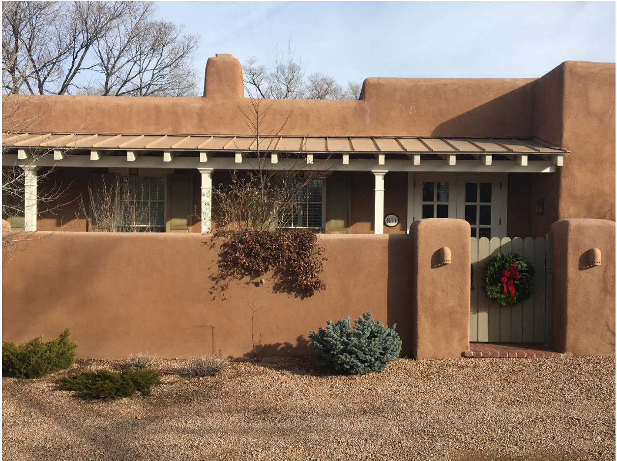
851 Camino Ranchitos (two houses north of subject property)
