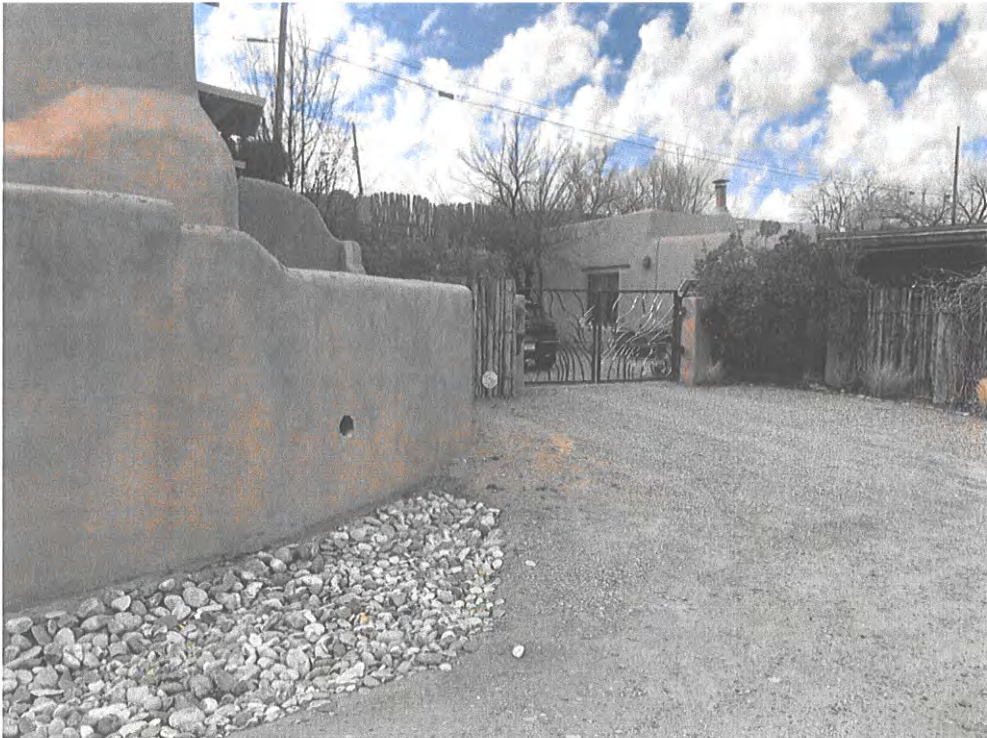
8. Northwest portion of yard wall – looking southwest towards 701 Alto St.
