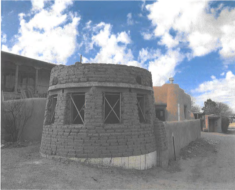
3. East side of adobe studio – looking west down lane
