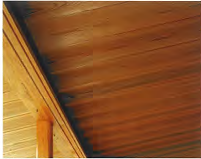
Exposed Exterior Wood: Stained SPF (spruce, pine or fir) with clear sealer:
