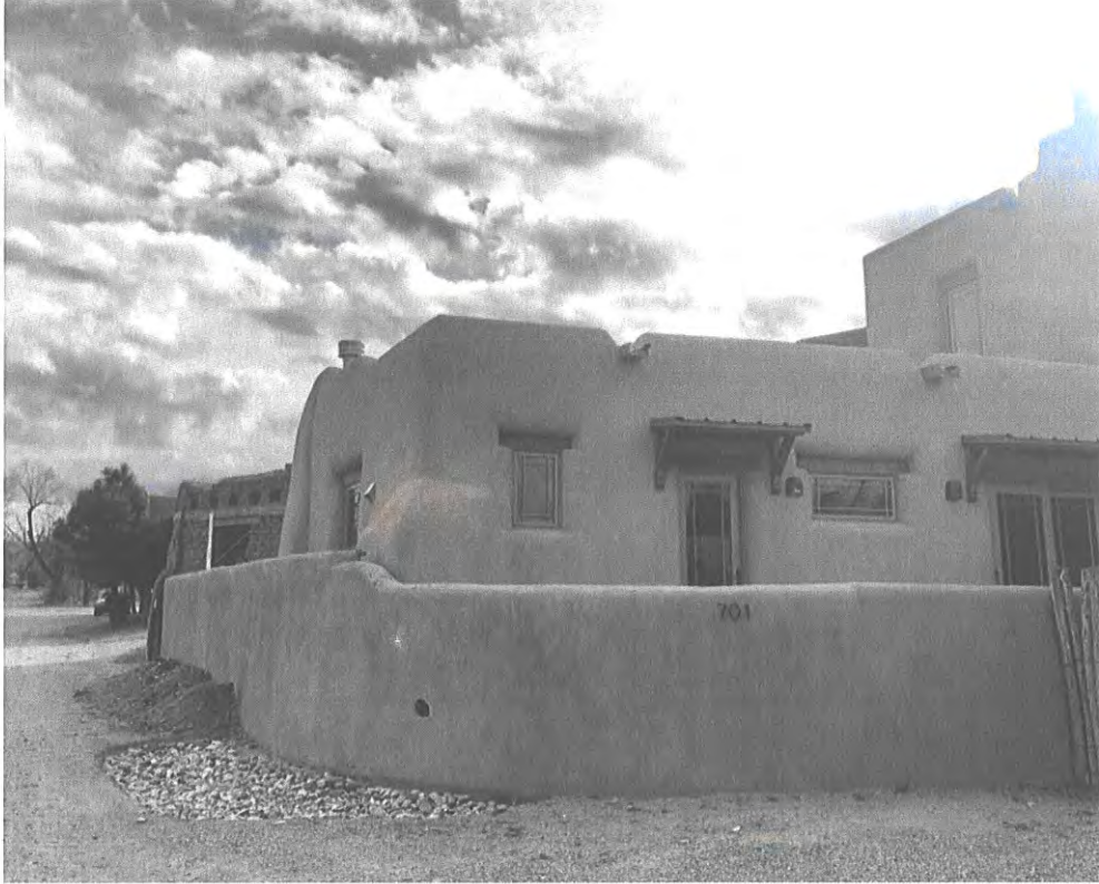
7. North and northwest portions of yard wall – looking east down lane
