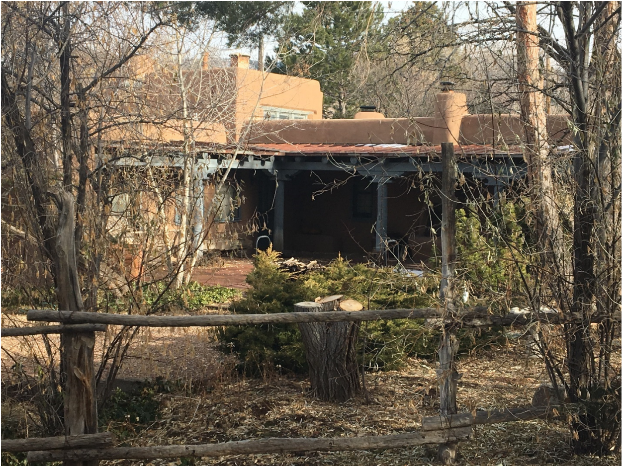
855 Camino Ranchitos (next door neighbor to the south)
