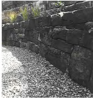
Dry stack Moss rock wall for retaining soil on southwest corner of the property & for northeast corner of the property
