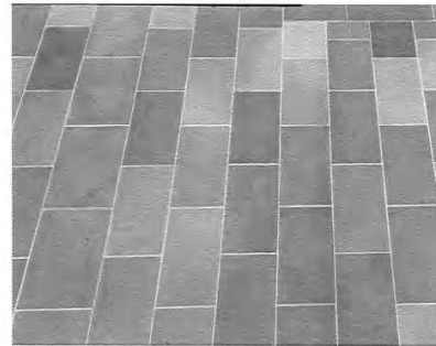
Bluestone Rectangular pavers for Courtyard and all Portals and caps on Entry Bench, Guest Portal half wall, and Grill area walls.
