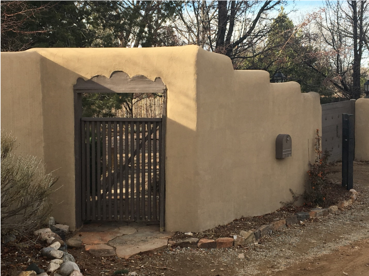
854 Camino Ranchitos (opposite side of the street, just a bit south from subject property)
