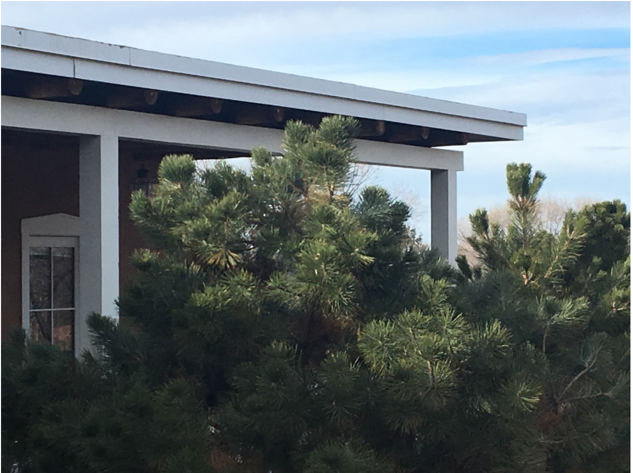
858 Camino Ranchitos (portal detail)
