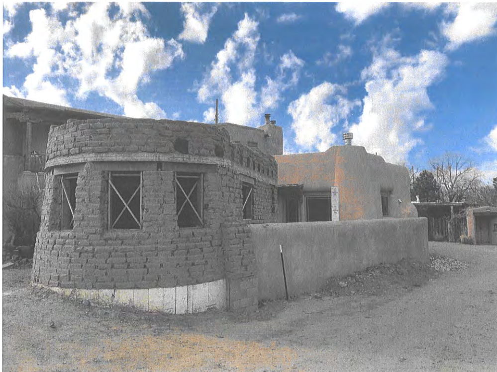
4. Northeast side of adobe studio and connected yard wall – looking southwest
