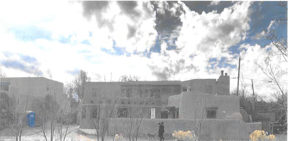
2. North side of adobe studio and yard wall – looking south from W. Alameda St.
