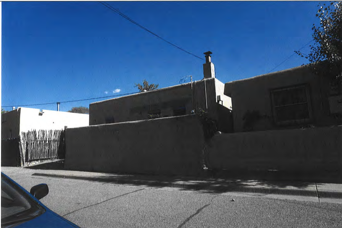
North Elevation from Alto Street, note the shadow of the removed porch.
