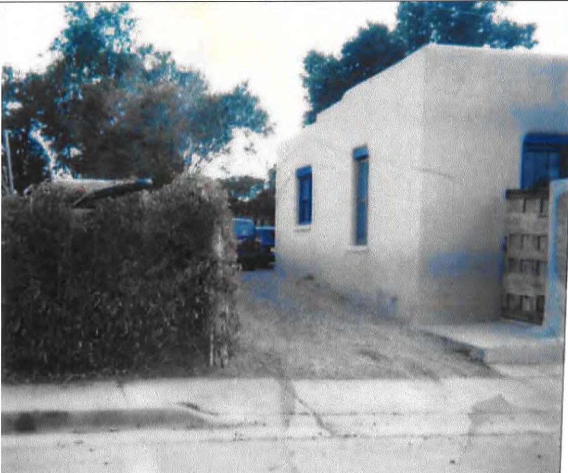
Photograph from Case # H-87-141 801 Alto, City of Santa Fe. Note new wall and gate. Original Windows.
