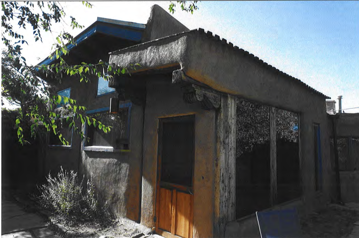
Rear addition, post 1987, with filled in porch, shed roof, exposed vigas and decking, corbels, wood fixed windows.
