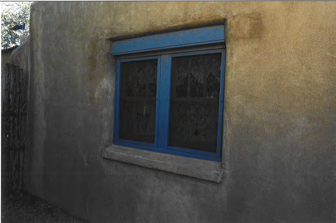
East facing wood windows, 3/1 tandem, also with wood lintel (original replaced?) and concrete sill
