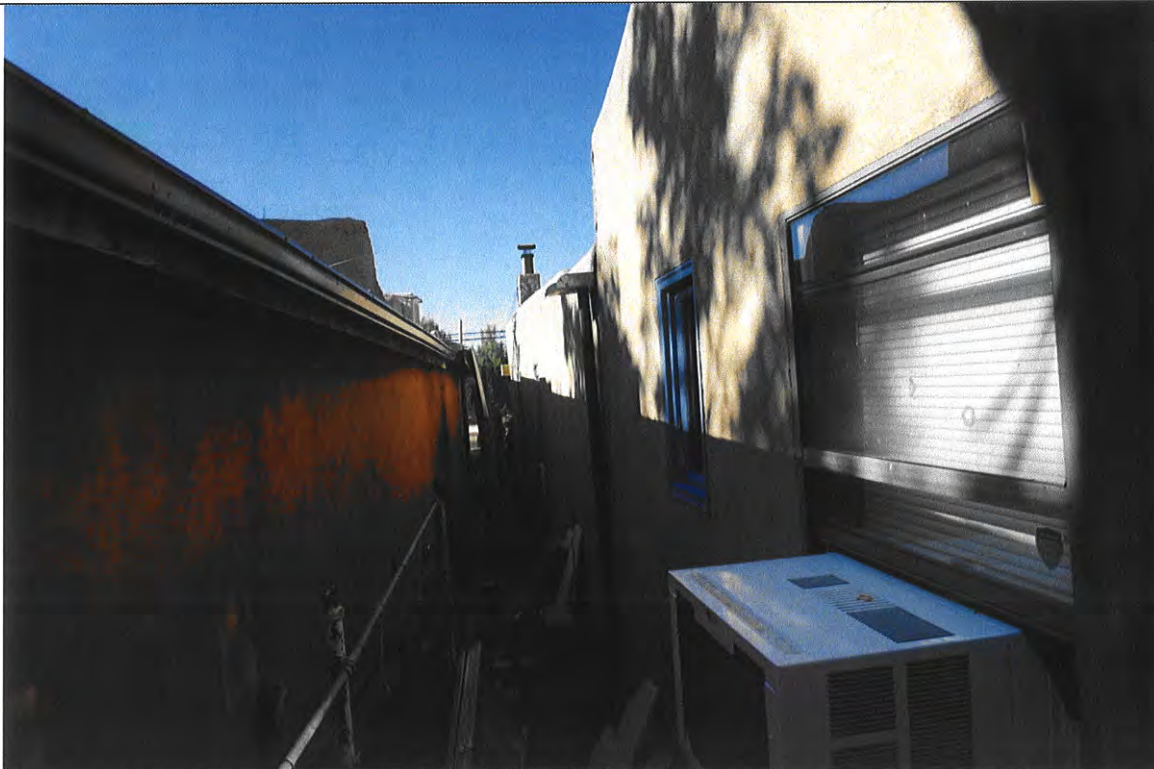
West façade from the south yard with aluminum SH window, wood casement, and two original 3/1 wood windows at the north end, metal canale, and chimney.
