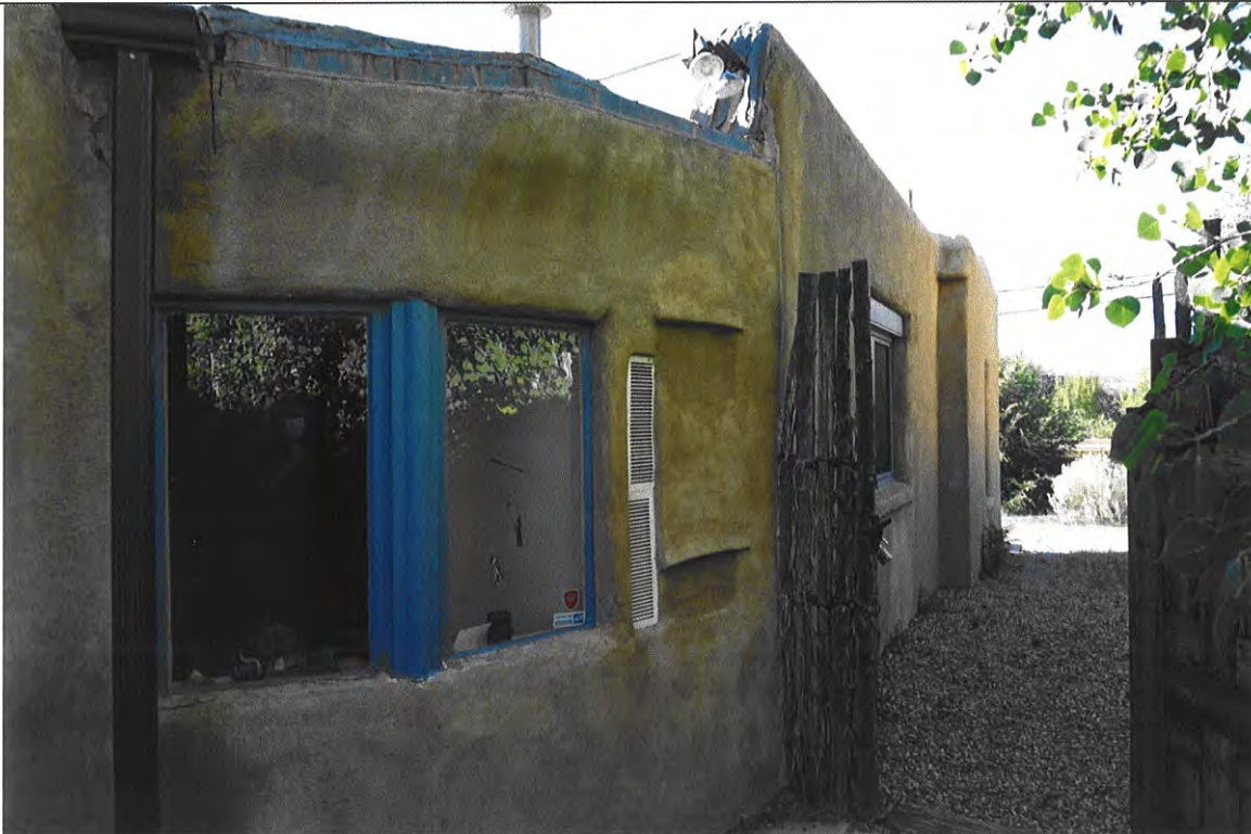
East façade looking north show the rounded porch filled in, the stepped parapet, and canal and downspout off of roof of original mass.
