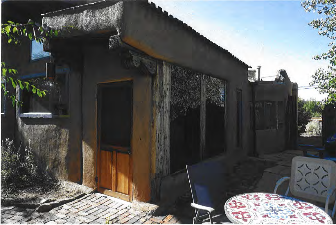
South view of rear addition showing old porch filled in
