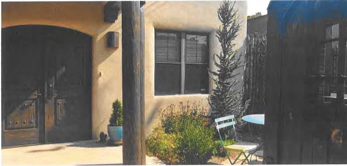
Photo 4: South, front façade, entry door and east window. Camera facing northeast.
