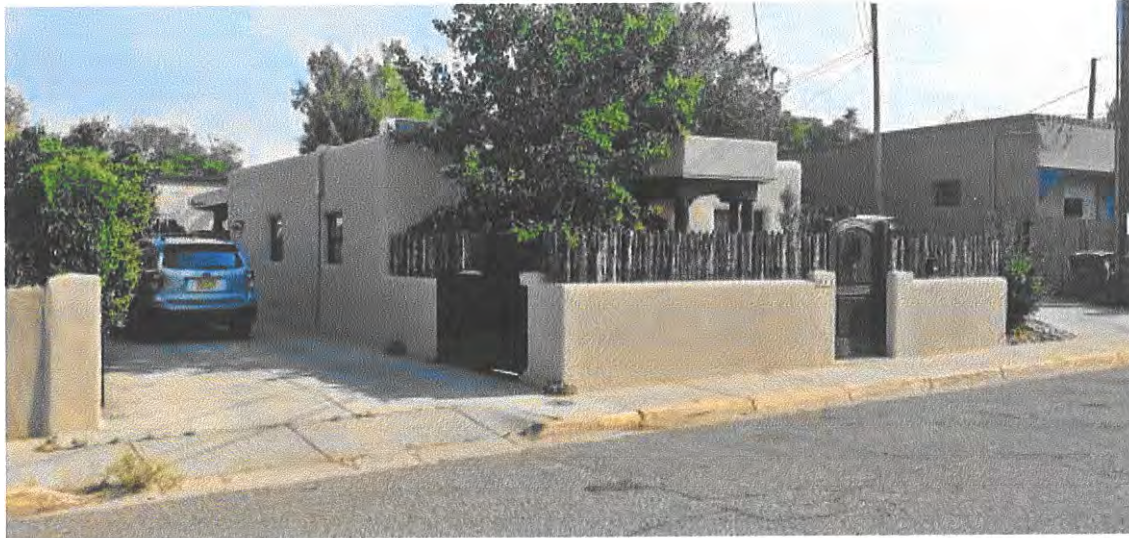
Photo 5: West elevation. Camera facing northeast.
