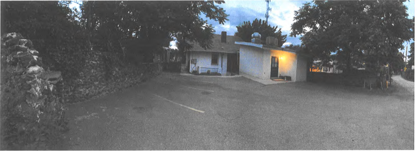
Panorama of North facade viewed from NE corner of property line
