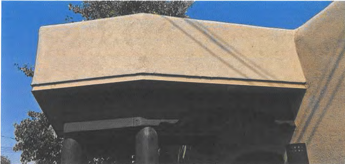
Photo 3: Non-historic portal roof, east side. Camera facing up.
