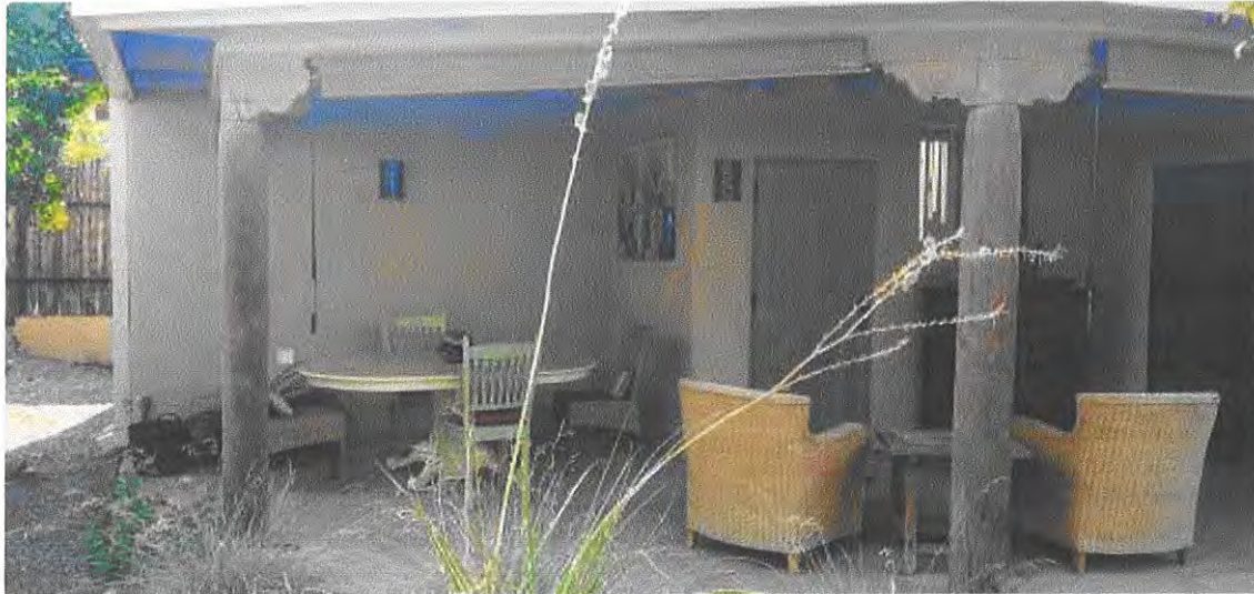
Photo 7: North elevation, non-historic portal. Camera facing south.
