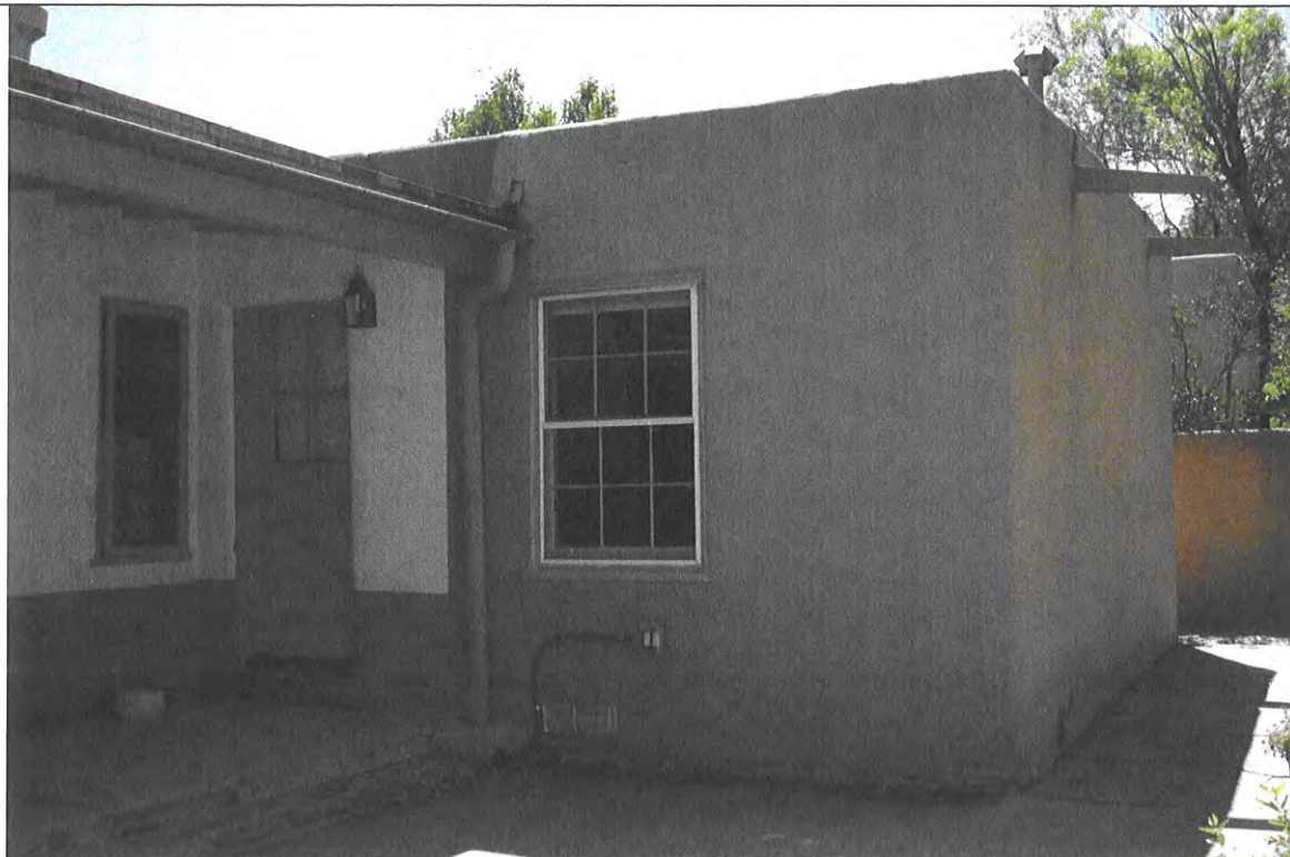
Back Porch facing west. The back massing was added after house was built in 1951. Note steel canals.
