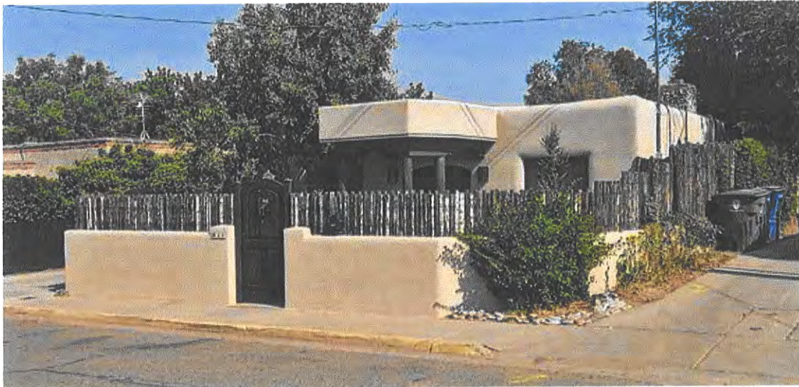
Photo 1: Street view of south, front façade. Camera facing northwest.
