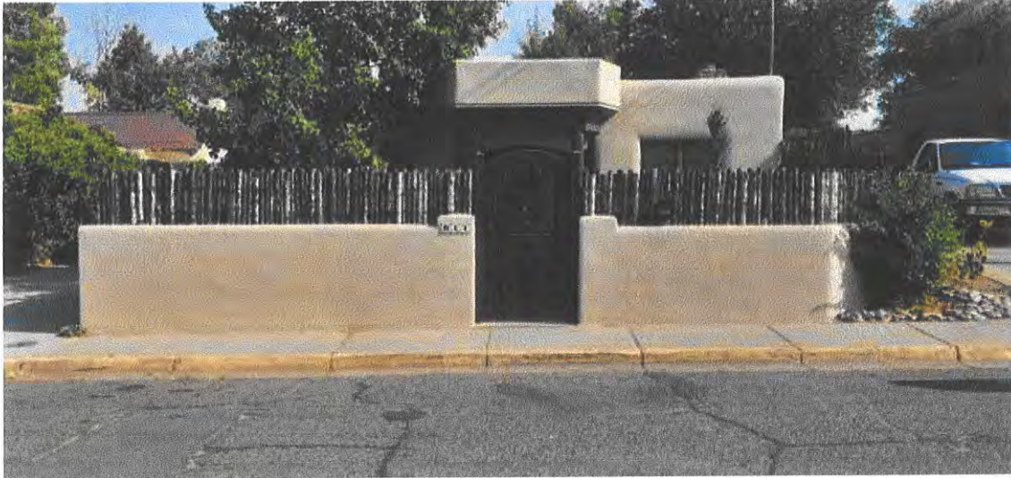
Photo 2: South, front façade. Camera facing north.
