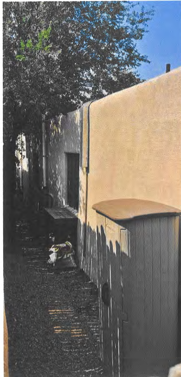
Photo 8: East elevation. Camera facing southwest.
