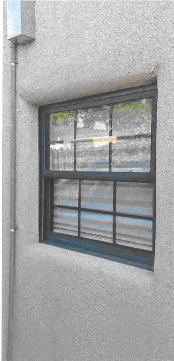
Photo 6: West elevation, typical window. Camera facing northeast.
