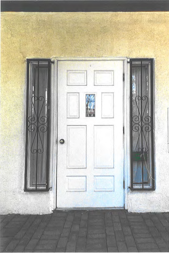
South Façade: West door on front porch, proposed to replace
