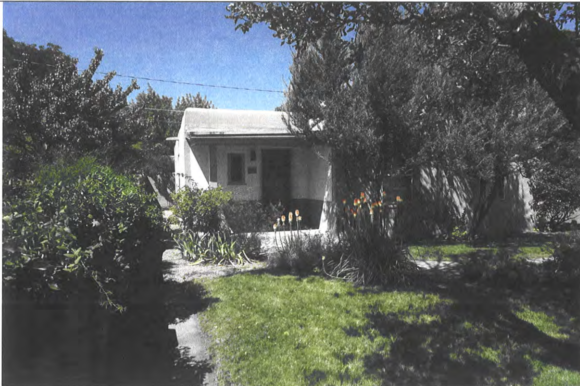
Front Porch facing east and the Street
