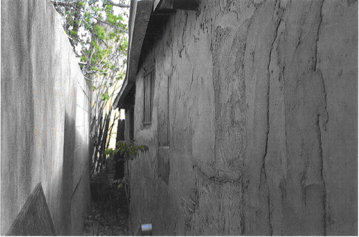
Portion of North Façade
