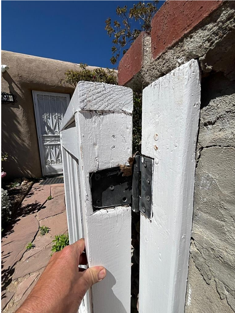
Photo 15: Gate. Detail of construction. Camera facing north.
