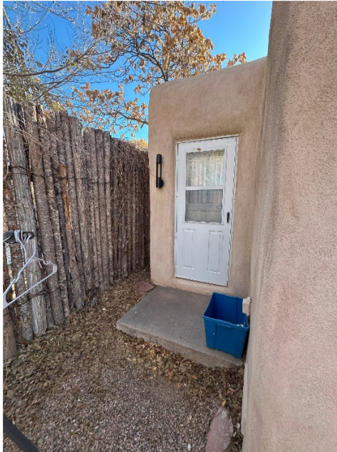
View of REMAINDER NORTH ELEVATION
