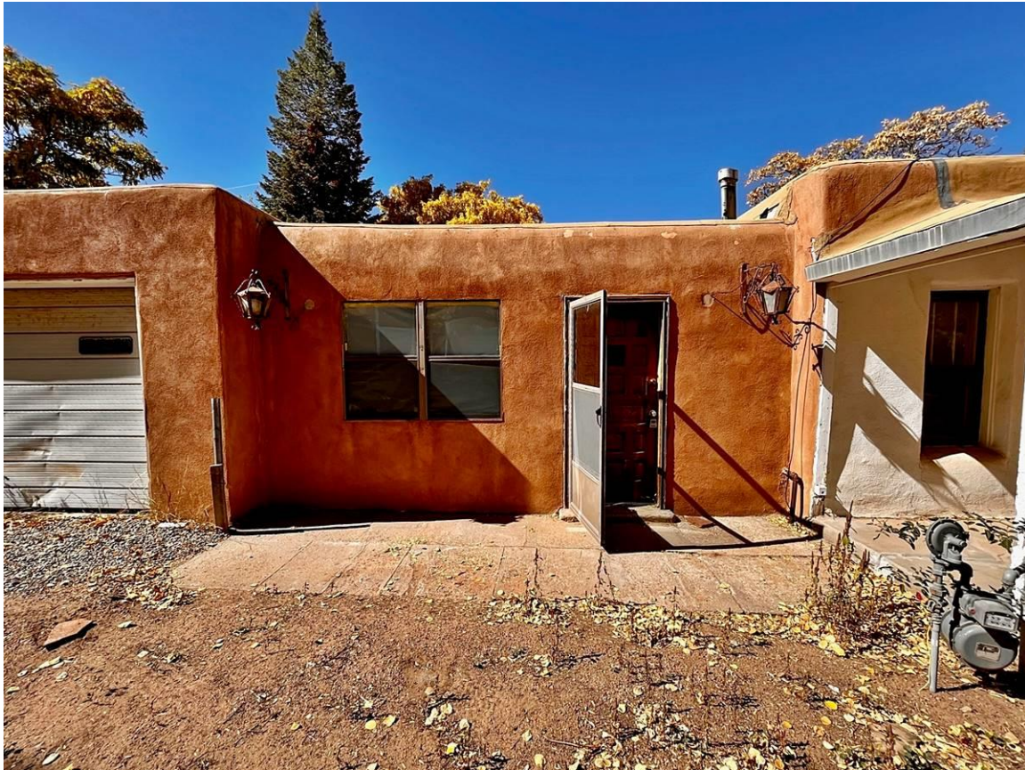
Photo 4: East façade, Family Room (c.1976). Camera facing west.
