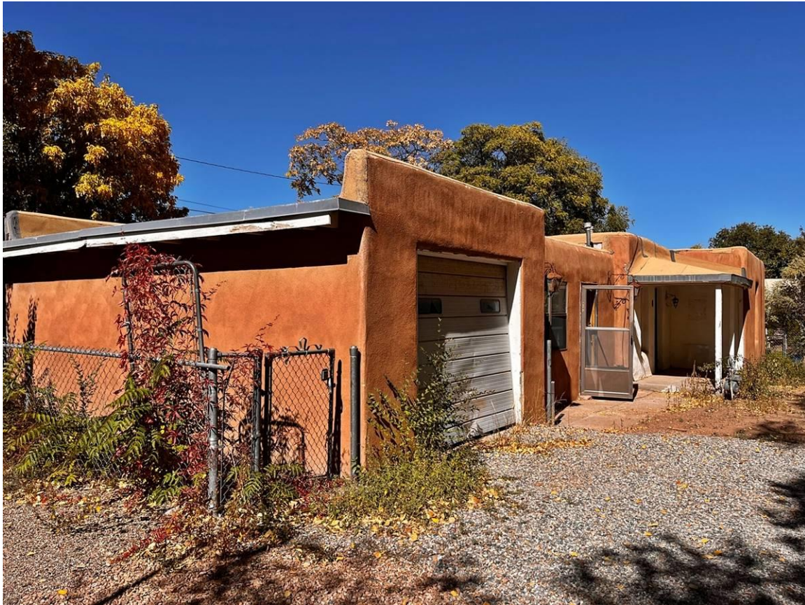
Photo 3: East façade, Garage (c.1966-1973). Camera facing northeast.
