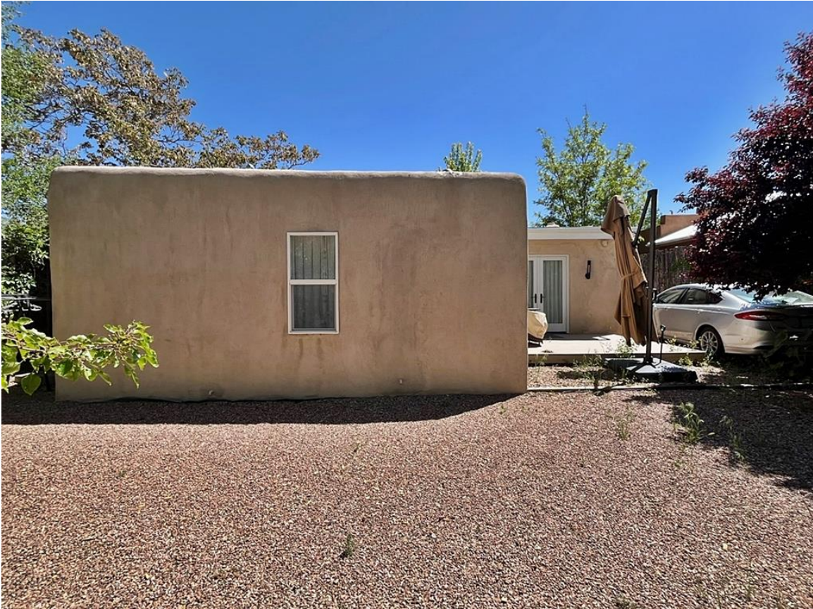
Photo 9: North elevation. Camera facing south.
