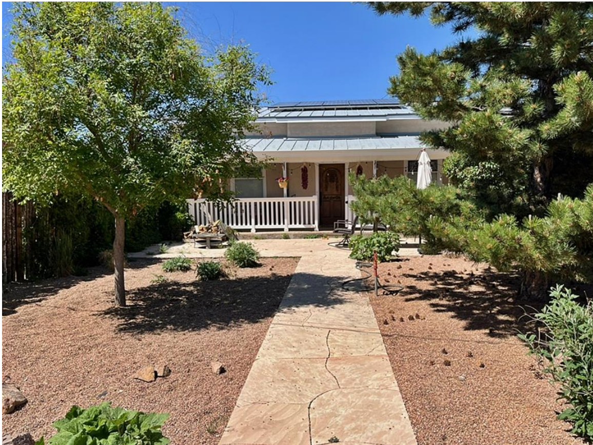
Photo 3: Hilario Ortiz House. Camera facing north.
