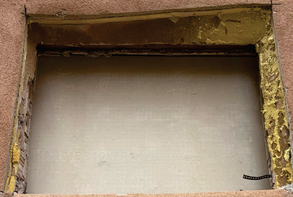
South Elevation Window #3
