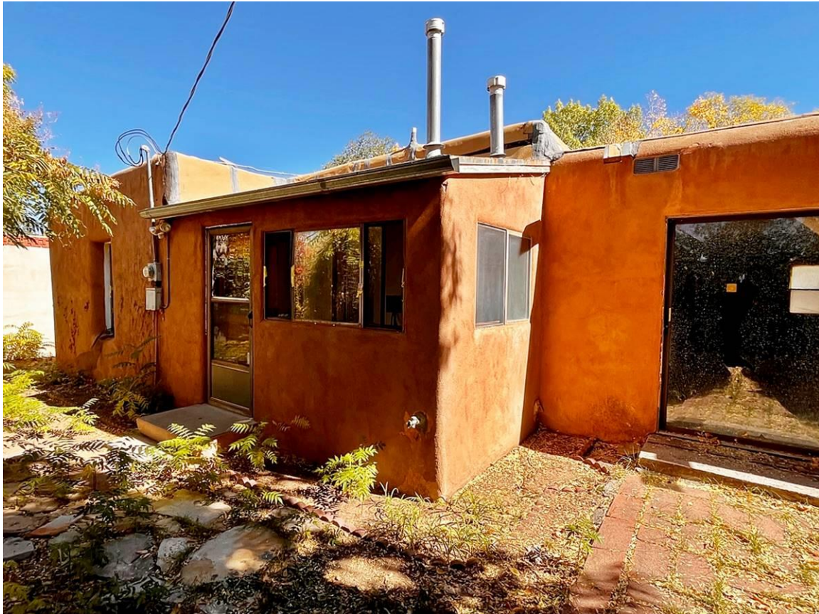
Photo 17: West elevation, Laundry Room (c.1958-1966) at center. Camera facing northeast.
