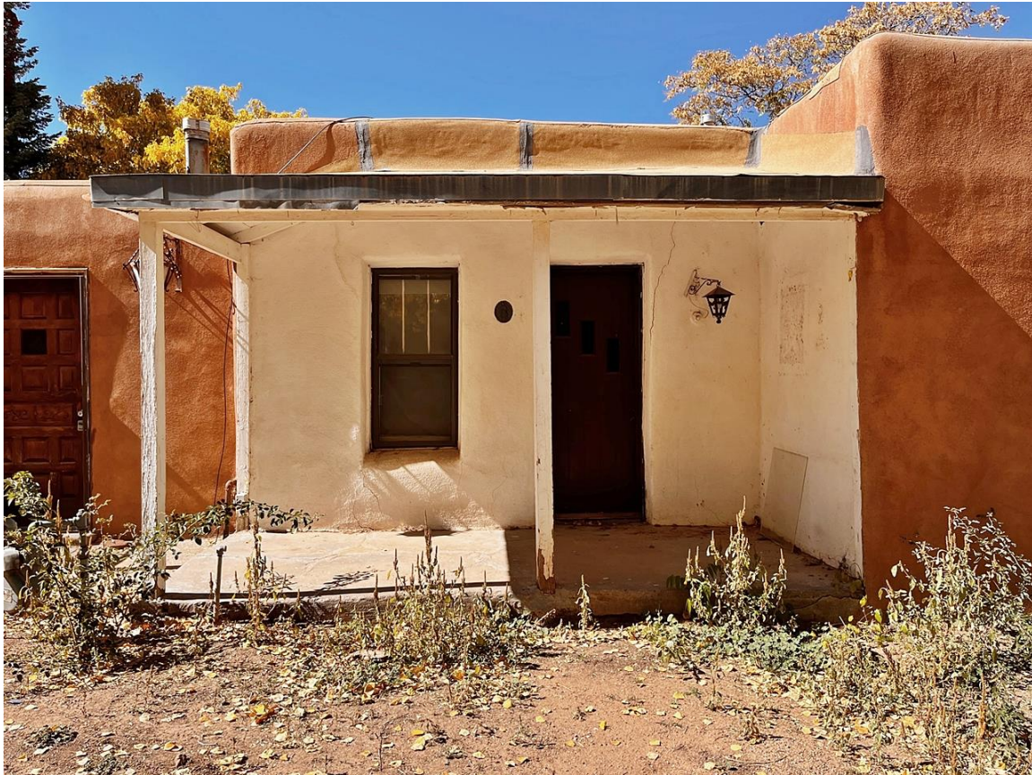
Photo 6: East façade, Porch (c.1966-1973). Camera facing west.
