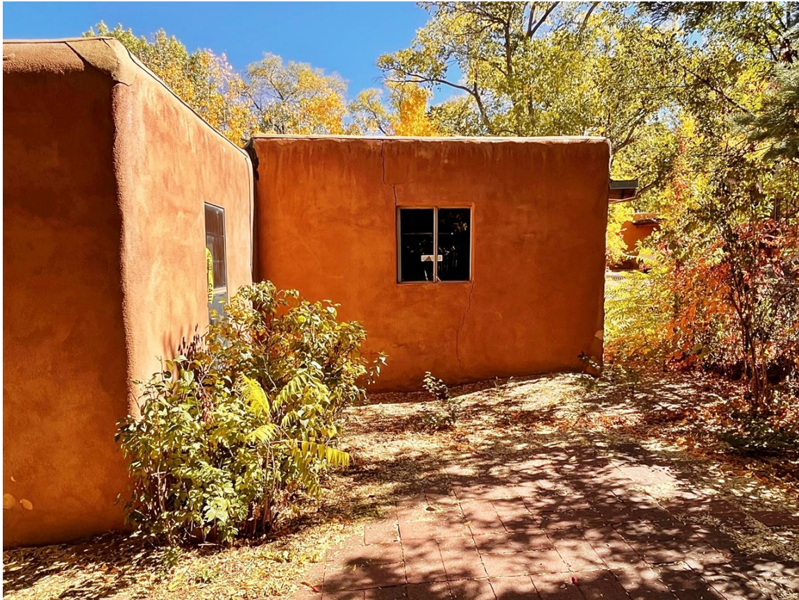
Photo 20: West elevation, Garage (c.1966-1973). Camera facing east.
