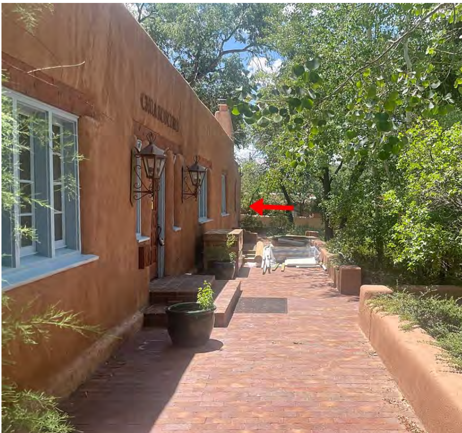
Figure 23: Comparison. North elevation, 1925 and 2025. Arrow indicates addition.
