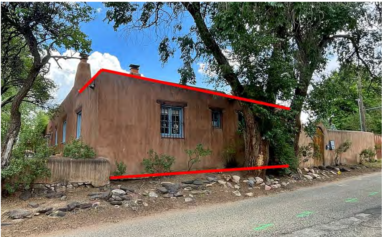
Figure 19: West elevation. Red indicates post-Austin/Meem additions.
