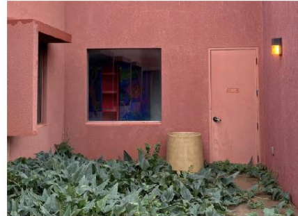
Typical openings. Fixed window(s) left, hollow metal door (right).
