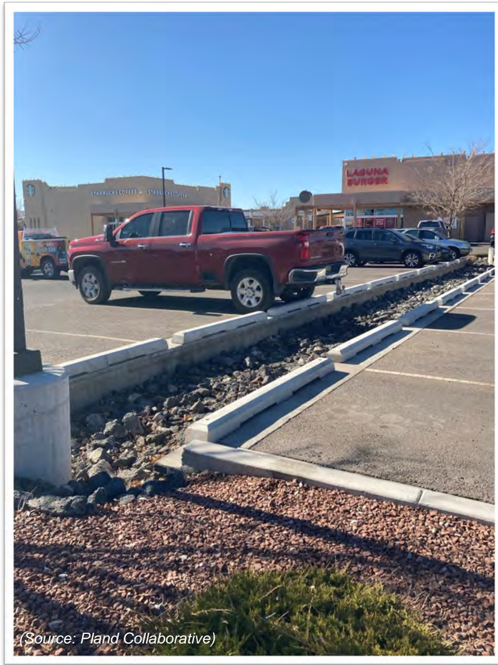
Figure 70: Infiltration trench in a commercial parking lot in Albuquerque, NM. This method can also be used along streets.
