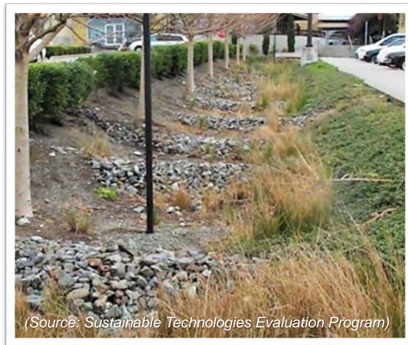
Figure 72: Check Dams Made with Rock
