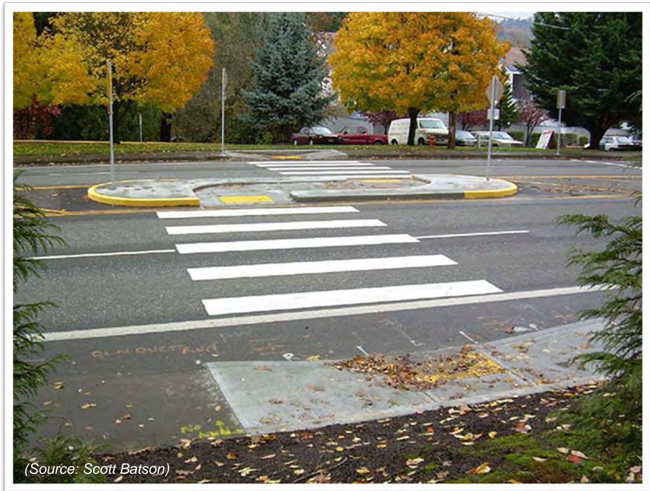
Figure 40: Median Island with Pedestrian Refuge and Offset Crosswalk
