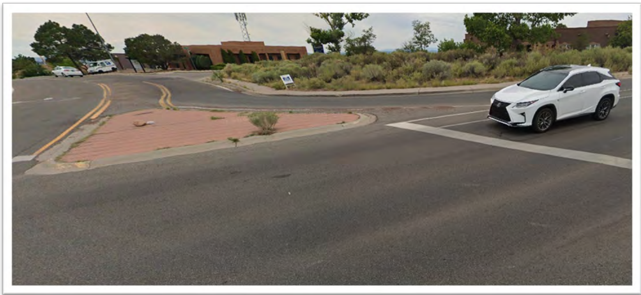
Figure 48: Mountable Curb Median Example
