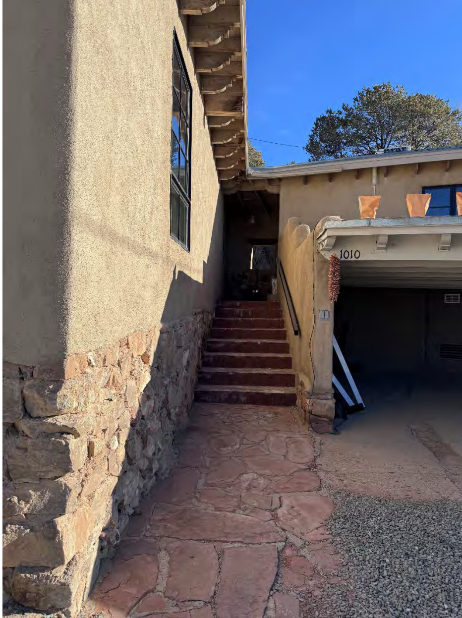
Detail of entry stairs, north and west elevations.
