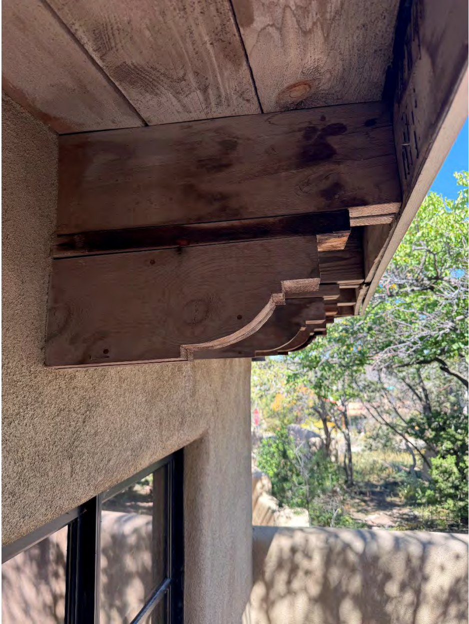
Detail of decorative corbelled brackets.
