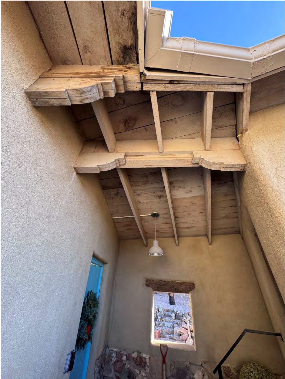
Detail of entryway between house (left) and carport (right).
