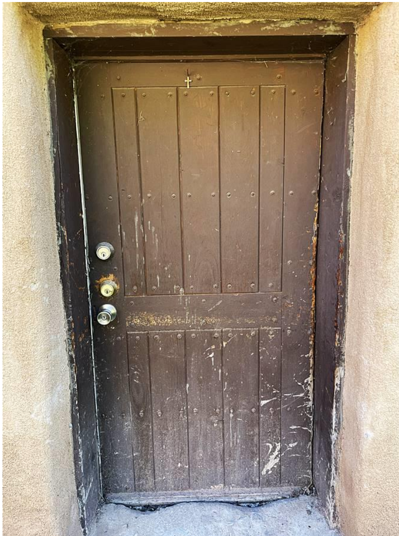
Photo 11: North elevation. Entry door at ground level. Camera facing south.
