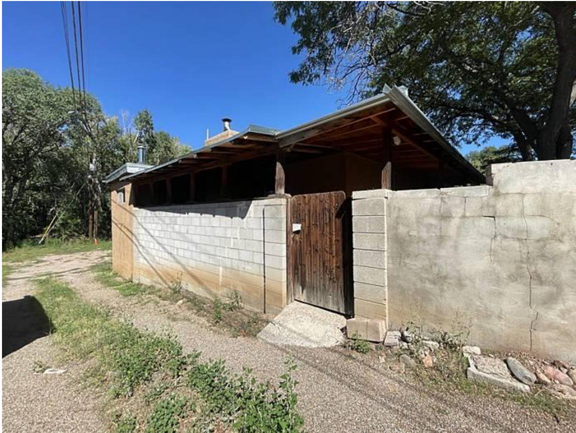
Photo 6: West elevation. Camera facing northeast.
