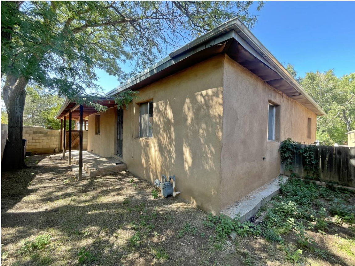
Photo 3: South(front) and east elevations. Camera facing northwest.
