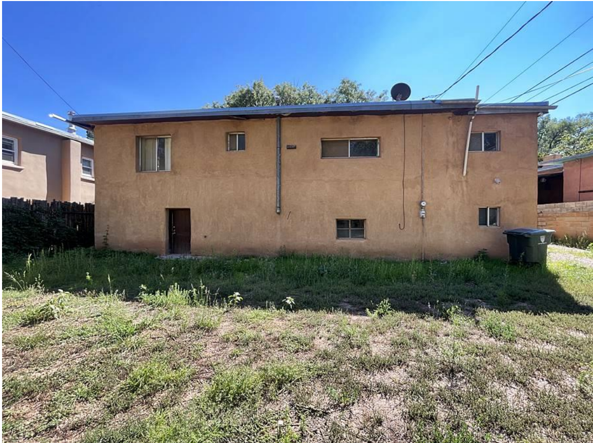
Photo 10: North elevation. Camera facing south.
