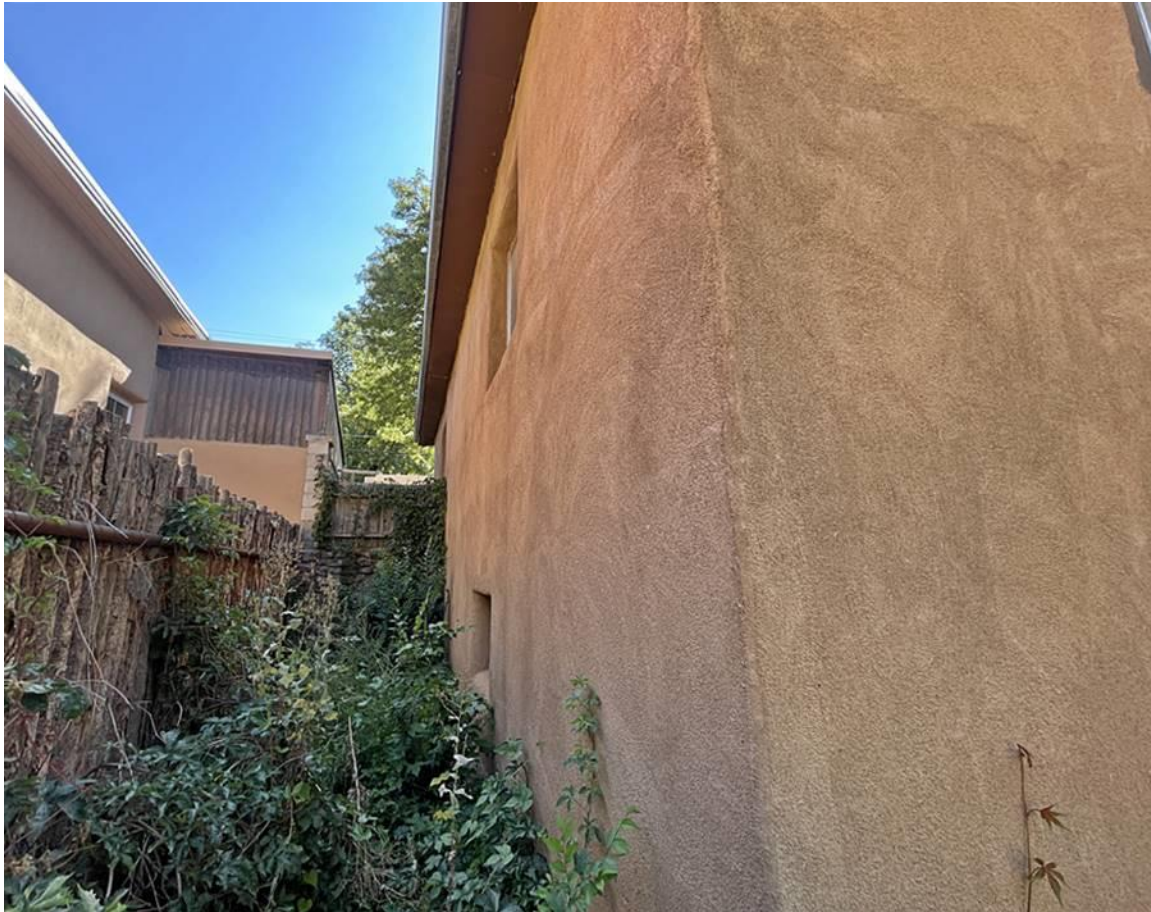
Photo 13: East elevation. Camera facing south.
