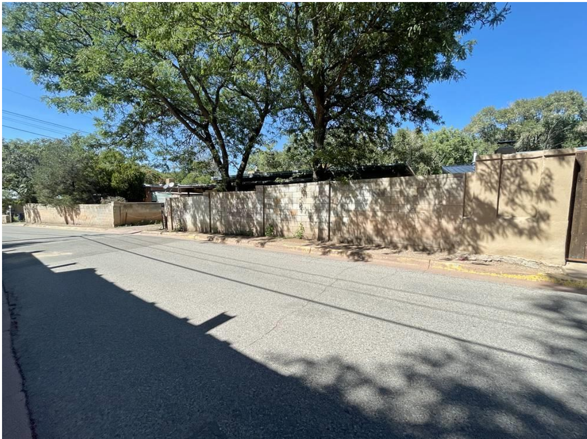
Photo 2: Canyon Road and street walls. Camera facing northwest.
