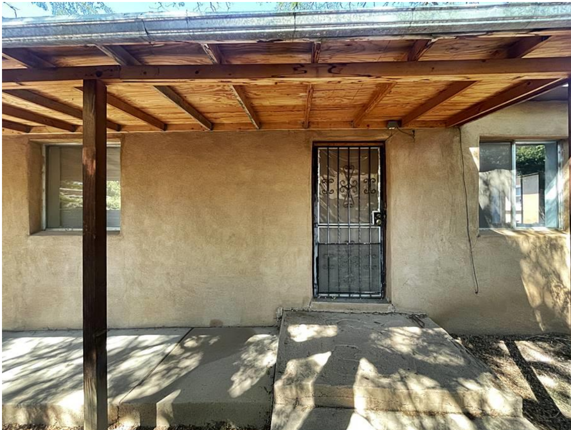
Photo 4: South (front) elevation and porch. Camera facing north.
