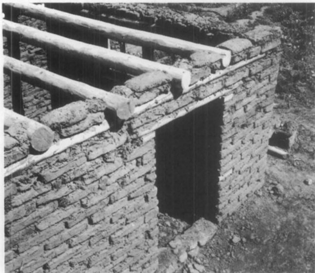
Roof Bearing. A roof bearing timber placed within the adobe walls provides even support for the weight of the roof. (Farm Security Administration Collection, Library of Congress)
