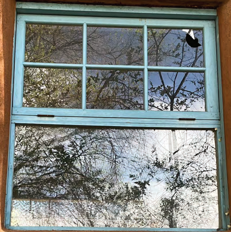
North Elevation 1st Floor Window S
