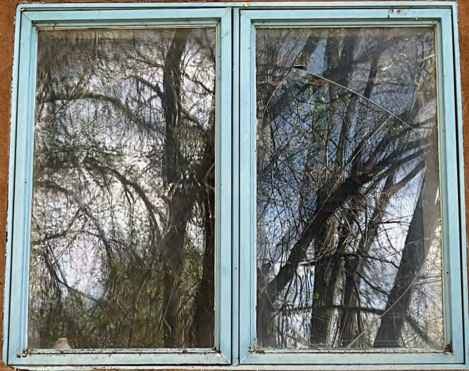
North Elevation 1st Floor Window Q
