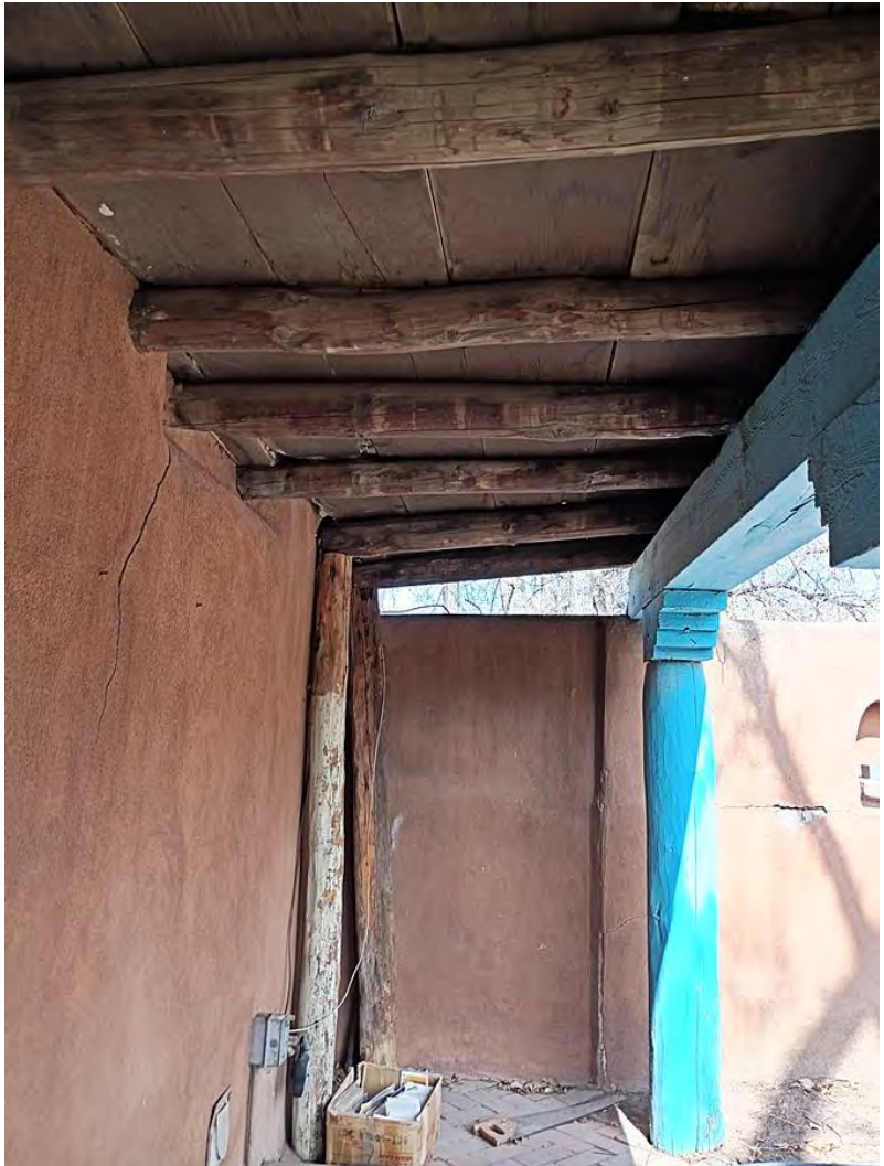
Photo 13: East elevation, portal. Camera facing north.
