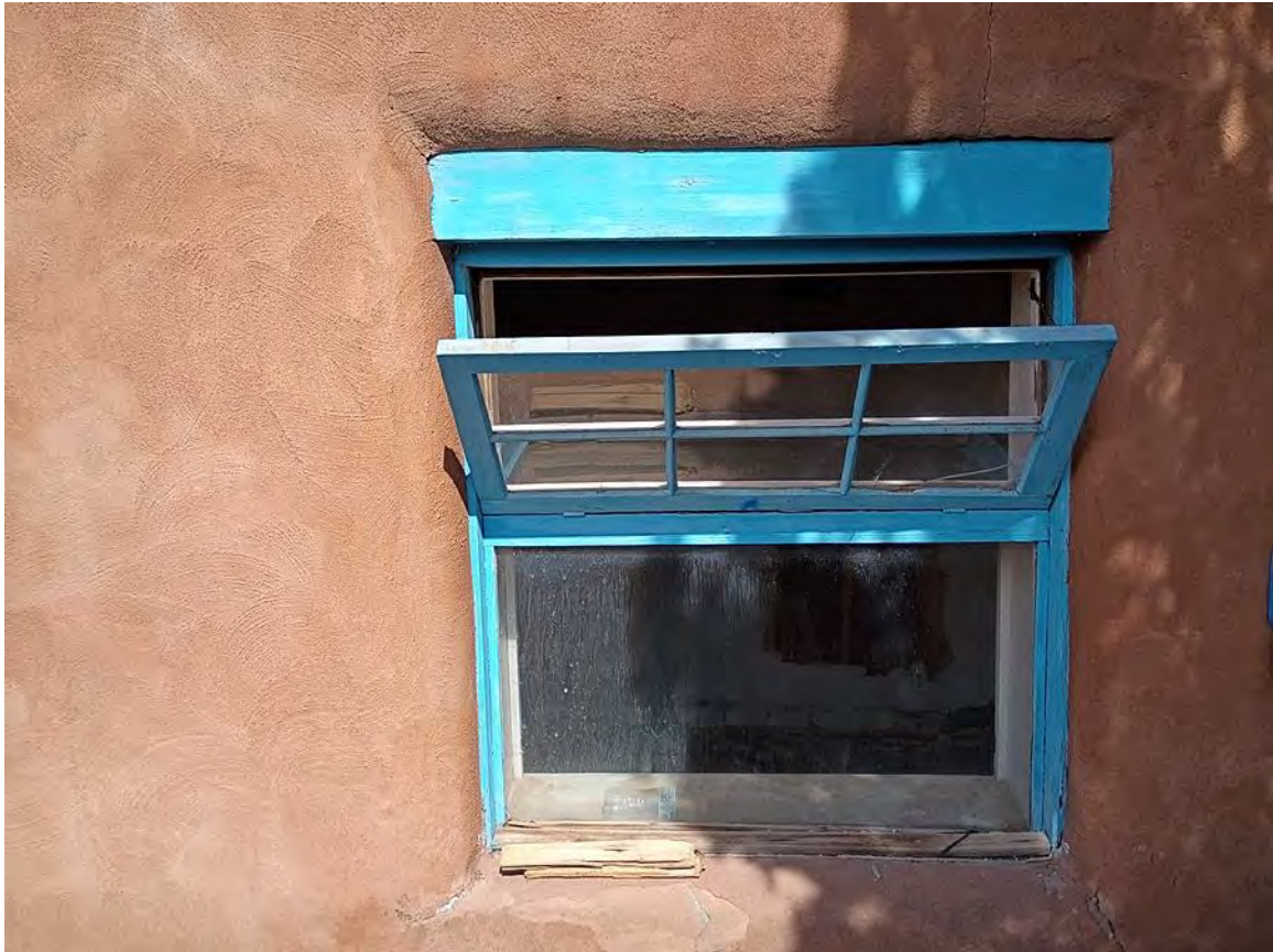
Photo 9: South elevation, ground floor window. Camera facing north.
