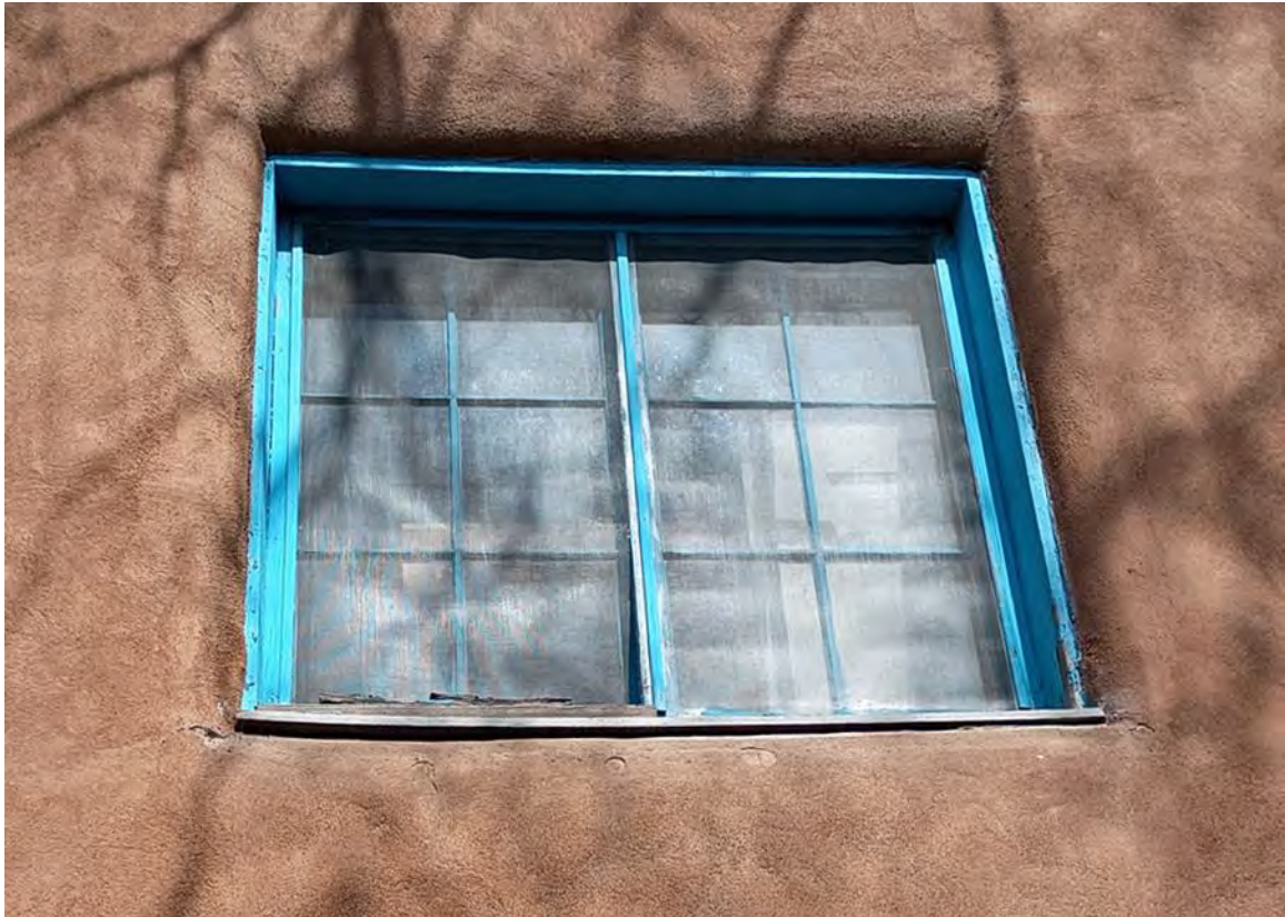
Photo 6: South elevation, second-story window. Camera facing up.
