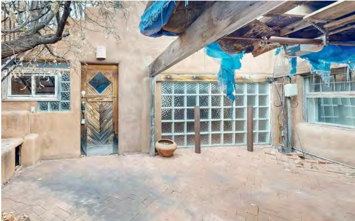
Photo 10: South elevation, original building and addition. Real estate photo.
