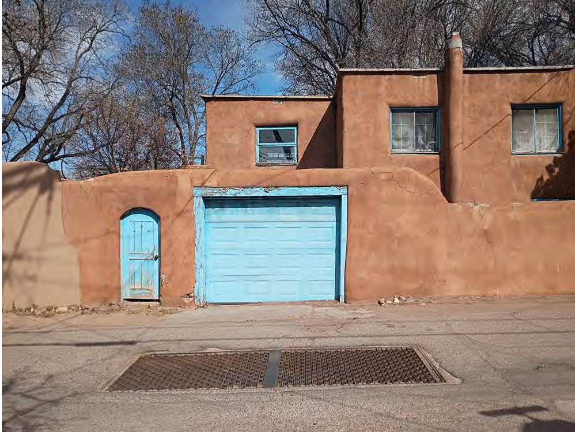
Photo 3: South elevation, west side. Camera facing north.
