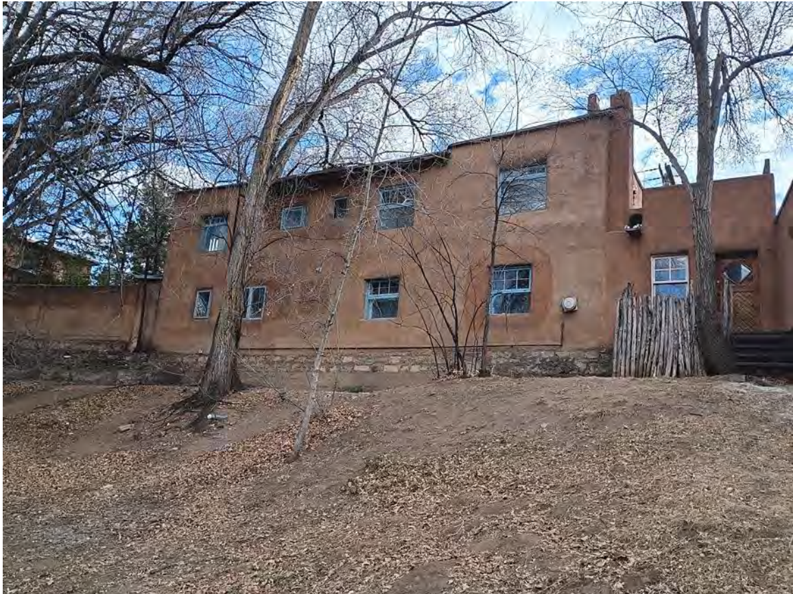
Photo 15: North elevation. Camera facing southeast.
