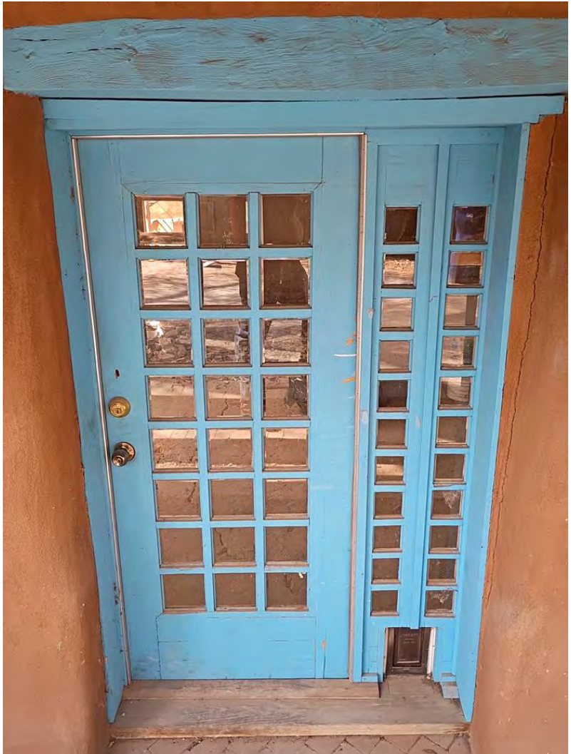
Photo 14: East elevation, ground floor entry. Camera facing down.
