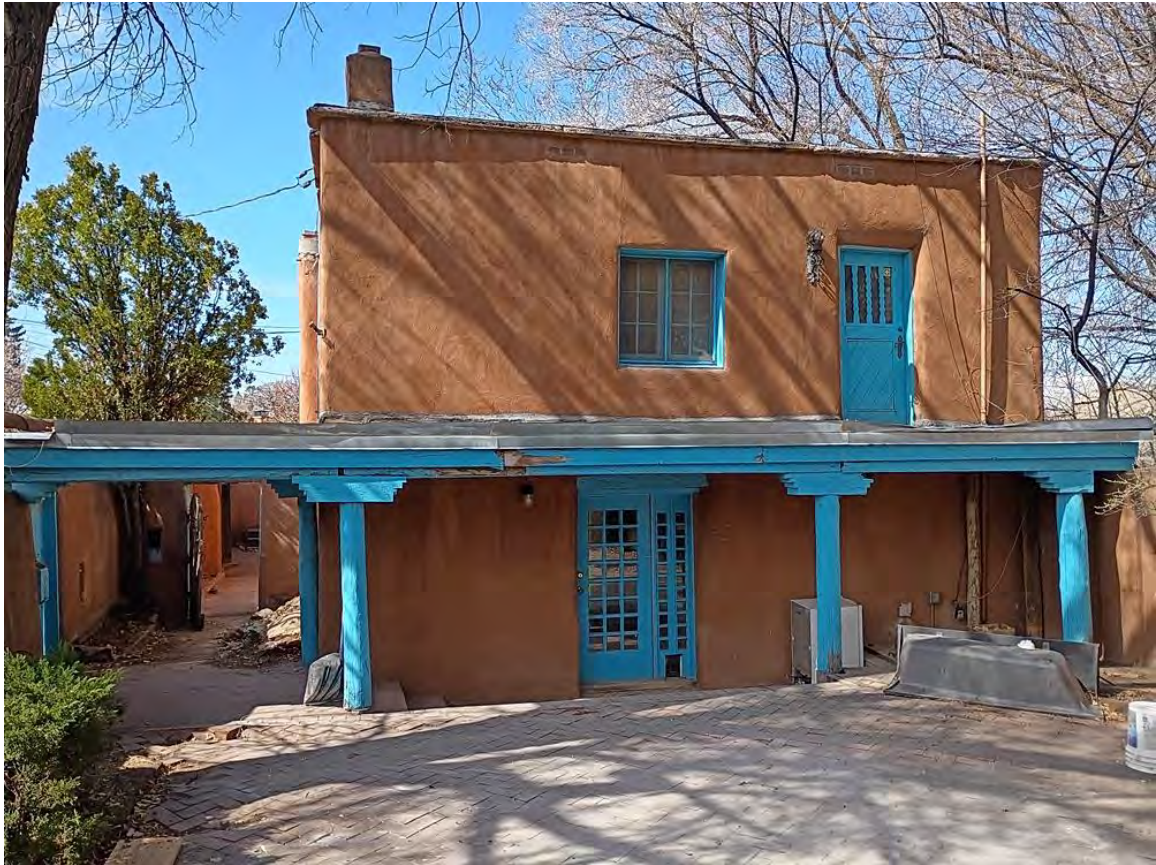
Photo 12: East elevation. Camera facing northwest.
