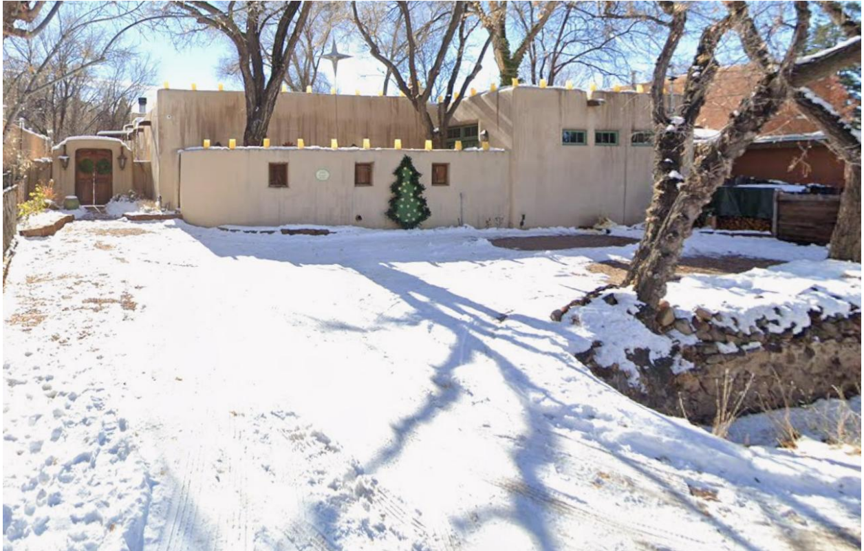
Figure 2: Streetview of Property
