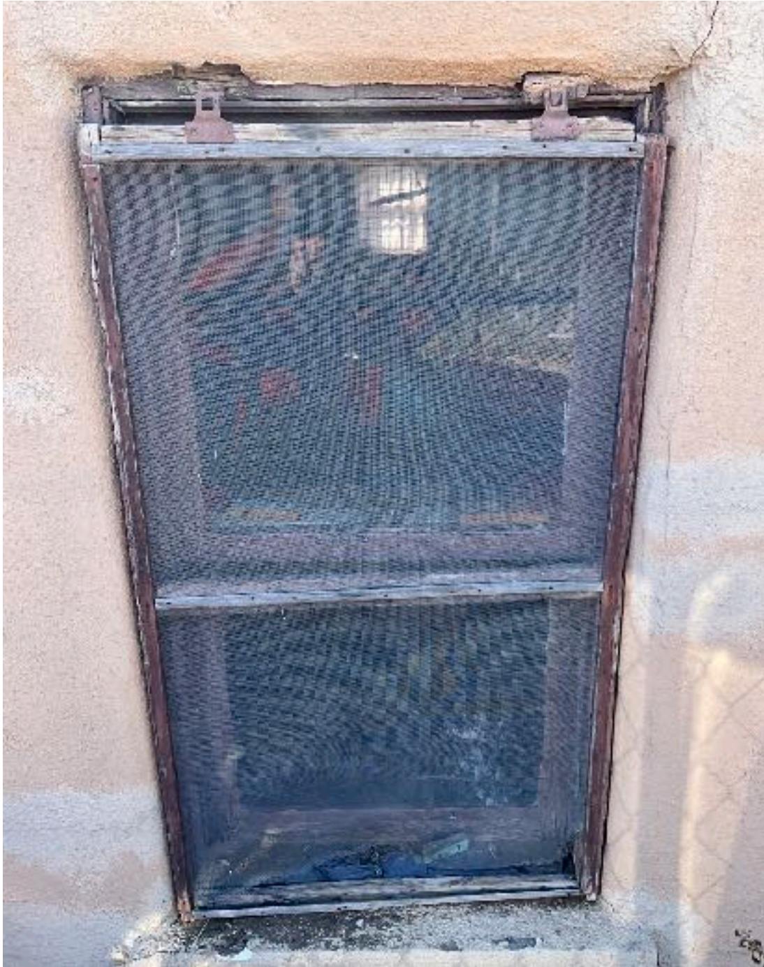
East Window #1 Double Hung Window 24 x 46
