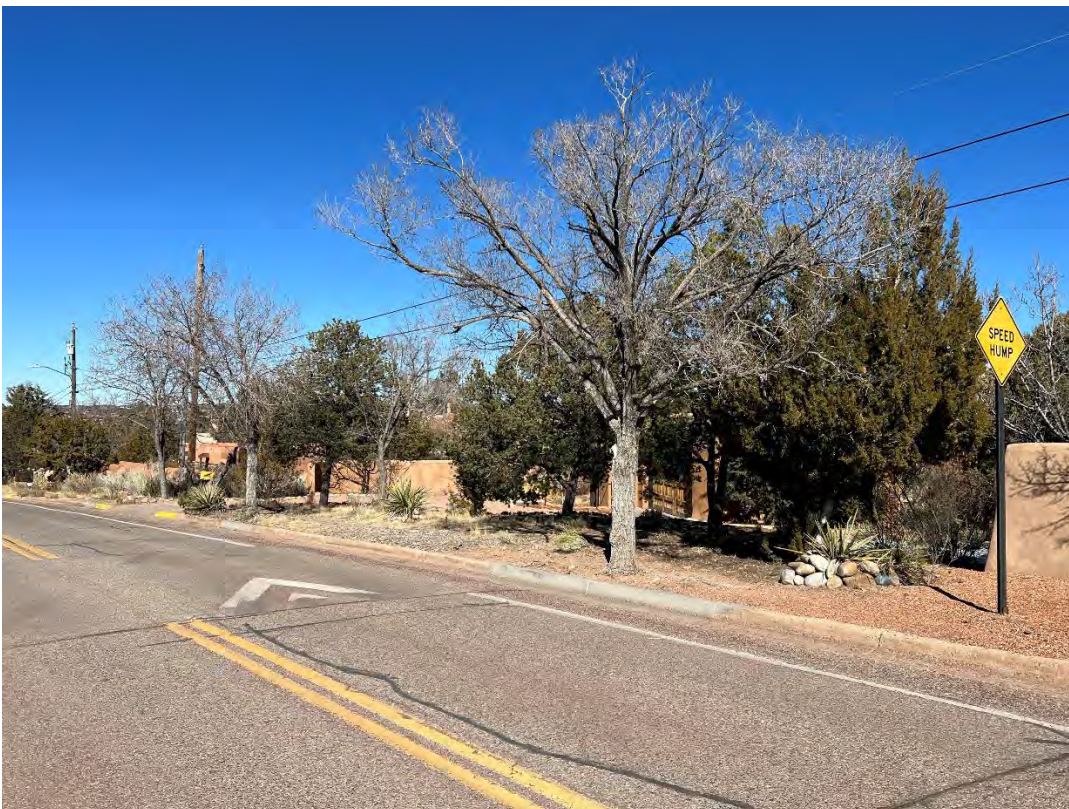
Garcia St. View – Looking North
