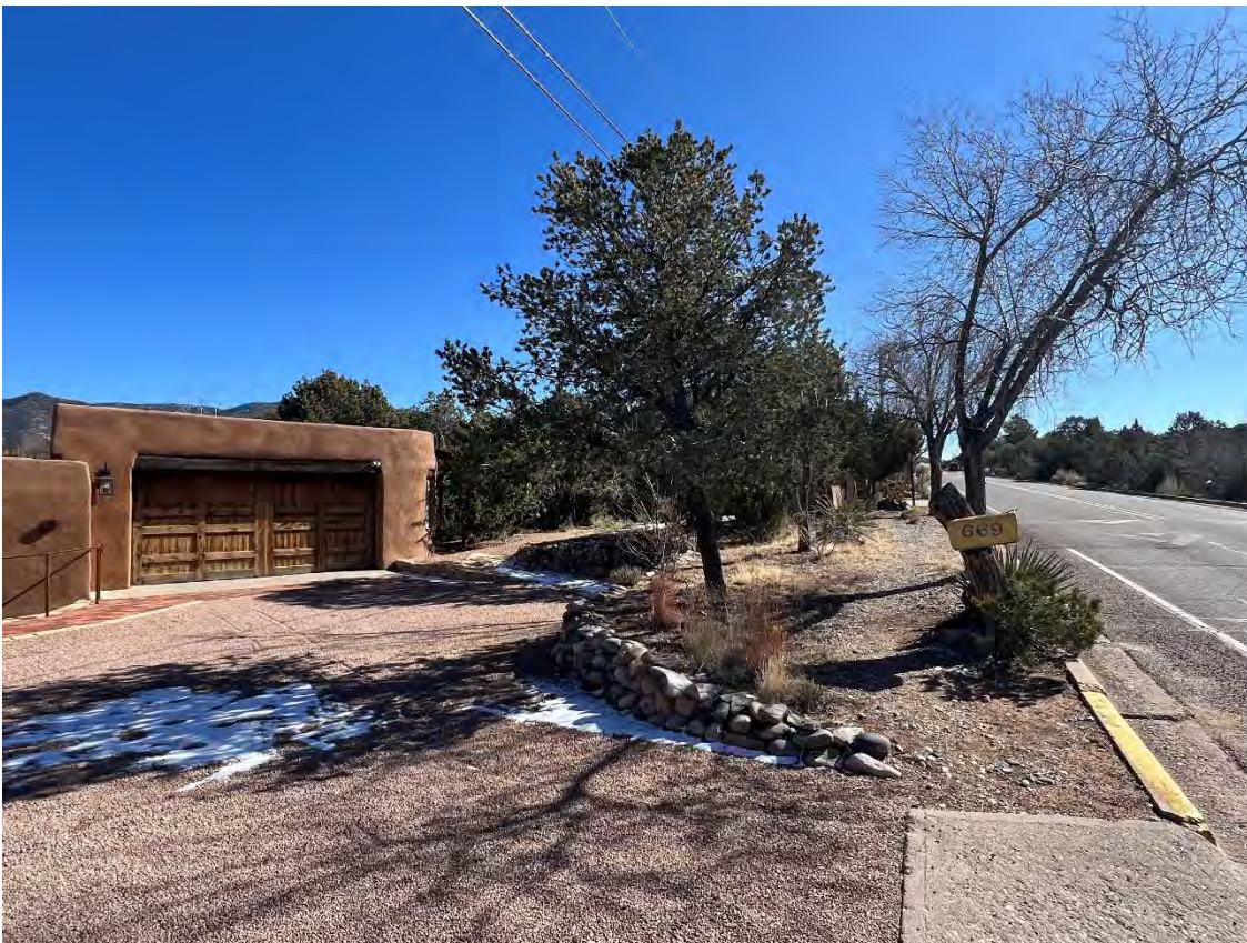
West Side – Drive Court Looking South – Proposed Vehicle Gate Location
