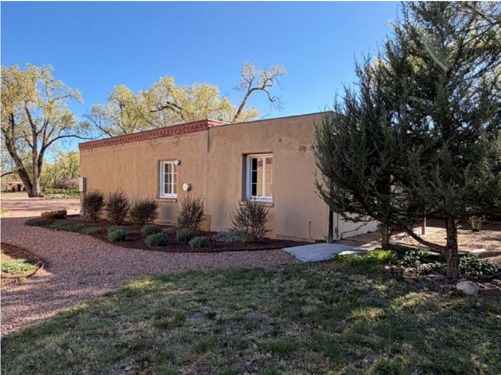
West Elevation Looking North
