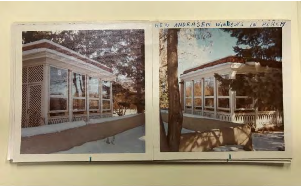
1974 Enclosure of Sleeping Porch
