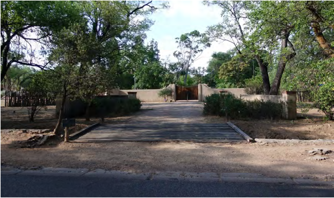
Estate Entry on Acequia Madre, indicating acequia bridge and view from public way
