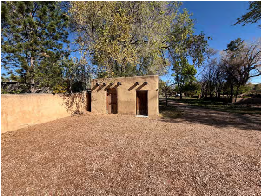
Former horse barn at west, south elevation
