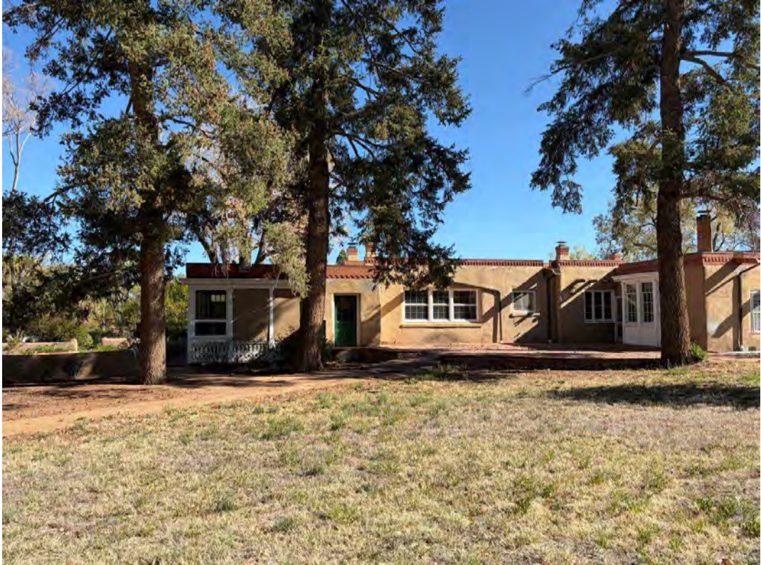
South Façade, West Side
