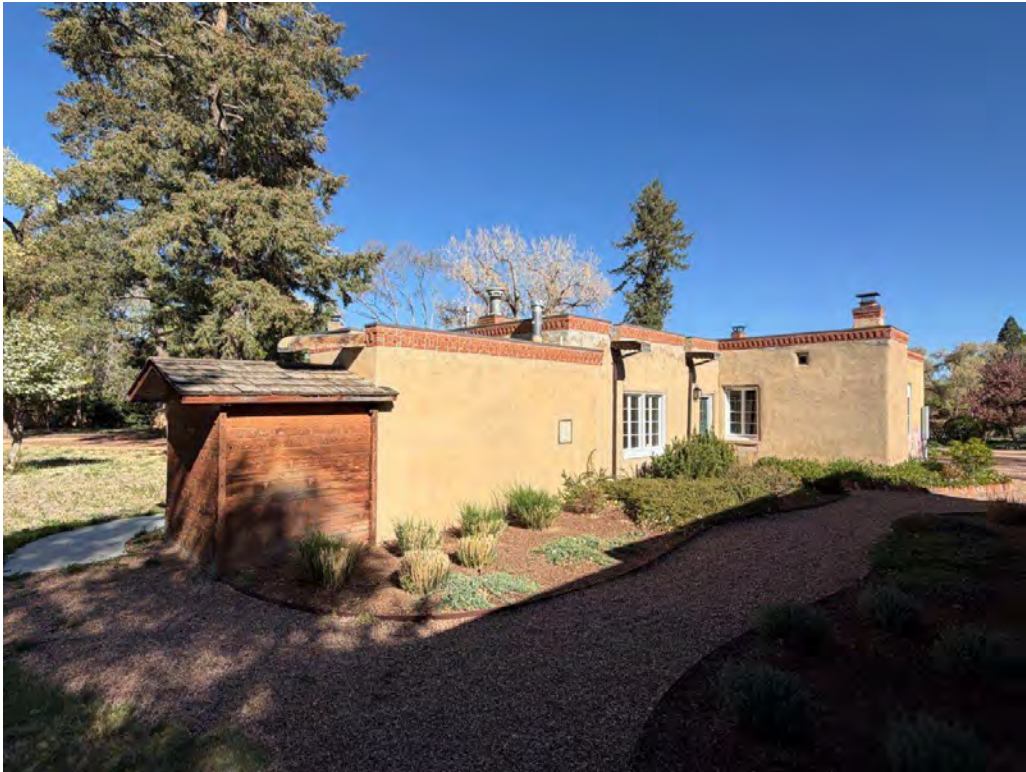
East Elevation, South Aspect (Sauna and Pool Changing Rooms are at left)
