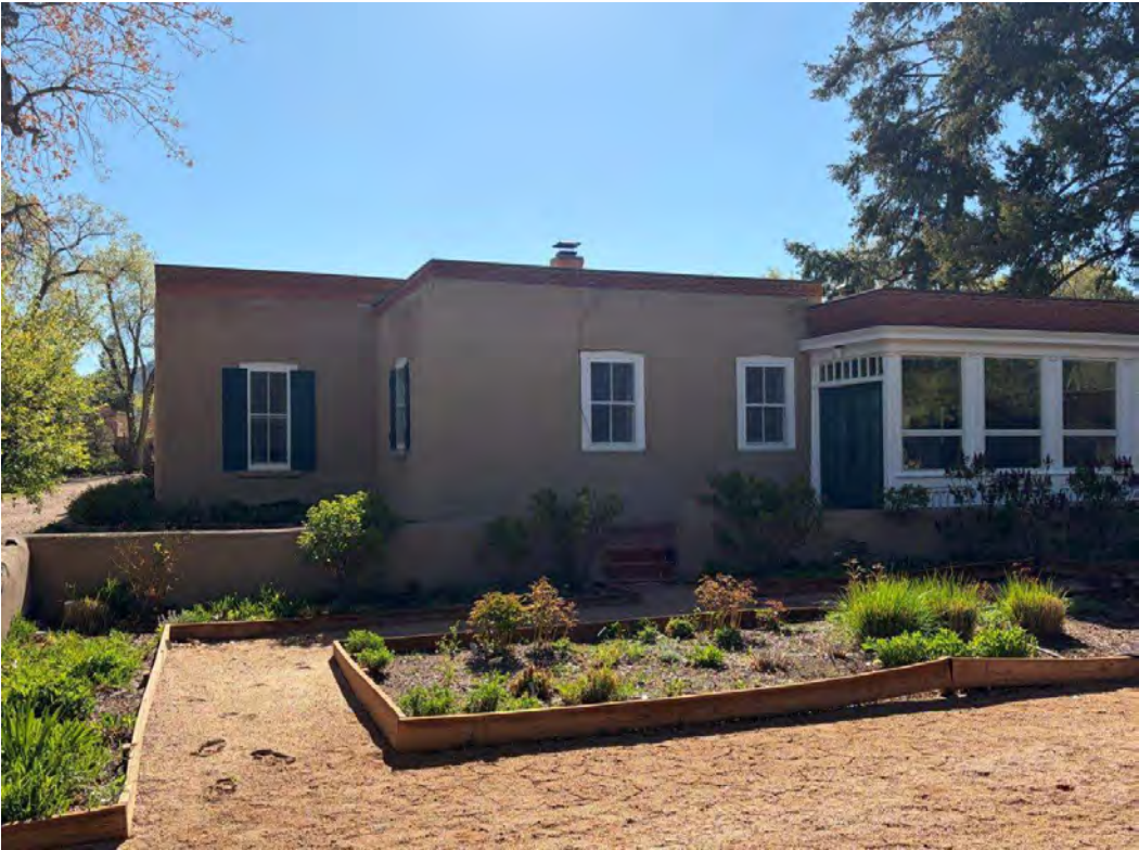
West Façade – at Northwest Corner (Green Door from 1974 Infill)
