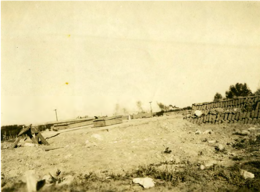
1925 view of adobe making operation, from Acequia Madre House Archives
