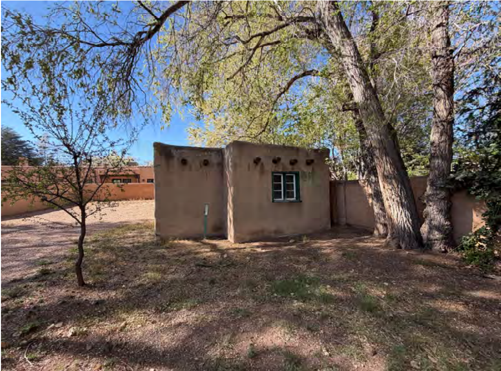
Former horse barn at west, north elevation
