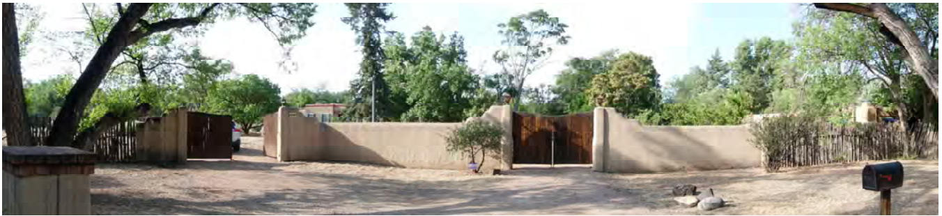
North (front) Landscape Wall and Entry Gates – Viewed from the Road
