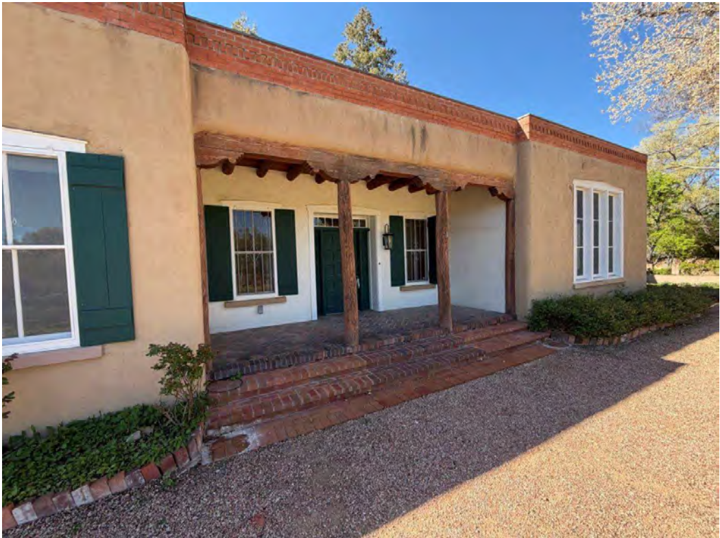
North Façade – Main Entry Portal with Shutters
