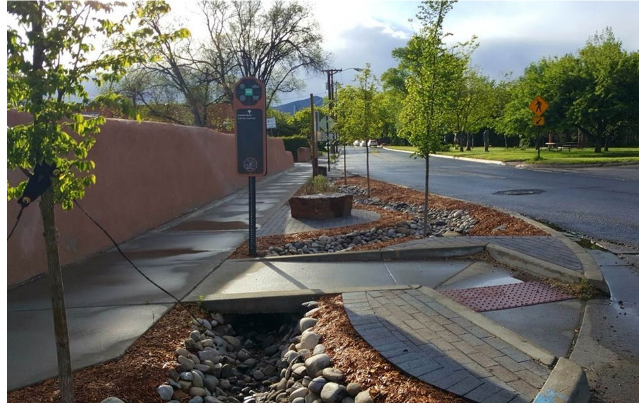
Rain Garden at Cathedral Pl and E Alameda (designed and constructed by Seeds of Wisdom)
