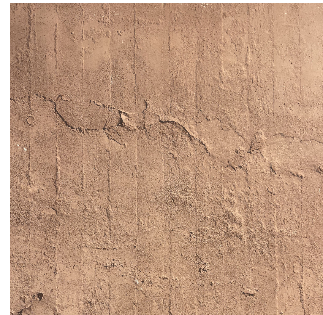
Existing Cast Concrete Retaining Wall
