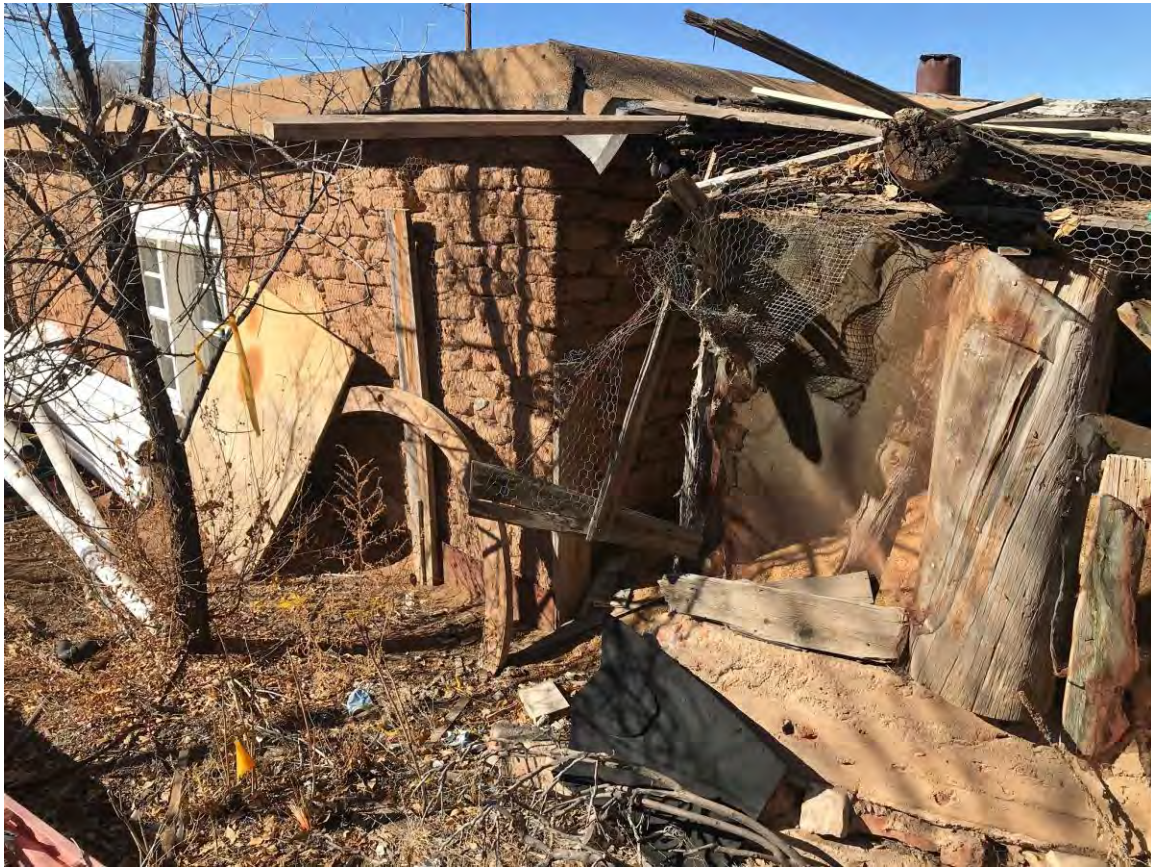
Photo 13: Shed, south portion at right. Camera facing northwest.
