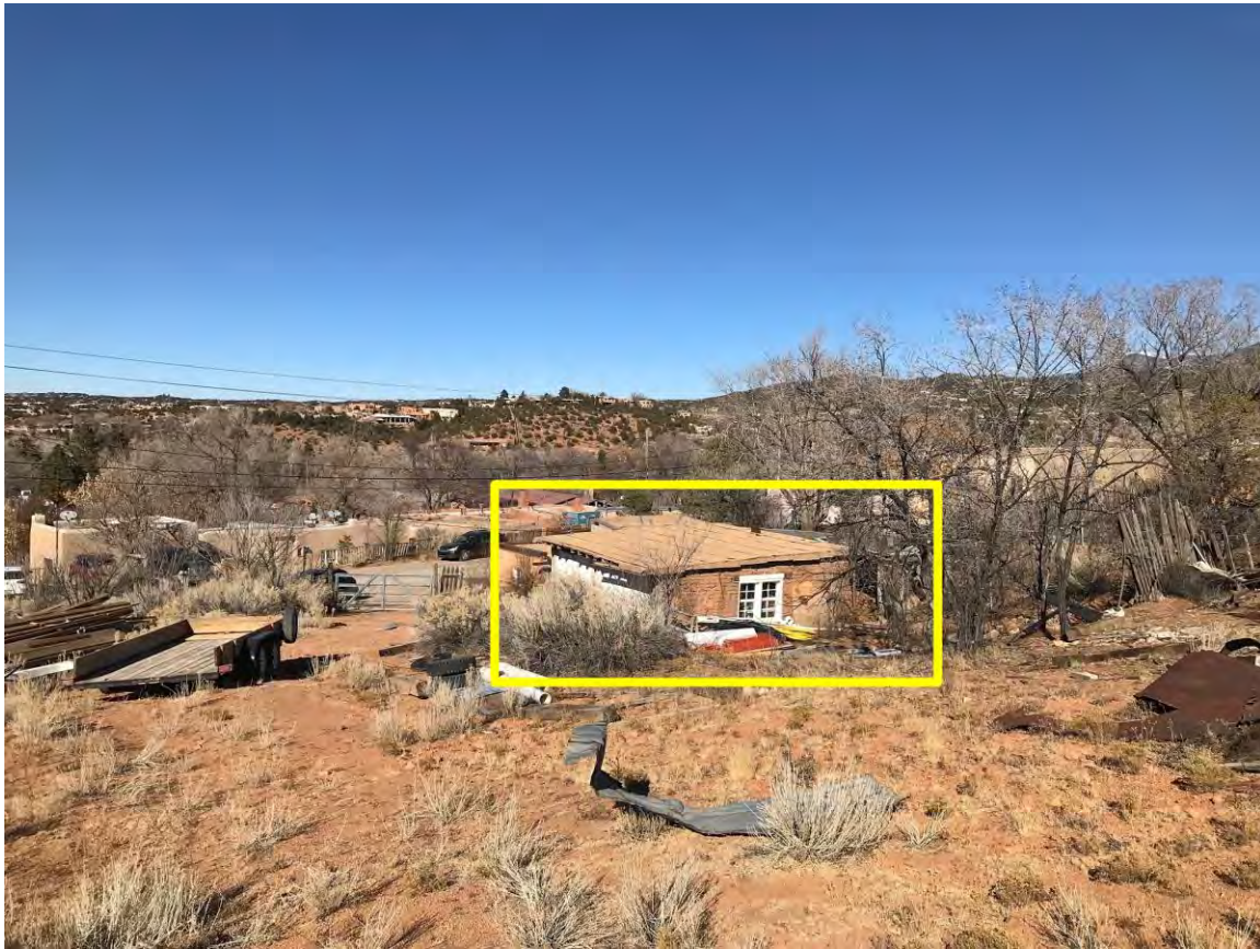
Photo 3: View of Upper Building from south edge of property. Camera facing northeast.
