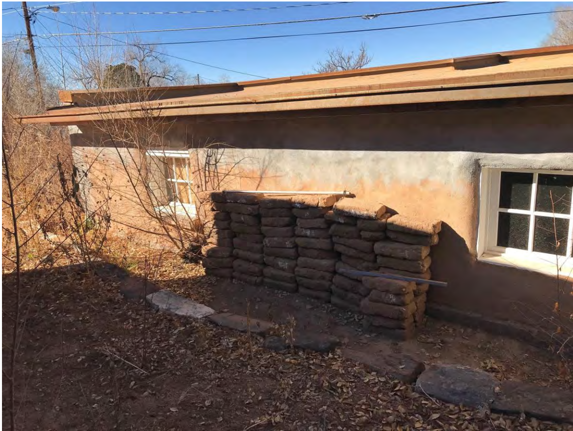
Photo 6: Lower Building, south elevation. Camera facing northwest.
