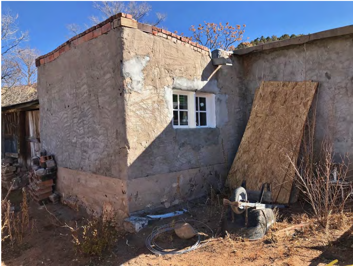
Photo 8: Upper Building, partial north elevation. Camera facing southeast.
