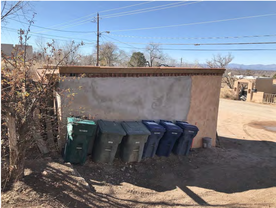
Photo 7: Lower Building, north elevation. Camera facing northwest.
