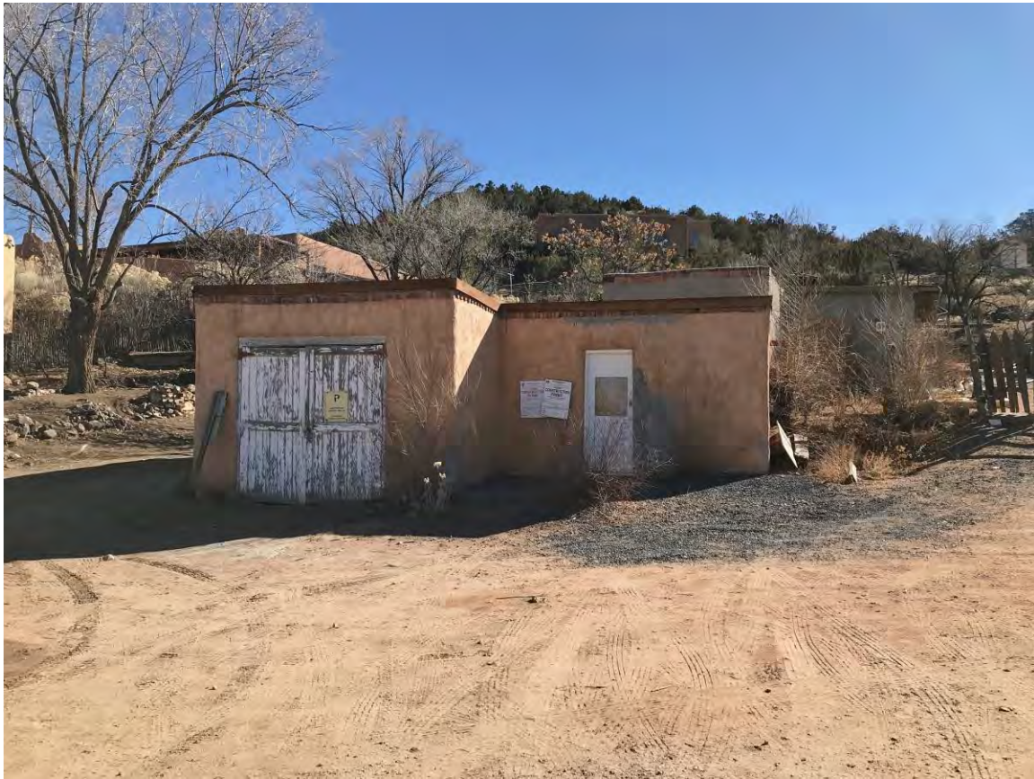
Photo 4: Lower Building, north elevation. Camera facing south.
