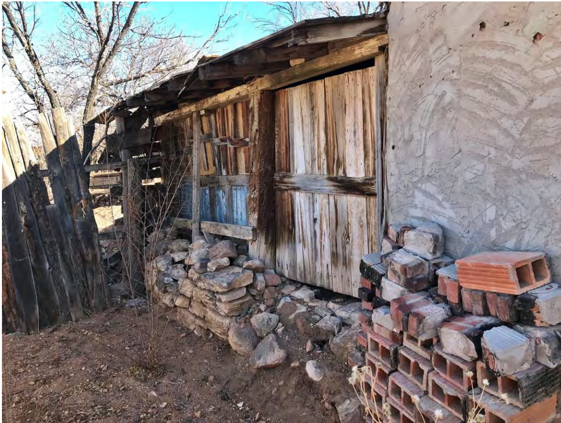
Photo 9: Upper Building, north elevation, shed portion. Camera facing southeast.
