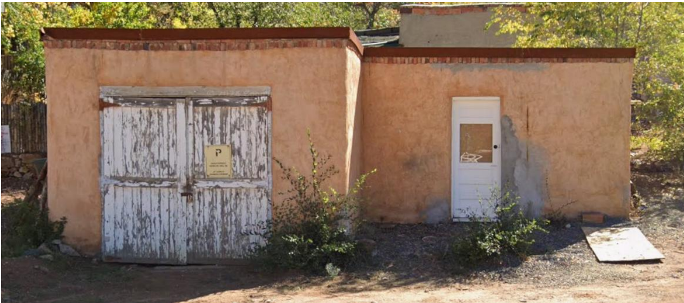
Figure 2: Existing Northern Contributing Garage Structure Historic Districts Review Board, Case #2026-012284-HDRB
