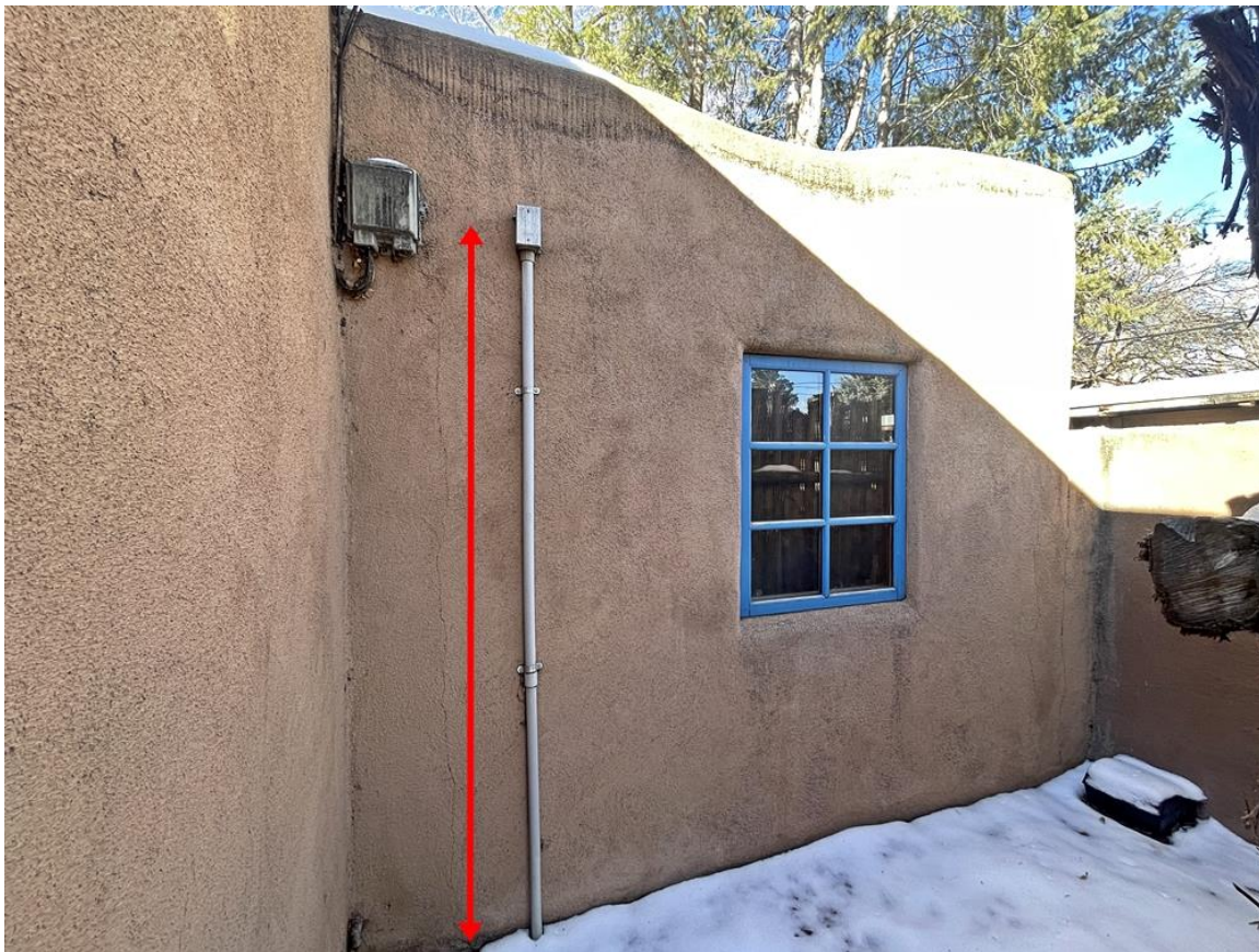
Photo 16: East elevation. 1936 replacement garage with door opening infilled after 1992. Camera facing northeast.
