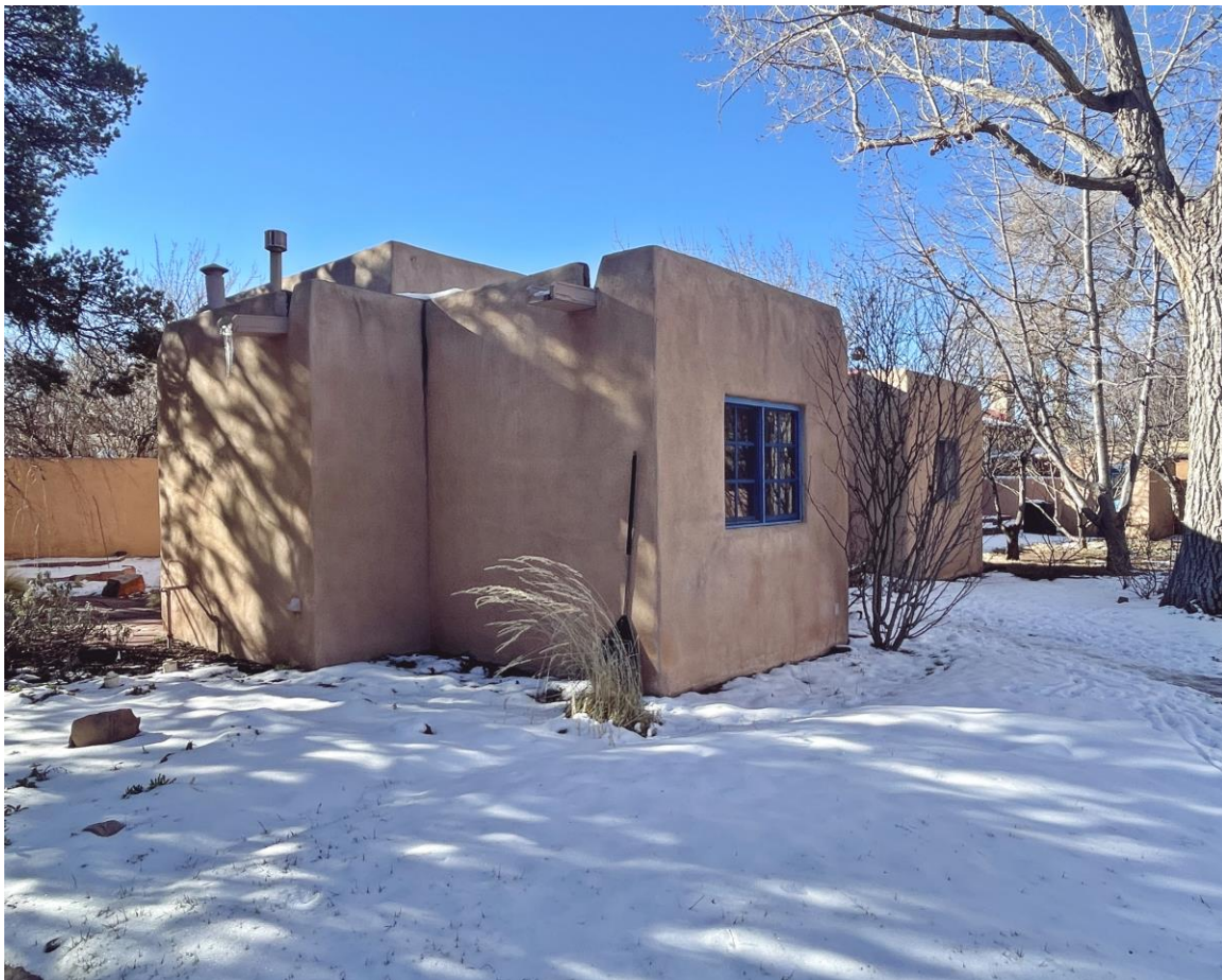
Photo 17: 1992-93 Guesthouse. North elevation. Camera facing southwest.
