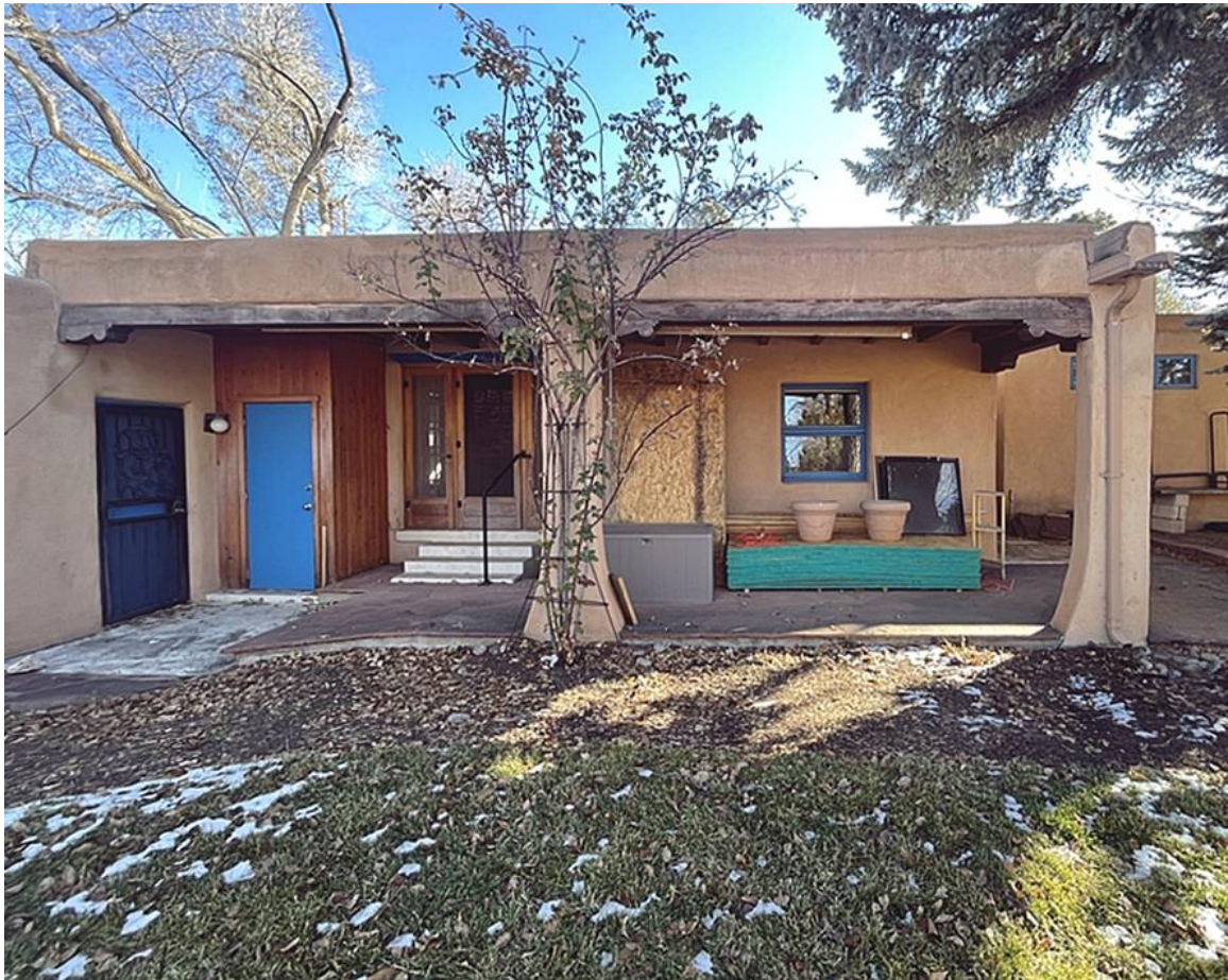
Photo 11: West elevation. Portal erected in 1958. Camera facing east.
