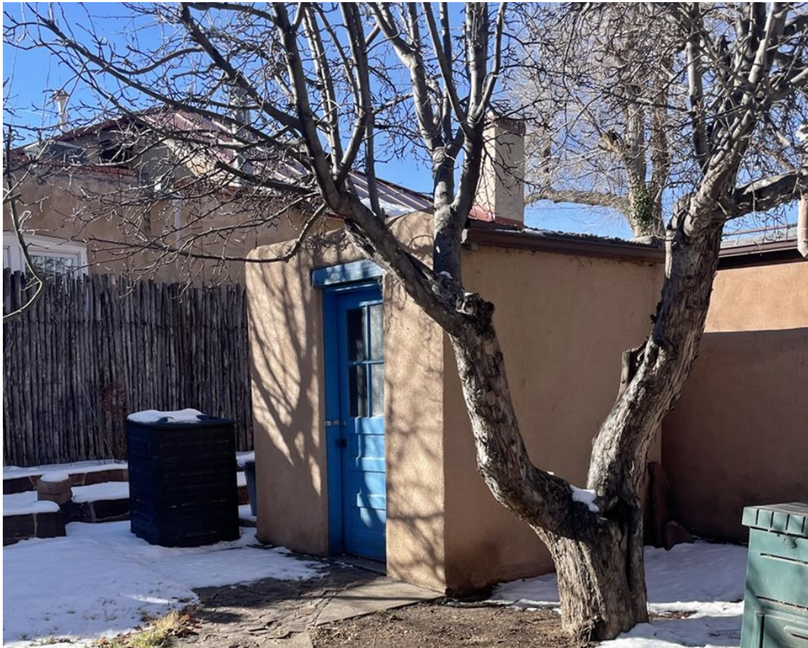
Photo 19: Shed. Camera facing southwest.
