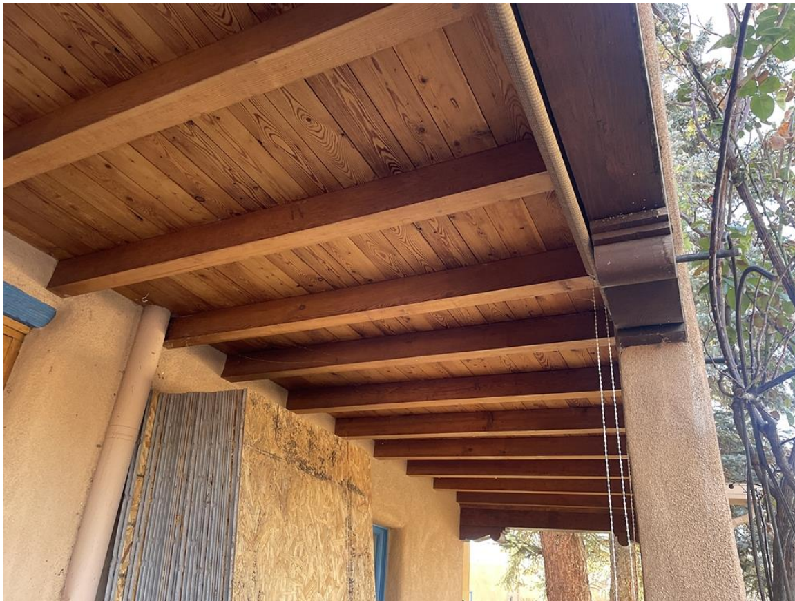
Photo 12: West elevation. Portal decking. Camera facing up.
