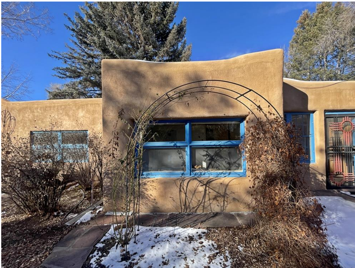
Photo 6: East elevation. South end of original building in foreground. Camera facing west.
