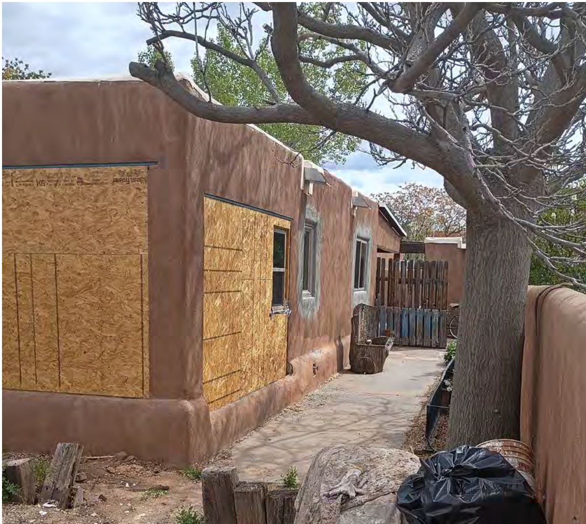
Photo 10: West elevation. Camera facing southeast.
