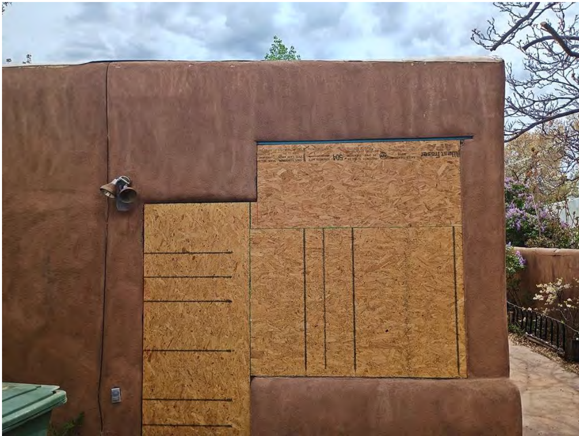
Photo 9: North façade, former entry and window of solarium filled in with OSB sheathing. Camera facing south.
