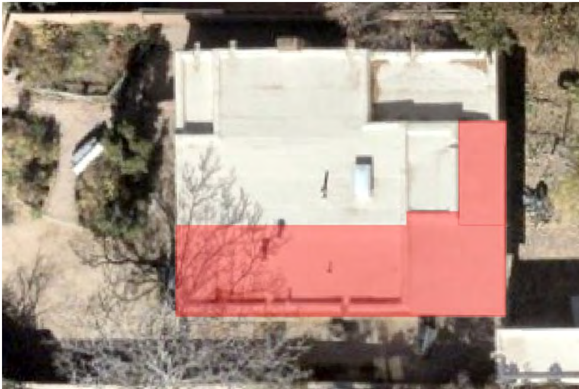
Figure 1: 2025 satellite view of 247 Barela Street. Red indicates new mass and/or roofed porch areas constructed after 1978.
