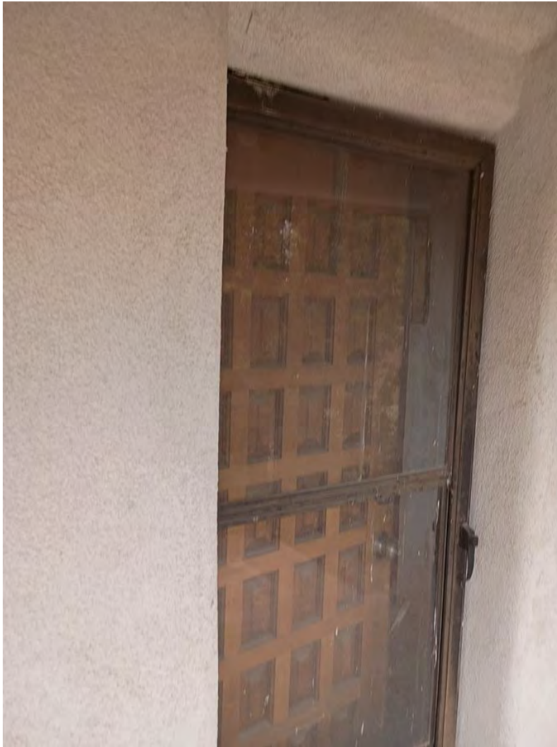
Photo 7: North façade entry portal, entry door. Camera facing southwest.
