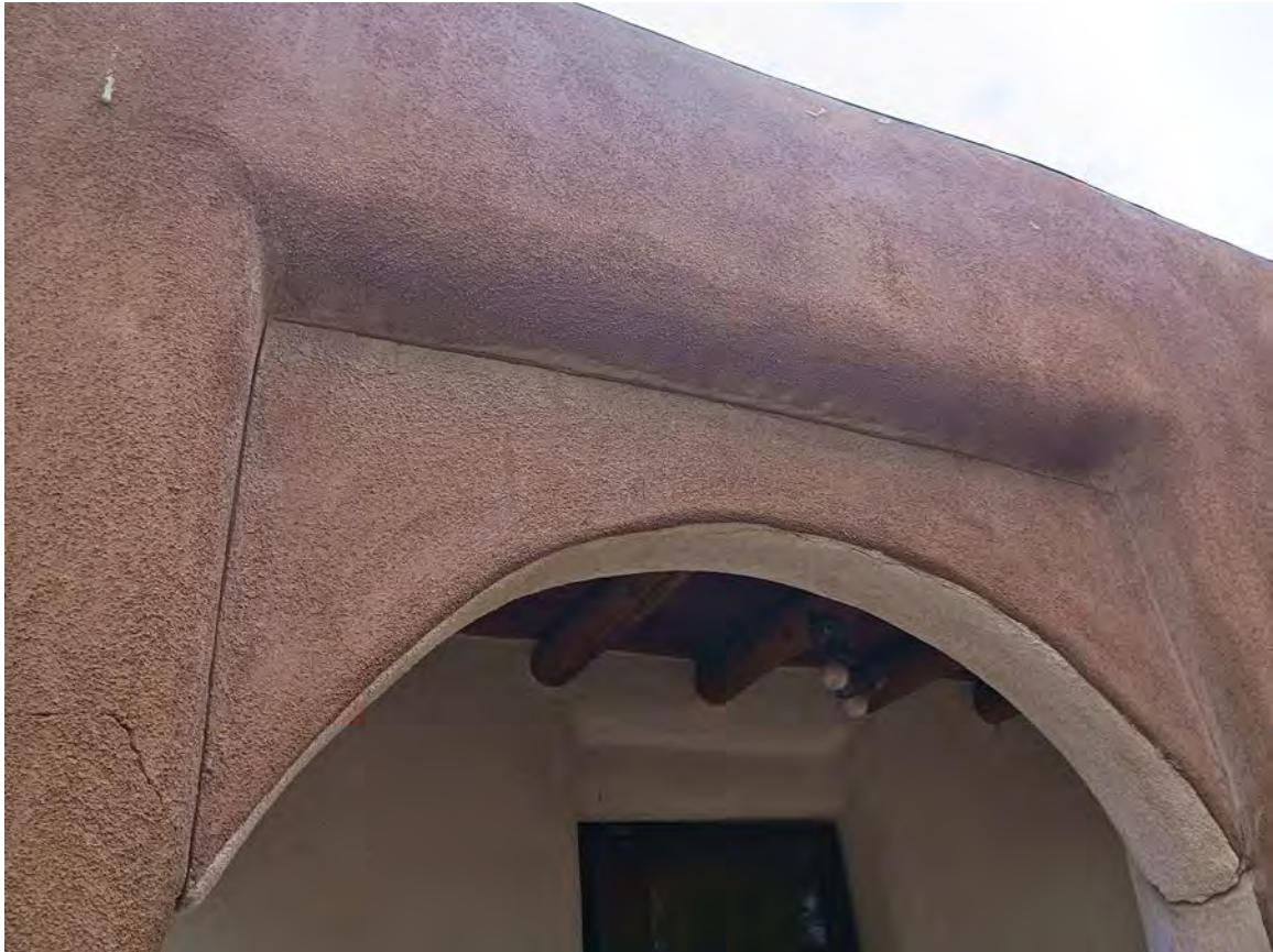
Photo 6: North façade entry portal, probable later arch insert. Camera facing up.
