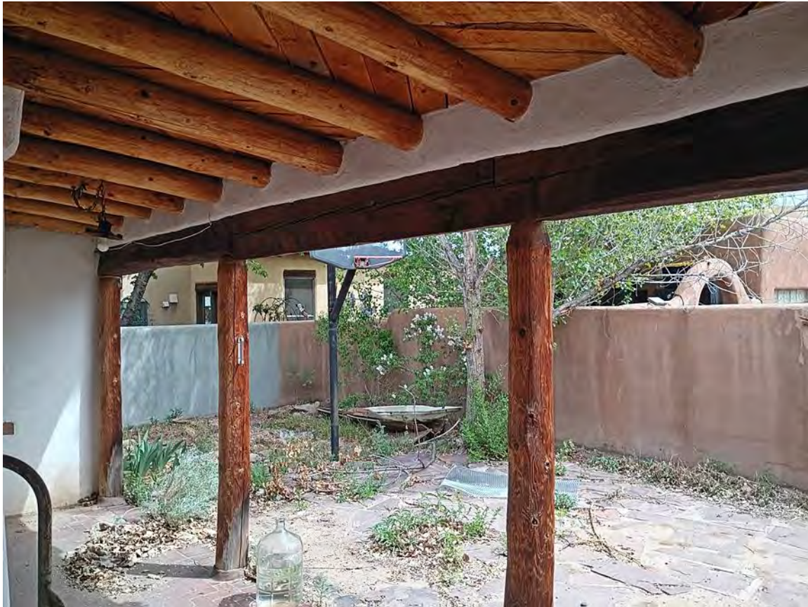
Photo 13: South elevation portal. Camera facing southeast.
