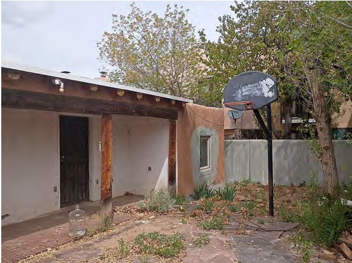
Photo 14: South elevation, east end. Note replaced window. Camera facing northeast.
