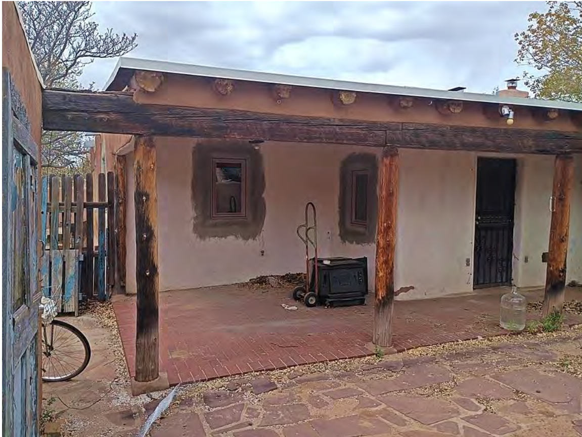
Photo 12: South elevation, west end. Note replaced windows. Camera facing northeast.
