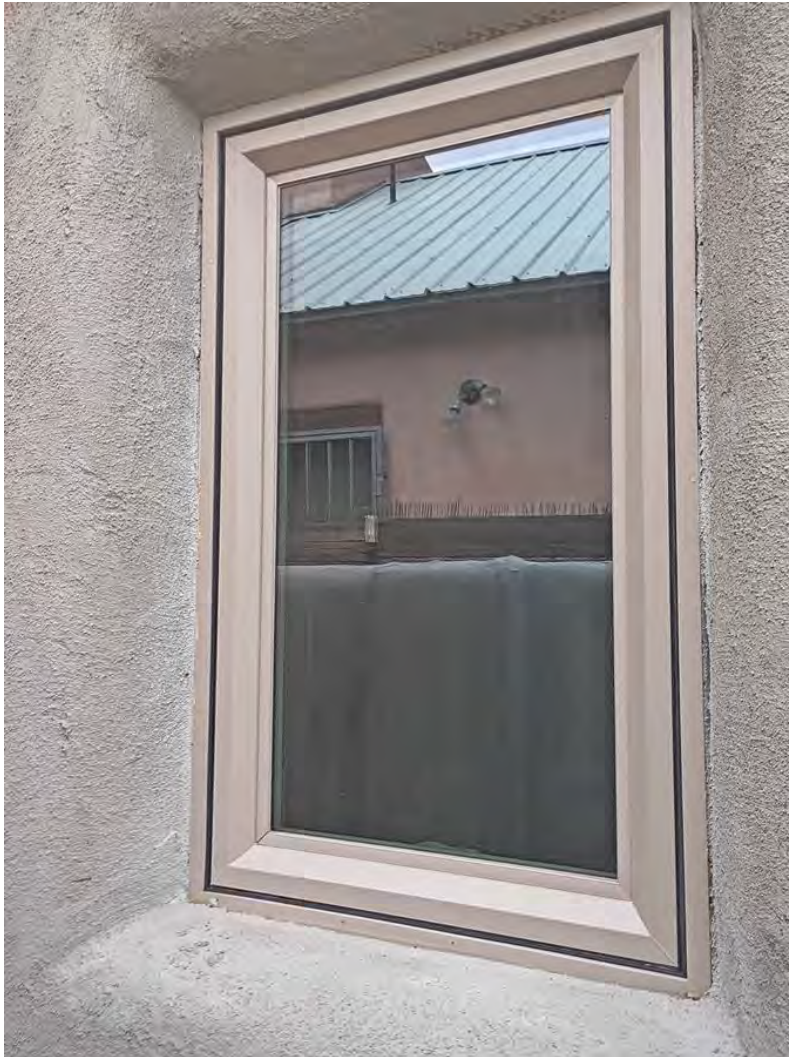
Photo 17: East elevation, replaced window. Camera facing southeast.
