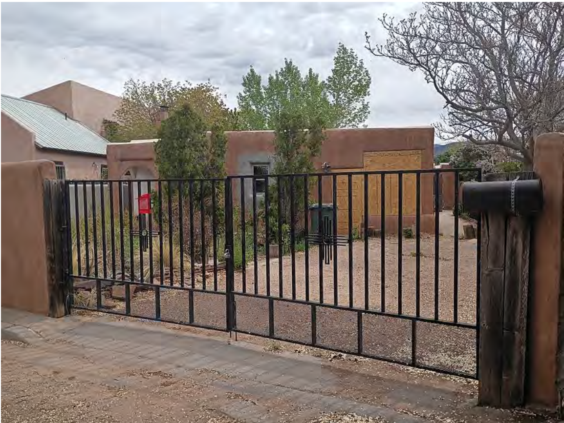
Photo 2: Non-historic vehicular gate and setting. Camera facing southeast.
