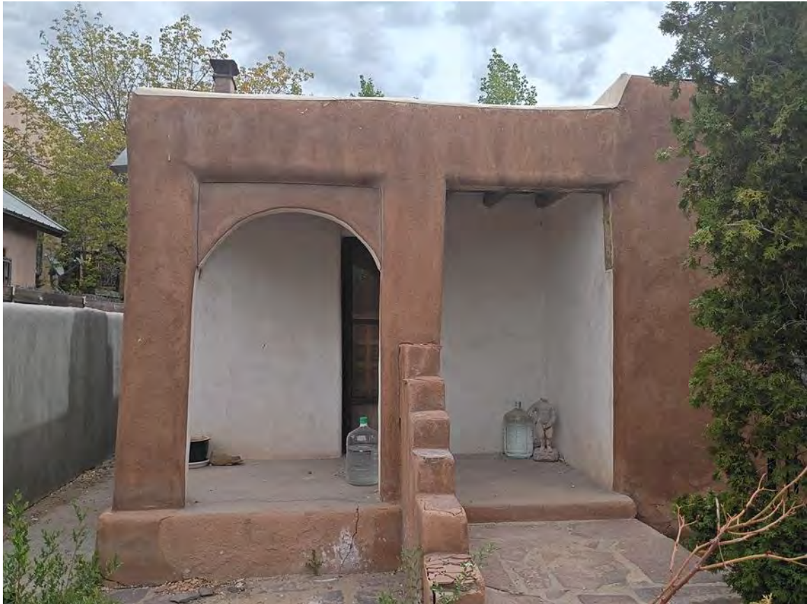
Photo 3: North façade entry portal. Camera facing south.
