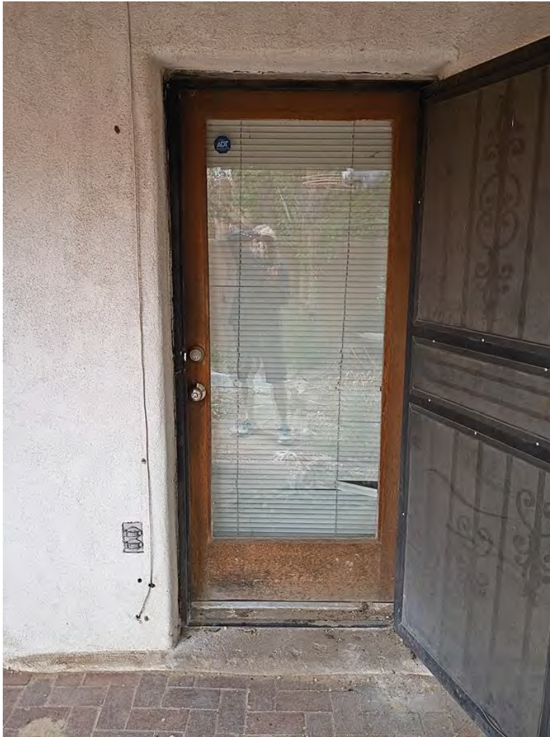
Photo 15: South elevation entry door. Camera facing north.
