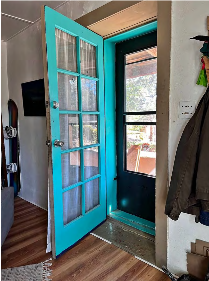
Photo 5: East (front façade), entry door. Camera facing northeast.
