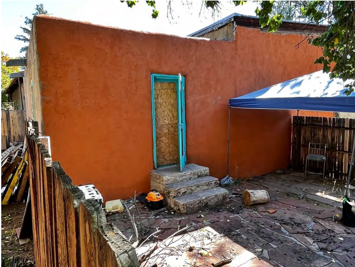
Photo 16: West elevation. Camera facing southeast.
