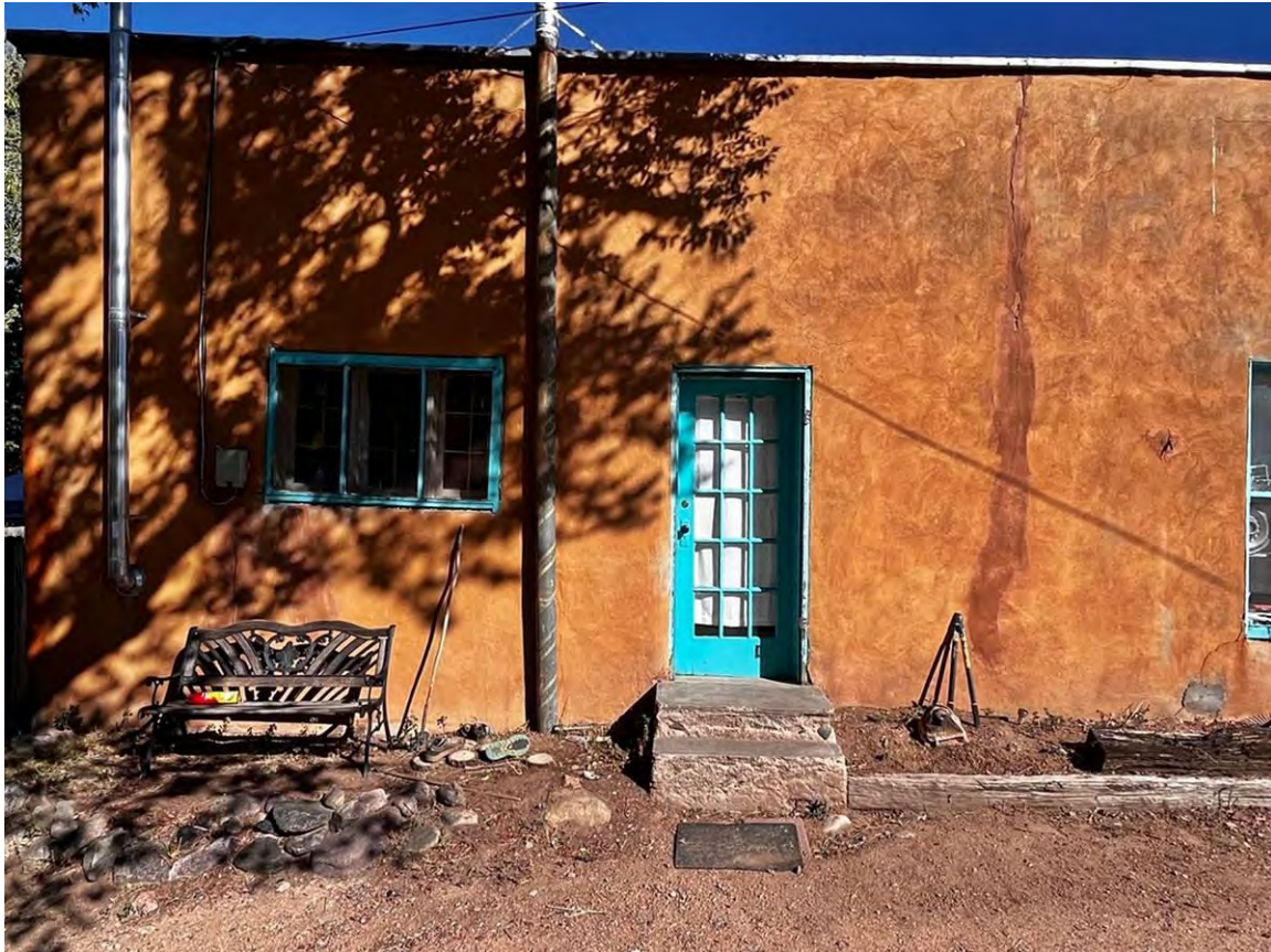
Photo 15: South elevation. End (west) apartment. Camera facing north.
