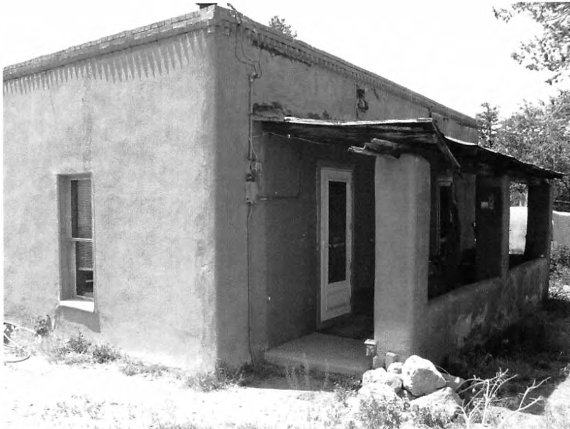
3. View Northwest of 1930s addition (ArcCom June 5, 2007).
