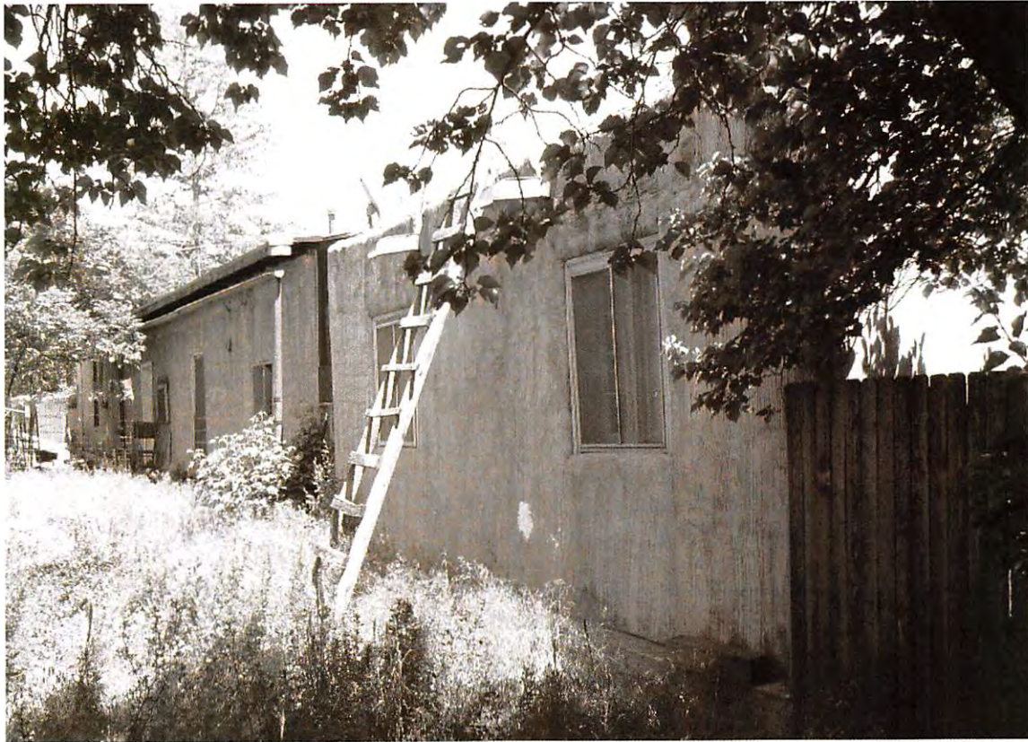
6. View Southeast of North elevation room additions (ArcCom June 5, 2007).
