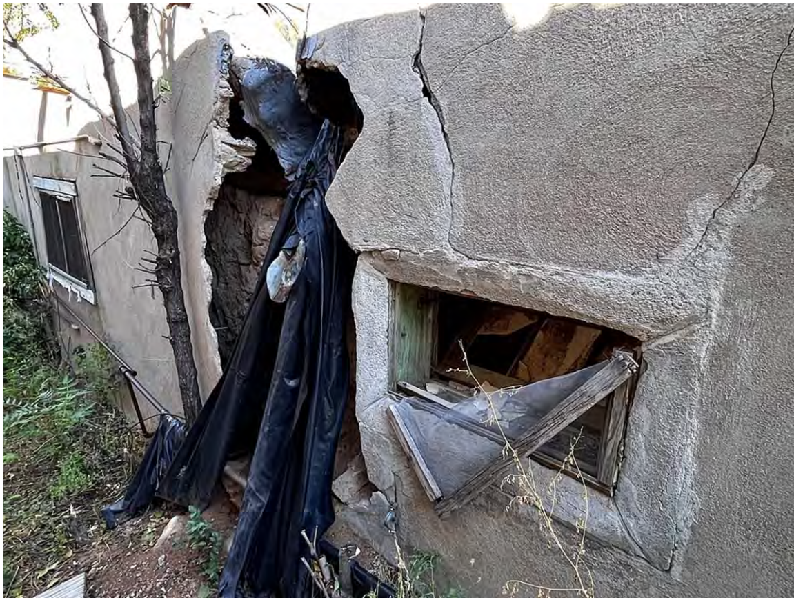
Photo 25: South elevation. Camera facing northwest.
