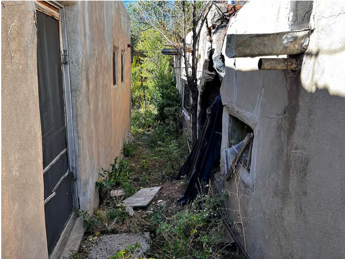
Photo 30: North elevation, left. Camera facing west.
