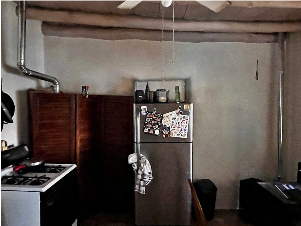
Photo 13: Midde apartment. Example of viga roof extension. Camera facing west.
