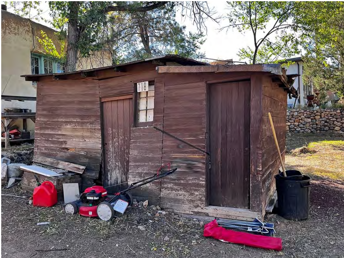
Photo 37: North and west elevations. Camera facing southeast.
