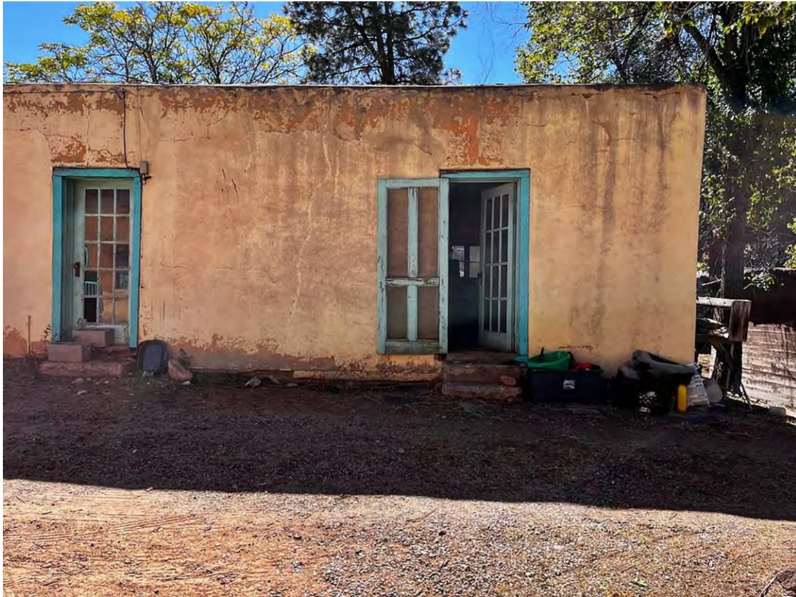
Photo 24: North elevation, west end. Camera facing south.
