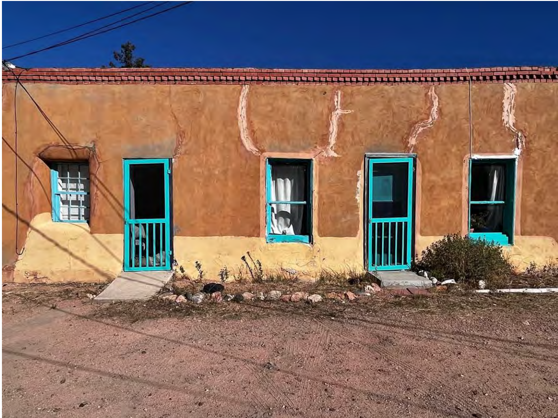
Photo 12: South elevation. Front (east) and middle apartments. Camera facing north.
