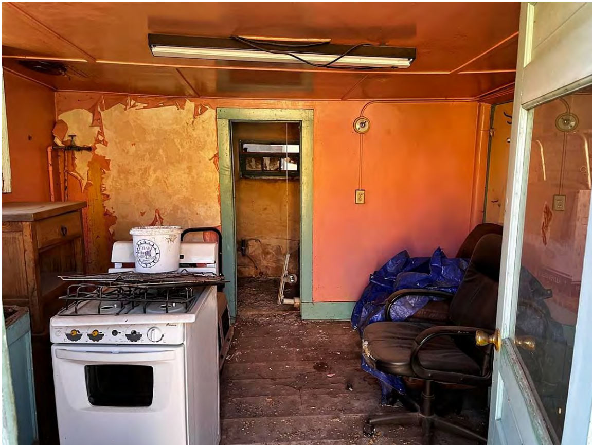
Photo 26: Kitchen. Camera facing south.
