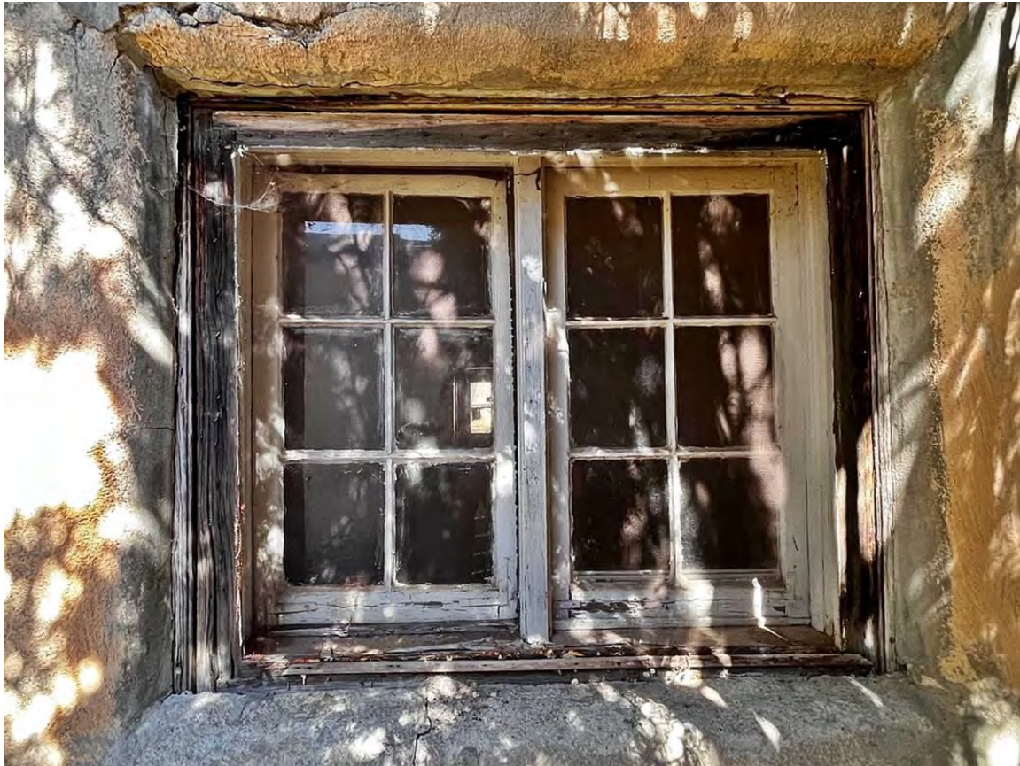
Photo 34: South elevation, east end. Camera facing north.
