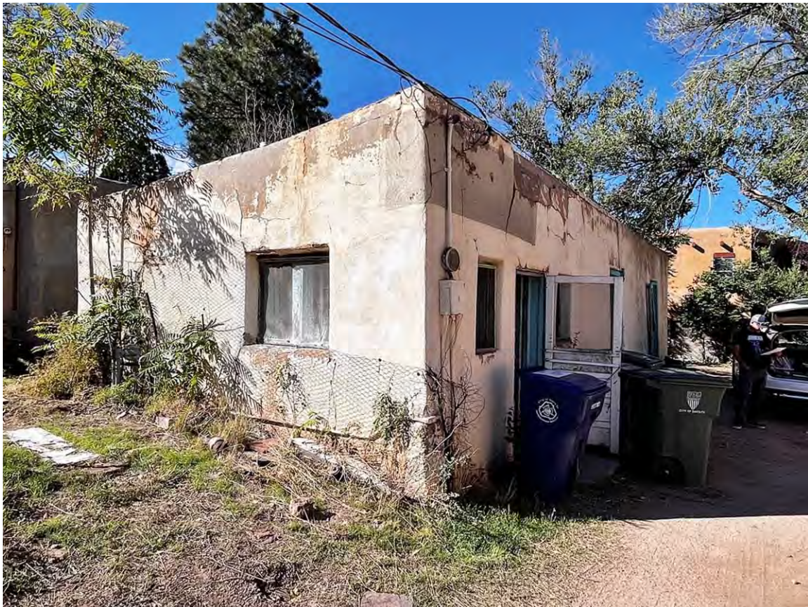
Photo 22: East and north elevations. Camera facing southwest.
