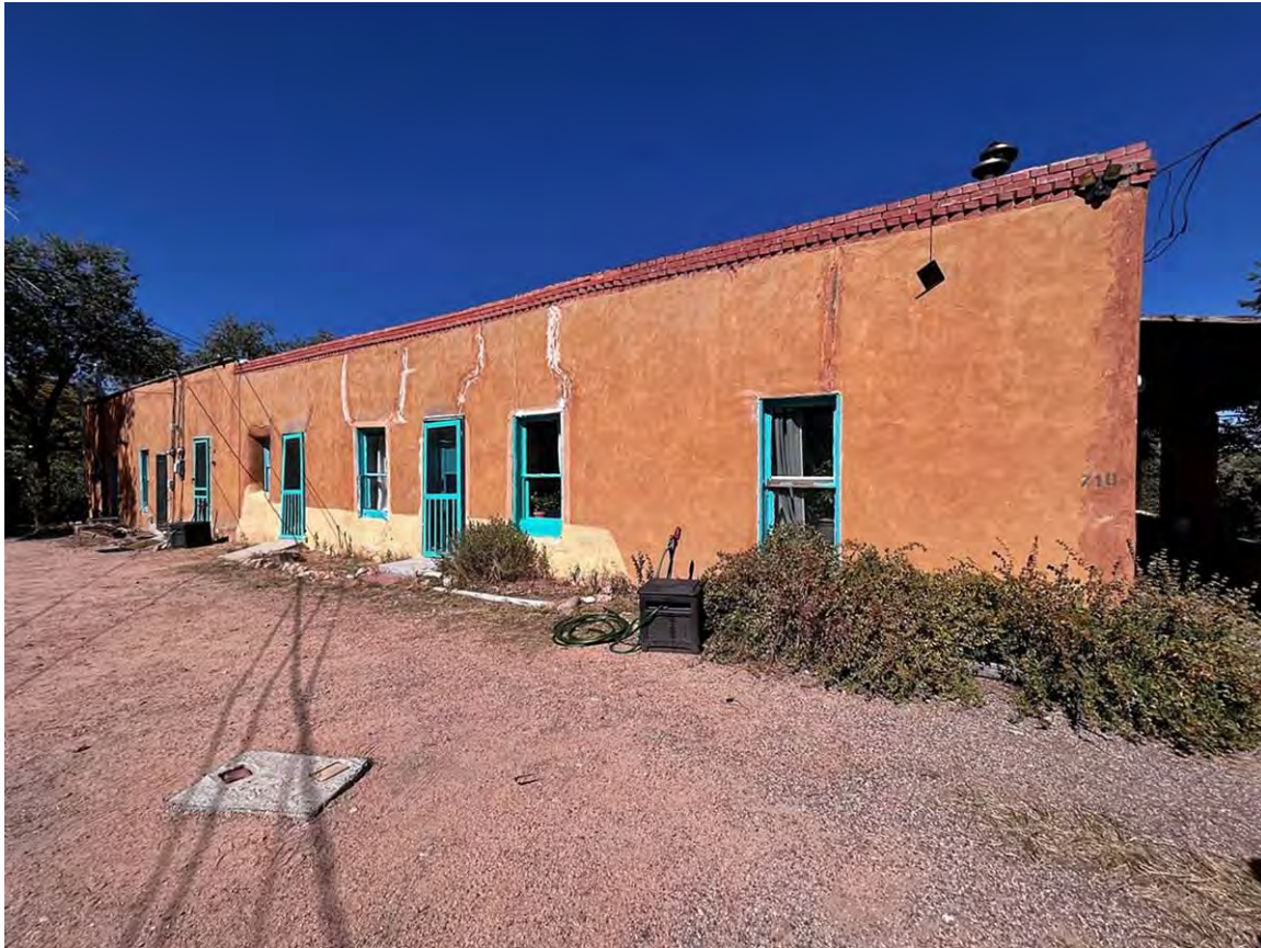
Photo 9: South elevation. Camera facing northwest.
