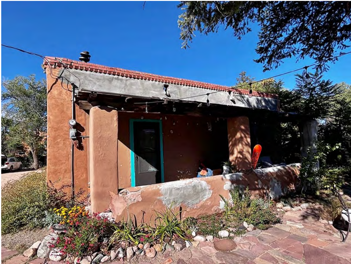
Photo 4: East (front façade). Camera facing northwest.
