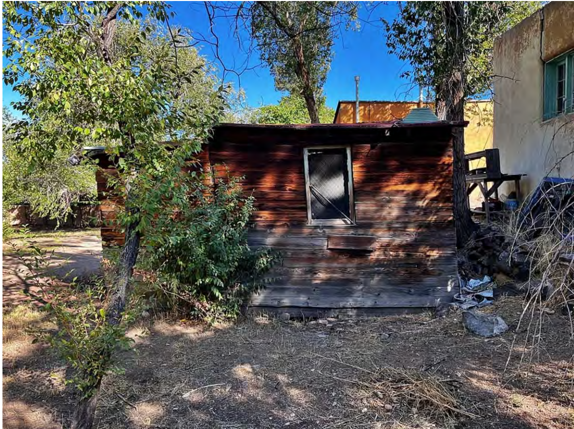
Photo 38: South elevation. Camera facing north.
