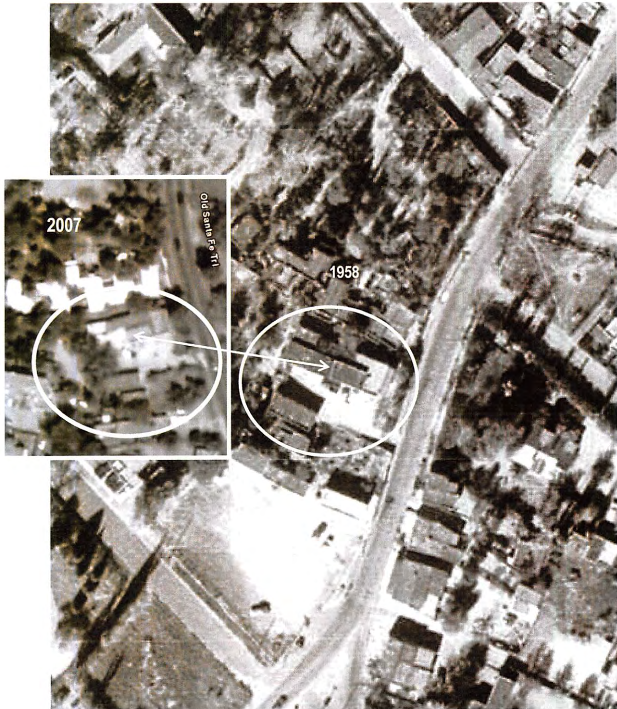
1958 NMDOT aerial photograph with 2007 Google image superimposed. Pointer indicates oldest part of building.
