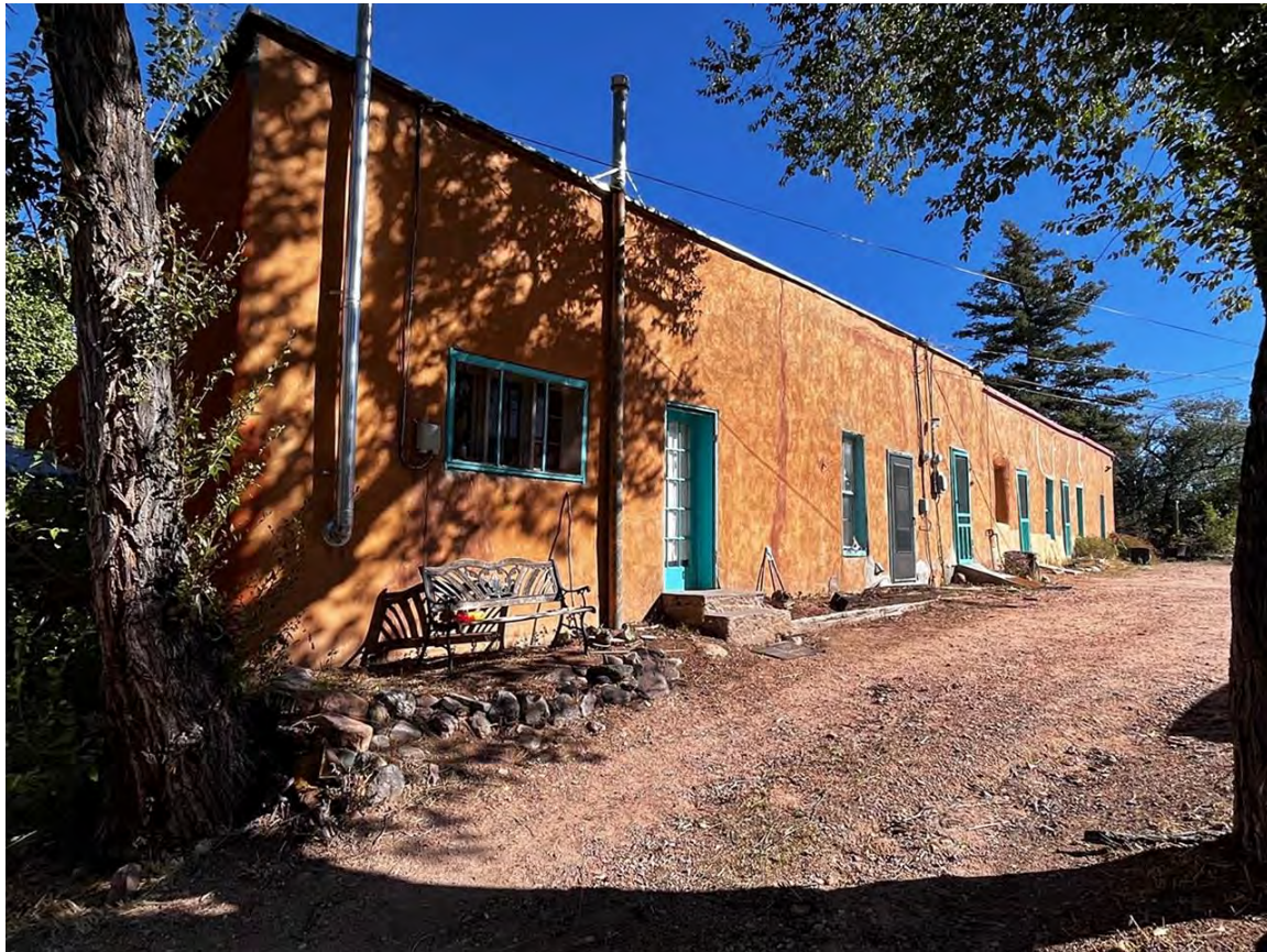
Photo 11: South elevation. Camera facing northeast.
