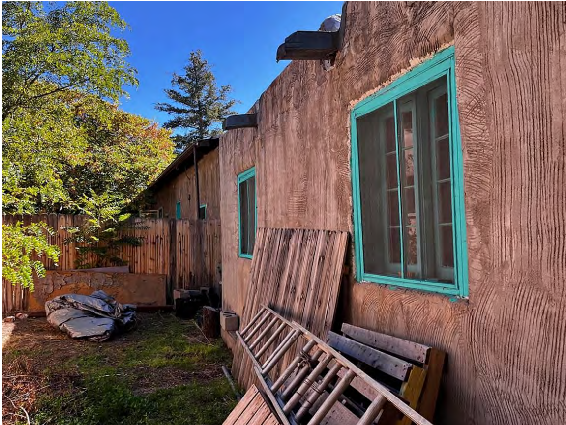
Photo 17: North elevation, northwest corner. Camera facing southeast.
