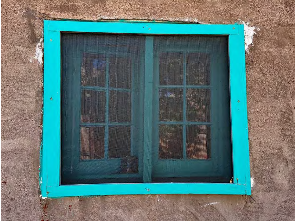
Photo 18: South elevation. Window at end (west) apartment. Camera facing south.
