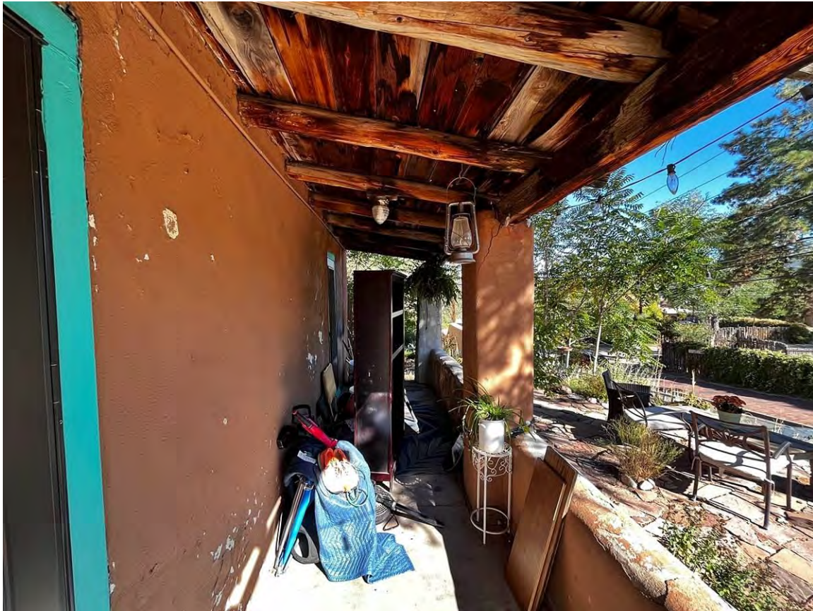
Photo 6: East (front façade), portal. Camera facing north.
