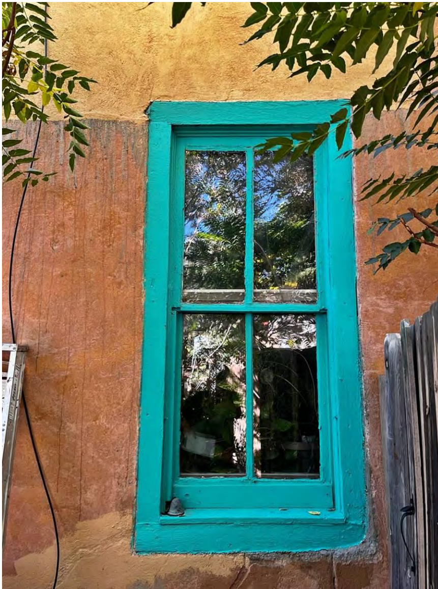
Photo 7: North elevation, northeast corner window. Camera facing up.
