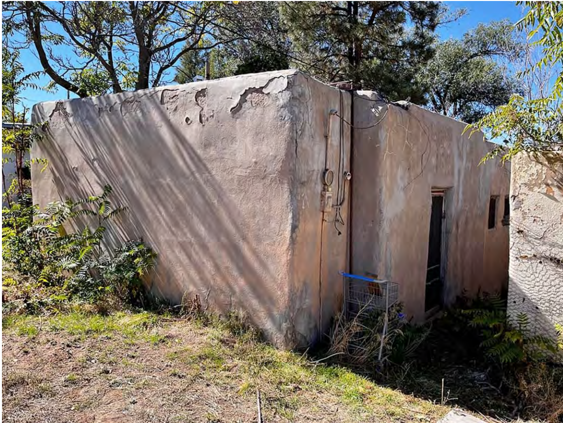
Photo 29: East and north elevations. Camera facing southwest.
