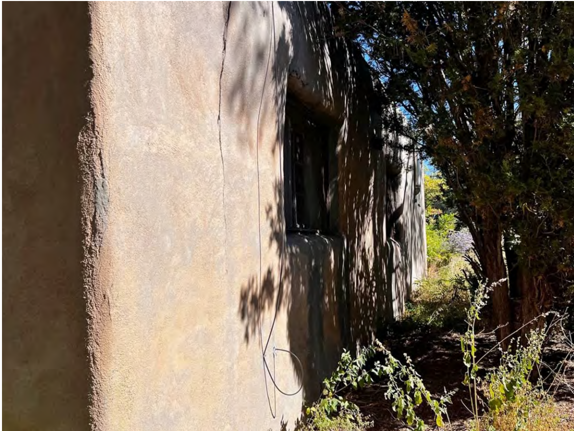
Photo 33: South elevation. Camera facing east.
