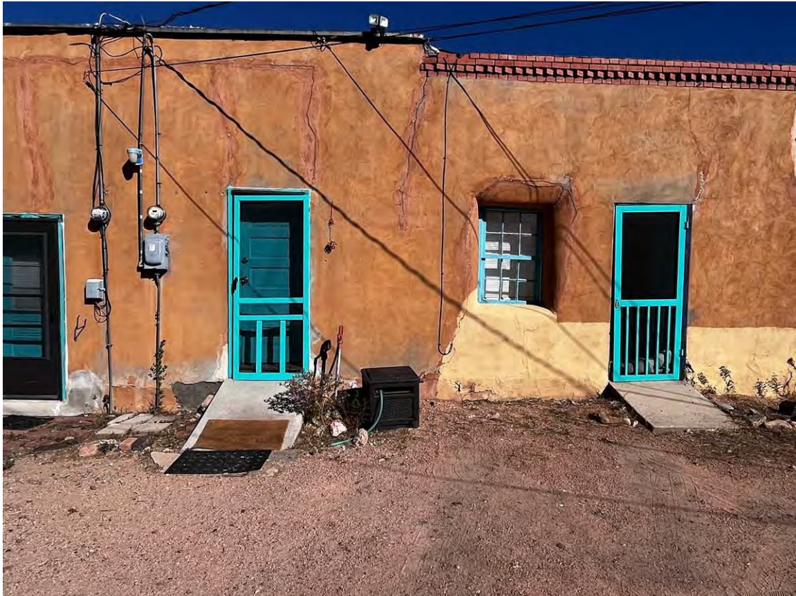
Photo 14: South elevation. End (west) apartment starts at left. Camera facing north.
