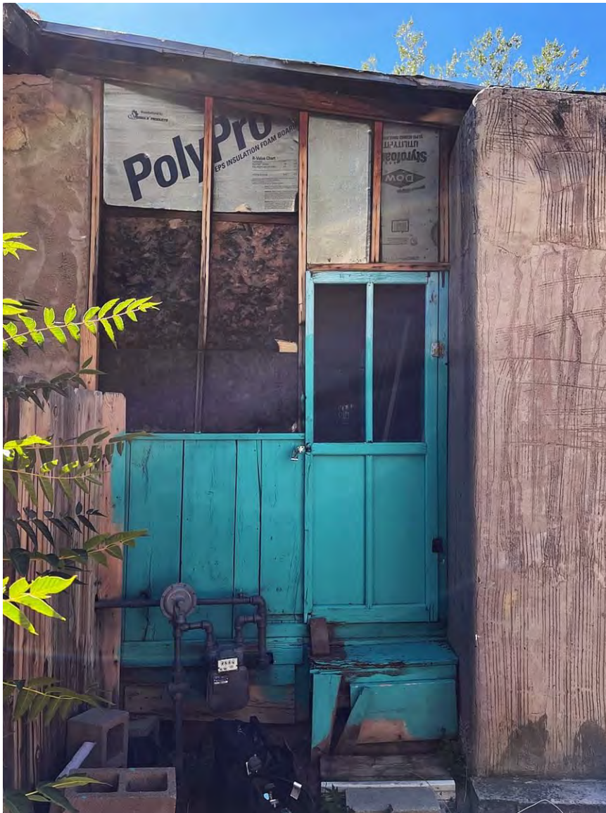
Photo 20: South elevation. Storage area. Camera facing south.
