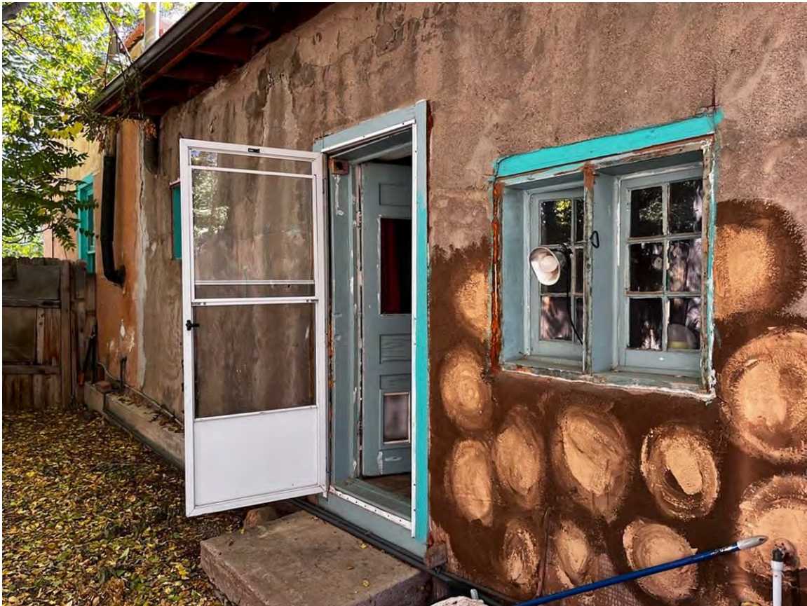
Photo 21: South elevation. Front (east) apartment. Camera facing southeast.
