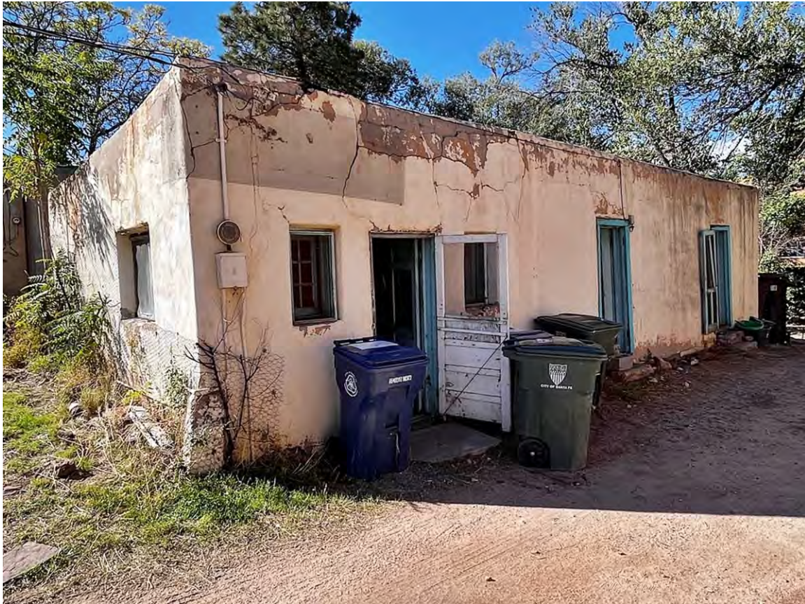
Photo 23: North elevation. Camera facing southwest.
