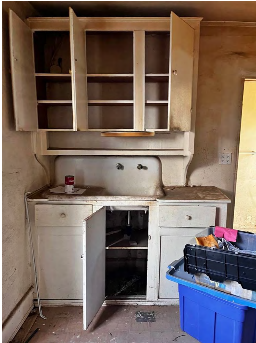
Photo 35: Kitchen. Camera facing south.
