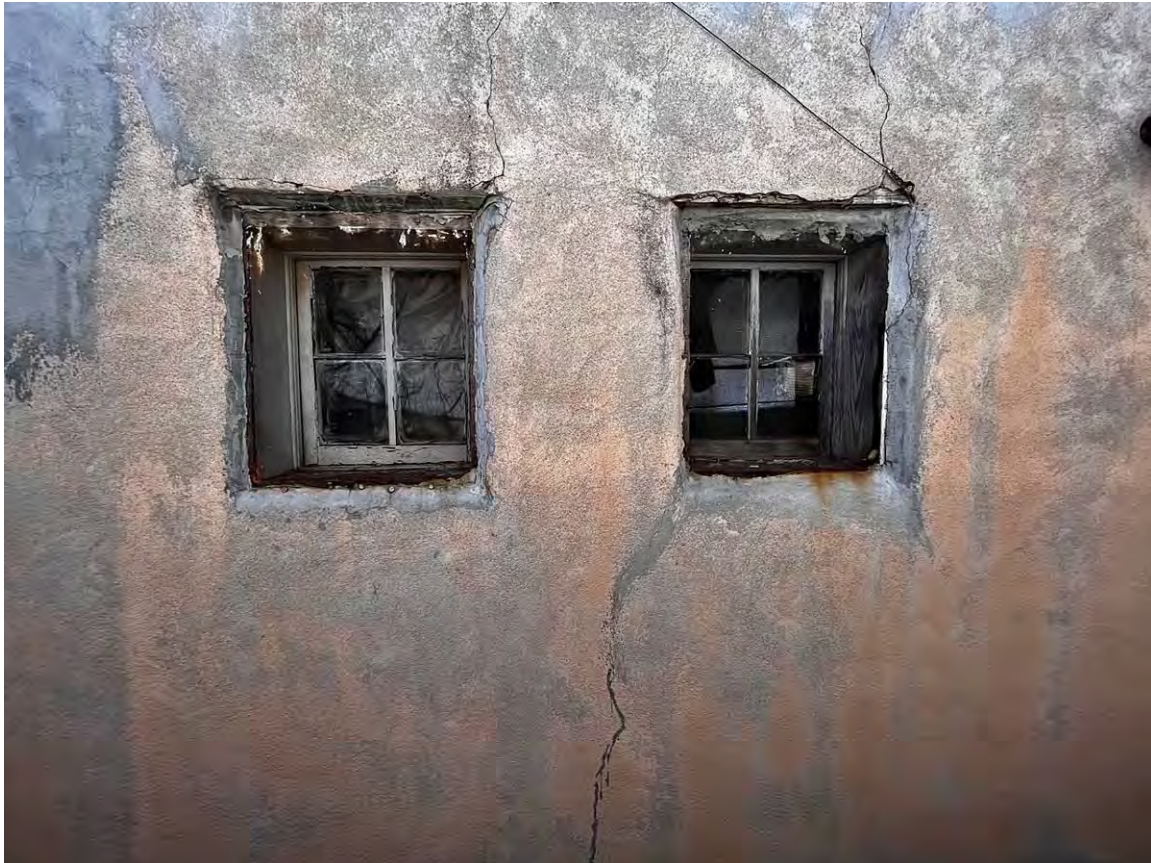
Photo 31: North elevation, west end. Camera facing south.
