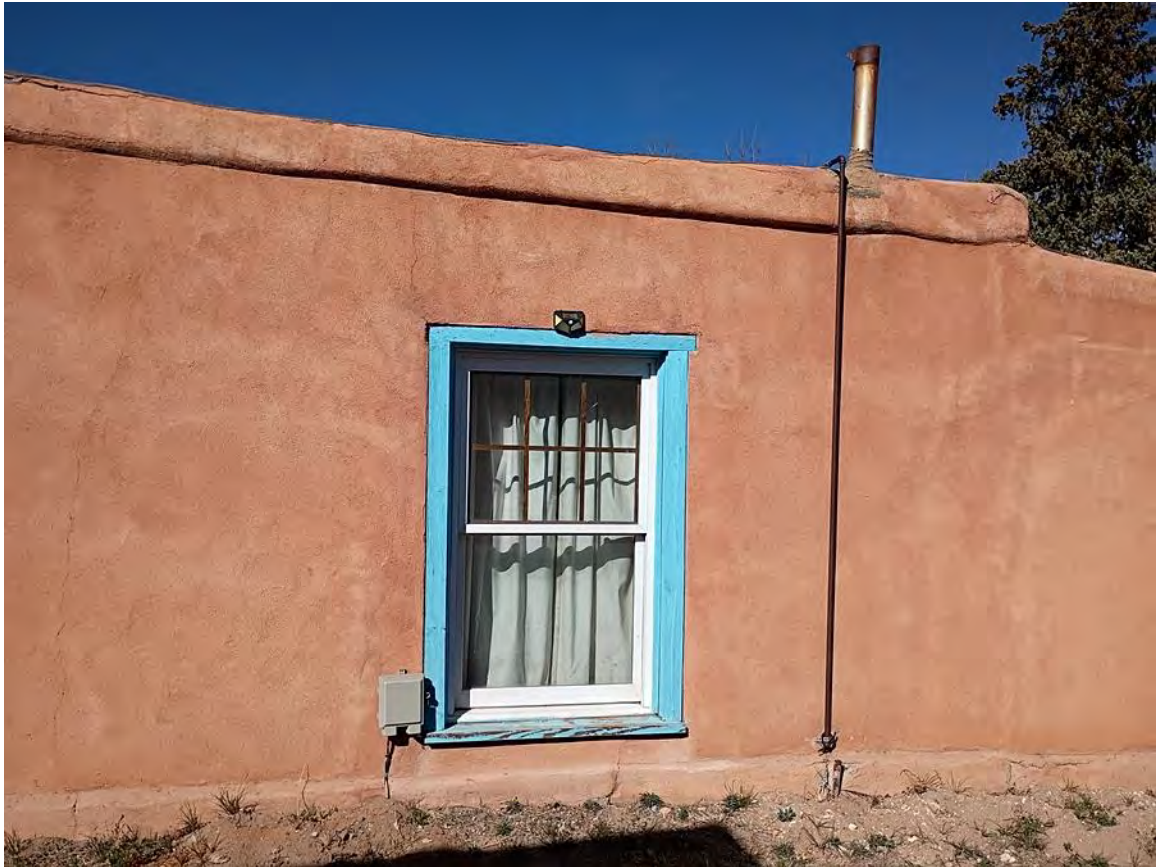
Photo 8: East elevation. Window detail. Camera facing west.
