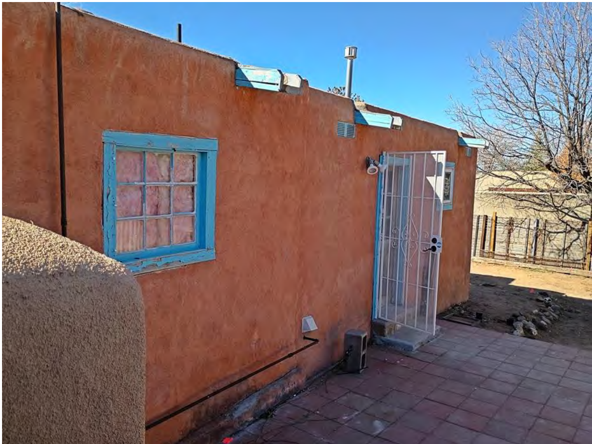
Photo 6: North elevation, Camera facing southwest.
