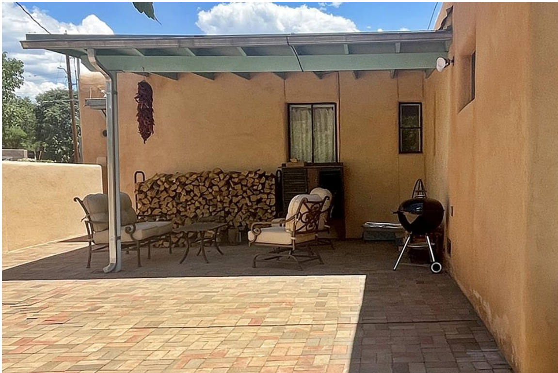
Photo 10: West elevation. Original section. Camera facing east.
