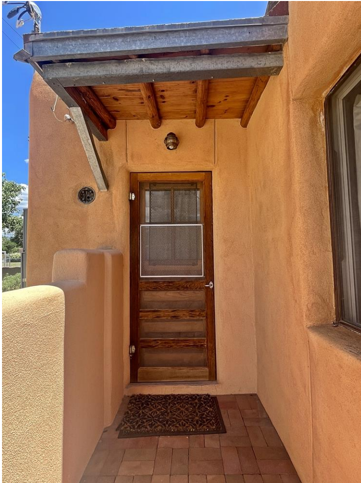
Photo 9: West elevation. Laundry room entry. Camera facing east.
