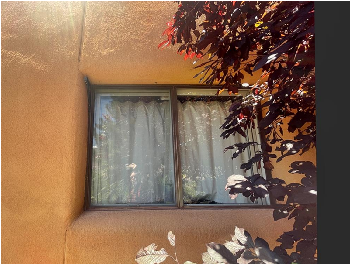
Photo 6: East (front) façade. Window and stucco detail. Camera facing west.
