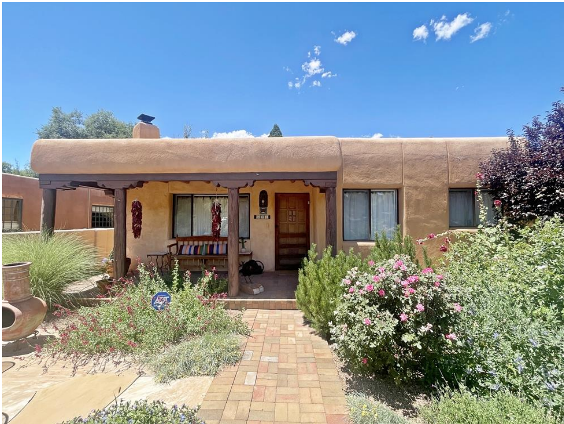
Photo 2: East (front) façade. Camera facing west.
