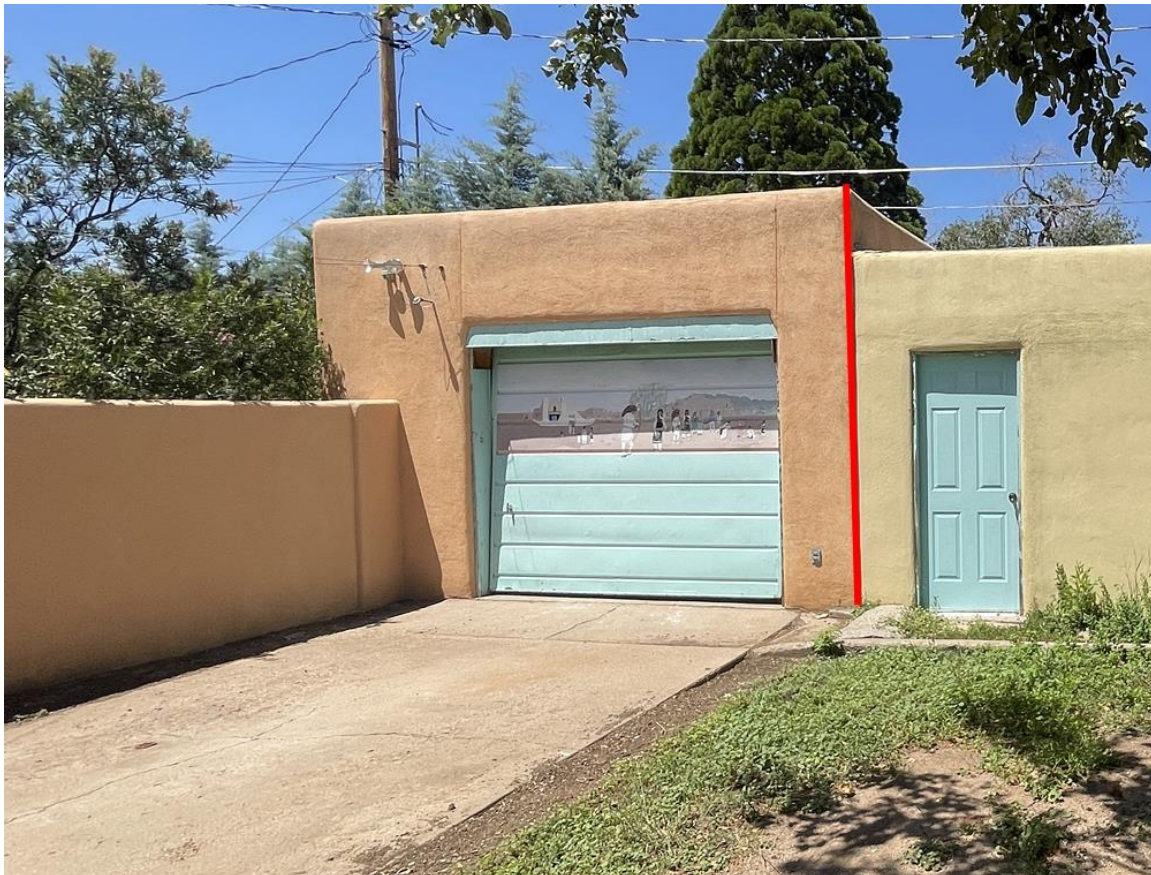
Photo 15: Garage (left of red line). Camera facing southwest.
