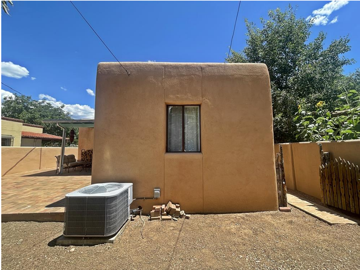
Photo 11: West elevation. Primary bedroom addition. Camera facing east.
