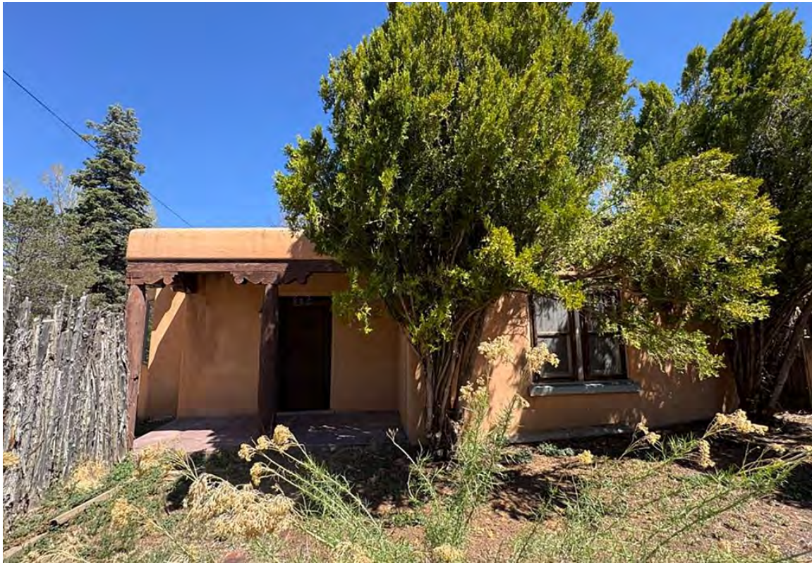
Photo 4: South (front) elevation. Camera facing north. Aviva Baumann, April 23, 2025.
