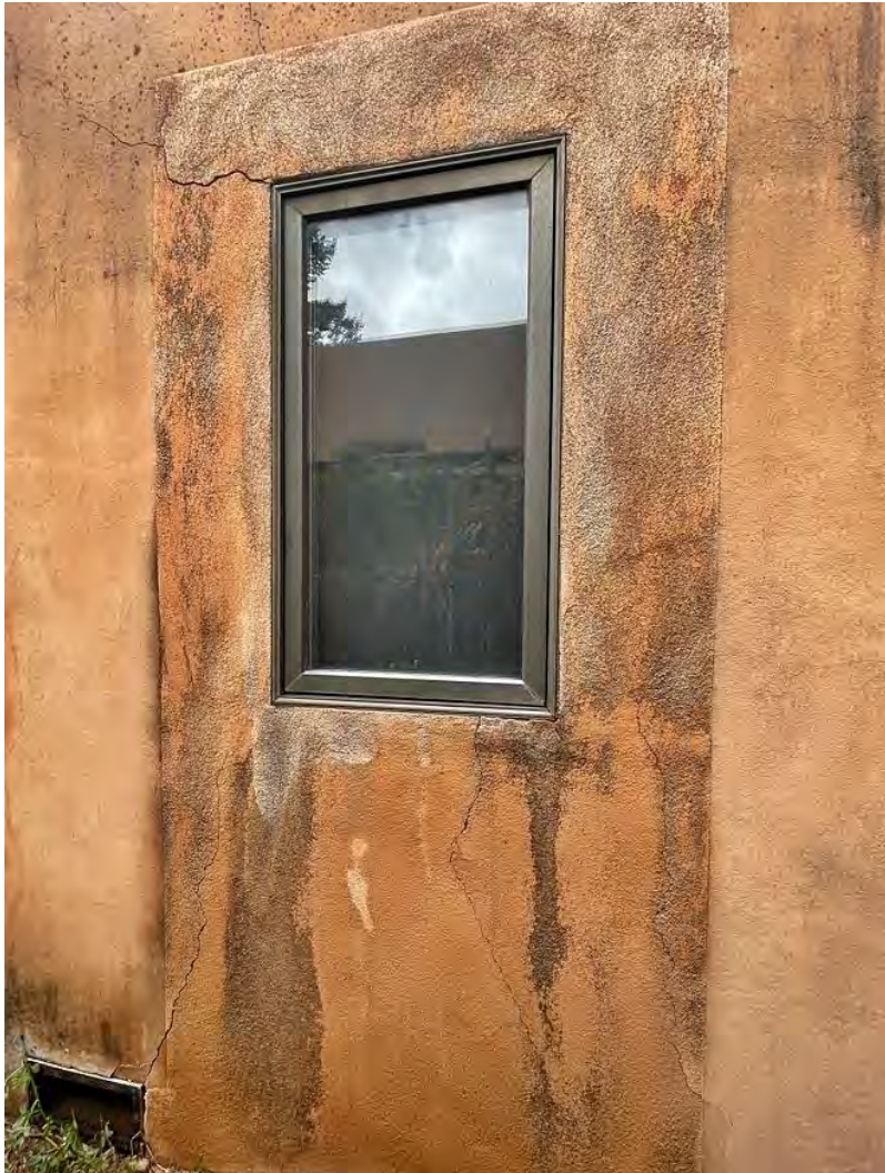
Photo 19: East elevation. Altered window at bedroom. Camera facing southwest.
