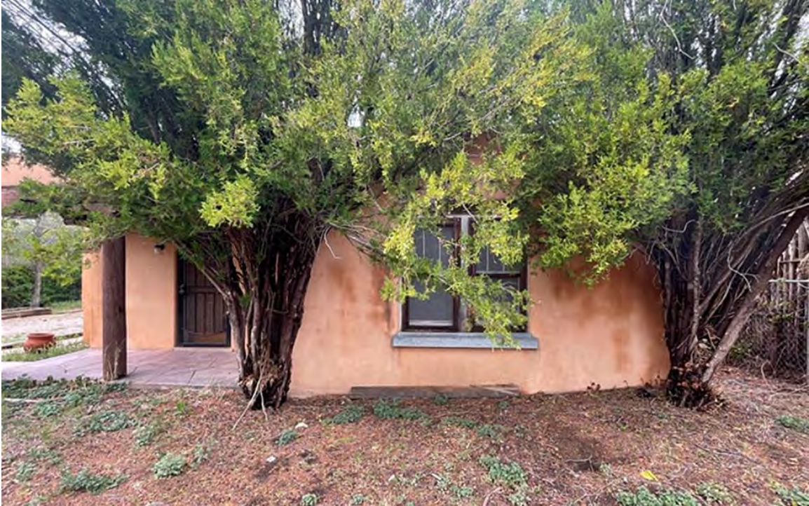
Photo 7: South elevation. Window at bedroom. Camera facing north.
