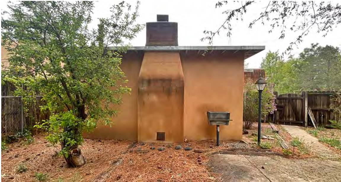
Photo 14: North elevation. Camera facing south.
