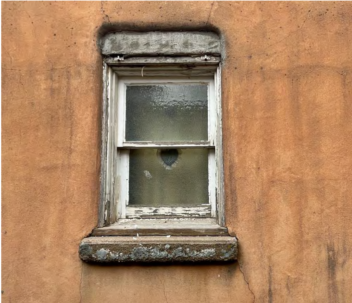
Photo 17: East elevation. Window at bathroom. Camera facing west.
