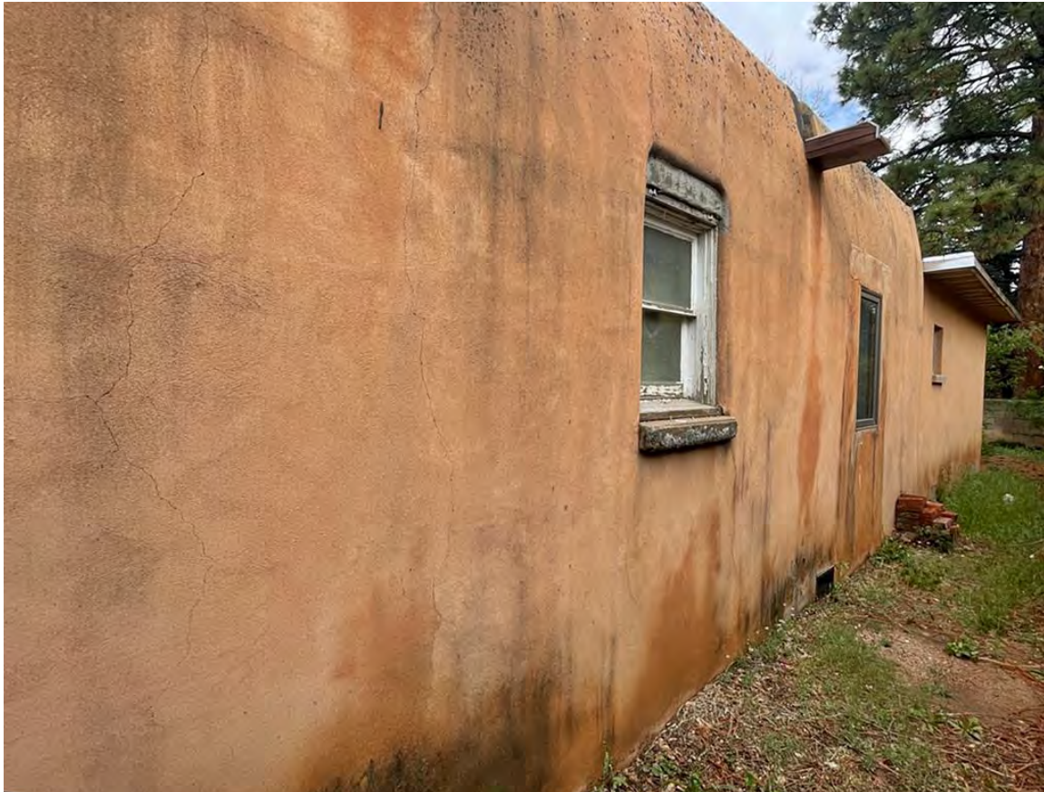
Photo 18: East elevation oblique from midpoint. Camera facing northwest.
