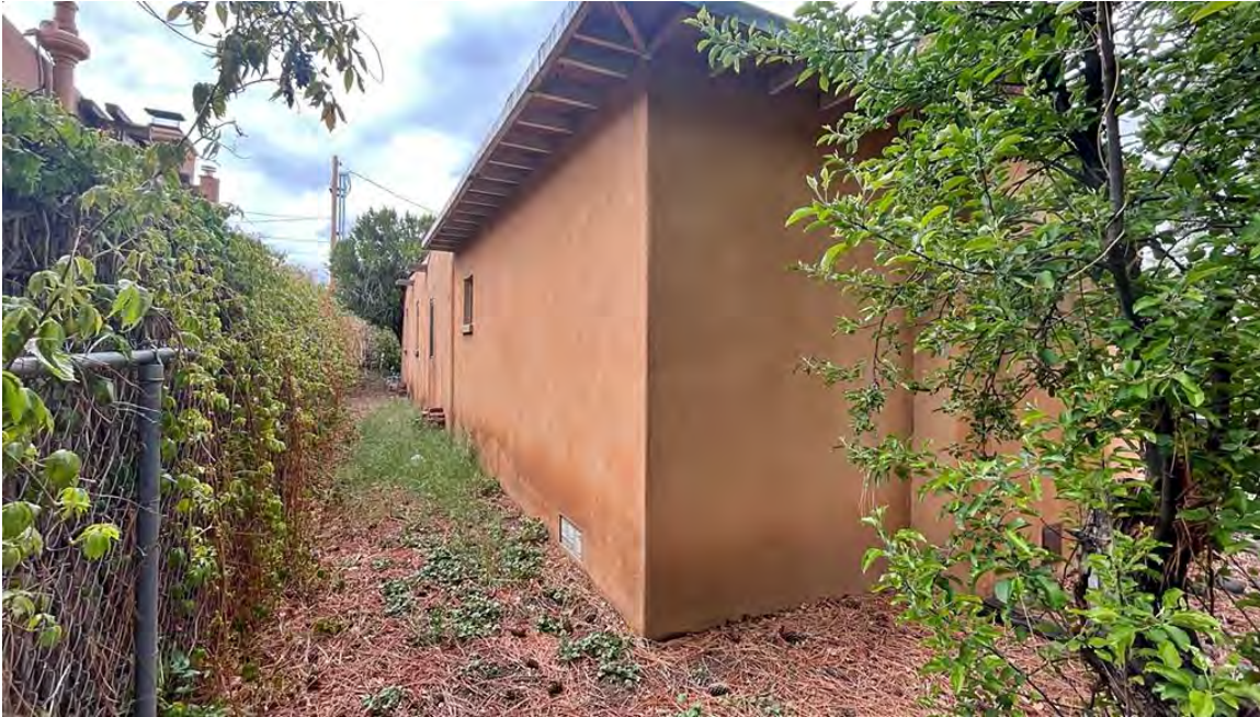
Photo 20: East elevation oblique from north end. Addition in foreground. Camera facing southwest.
