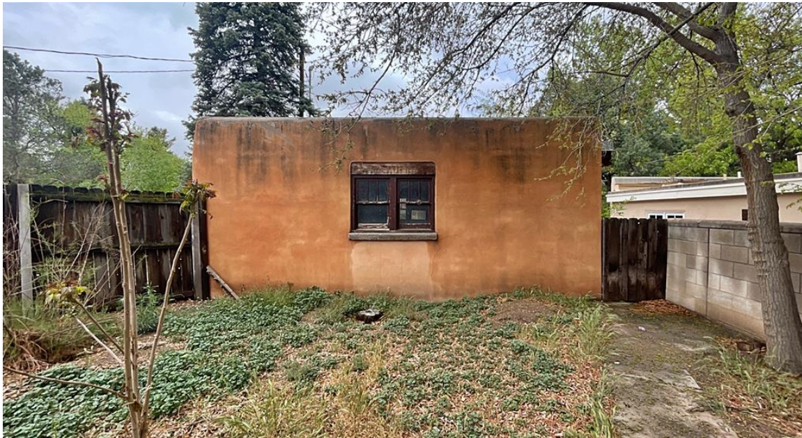
Photo 22: Garage. East elevation. Camera facing west.
