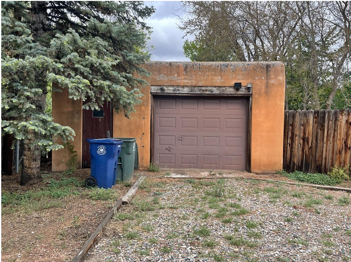
Photo 21: Garage. South elevation. Camera facing north.
