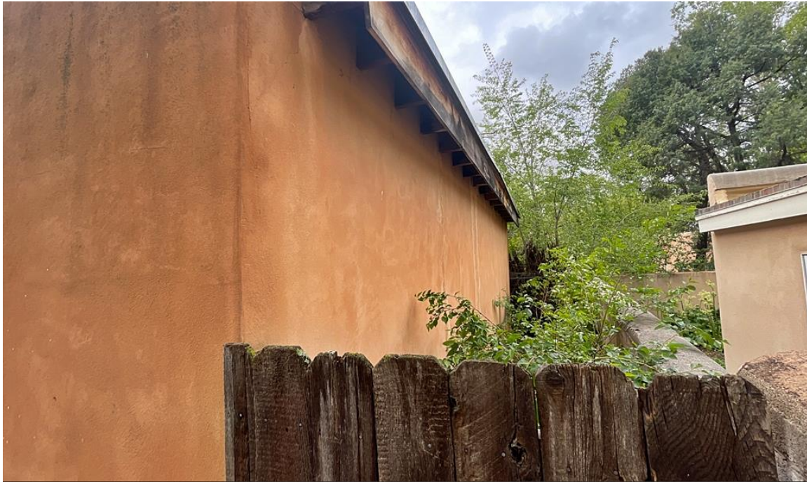
Photo 24: Garage. North elevation. Camera facing west.
