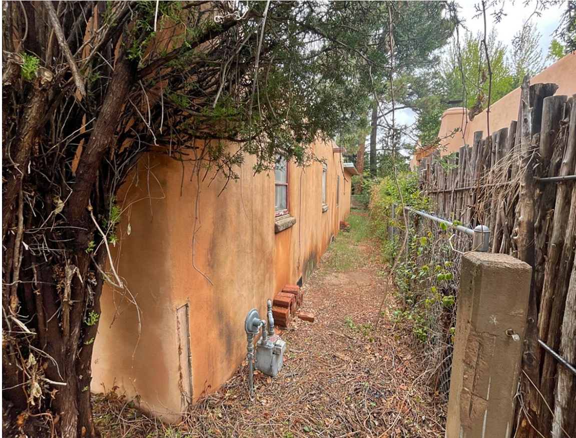
Photo 15: East elevation oblique from south end. Camera facing northwest.
