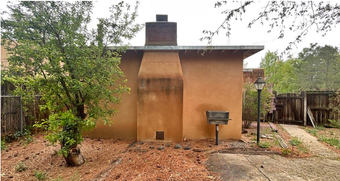
Photo 14: North elevation. Camera facing south.
