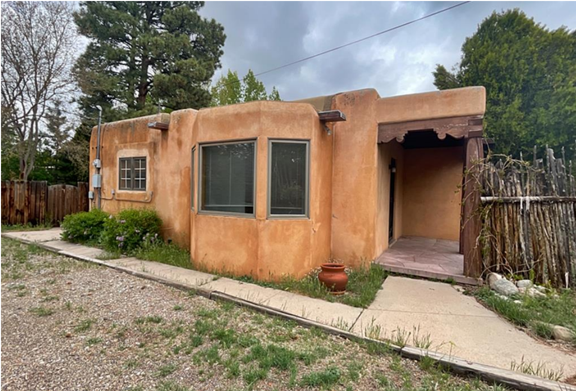
Photo 9: West elevation oblique. Camera facing northeast.
