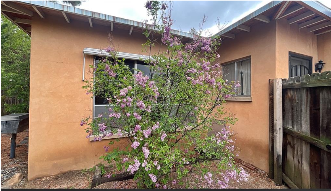
Photo 12: West elevation. Addition. Camera facing southeast.
