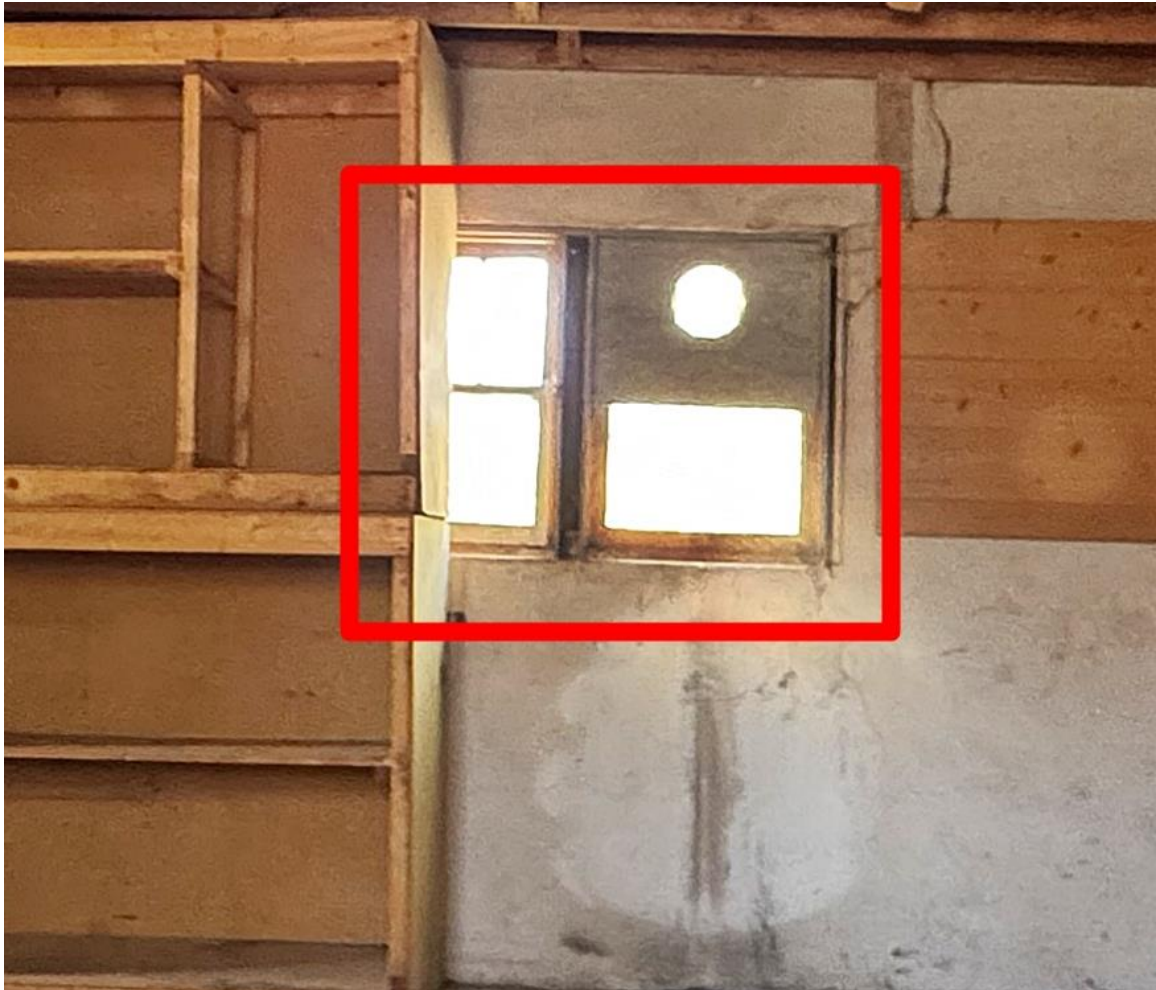
Photo 23: Garage. West elevation. Windows from the interior. Aviva Baumann, April 23, 2025.
