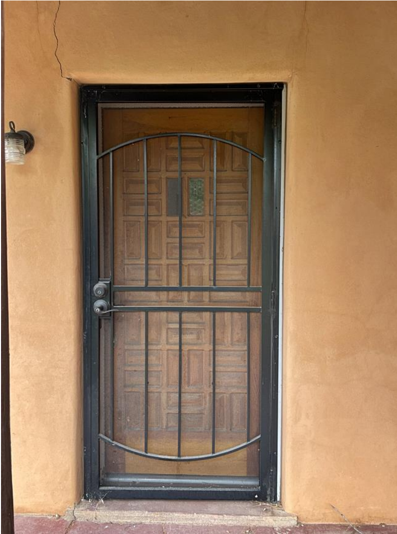
Photo 6: South elevation. Entry door. Camera facing north.
