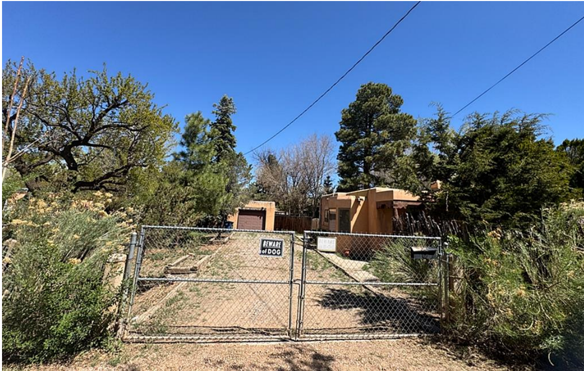
Photo 3: Setting of property. Camera facing north. Aviva Baumann, April 23, 2025.
