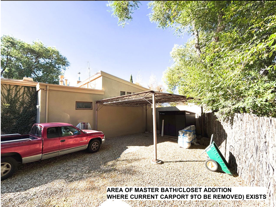
AREA OF MASTER BATH/CLOSET ADDITION WHERE CURRENT CARPORT 9TO BE REMOVED) EXISTS
