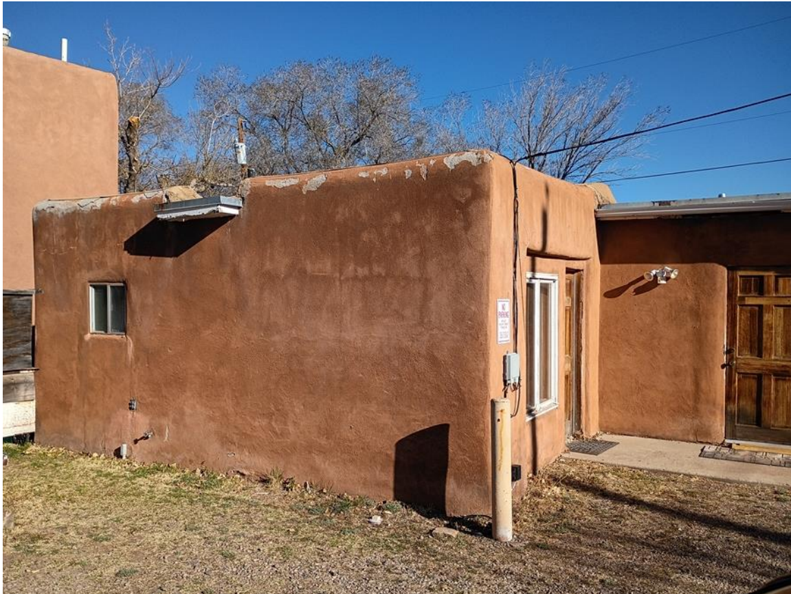
Photo 5: South elevation. Former garage. Camera facing northwest.
