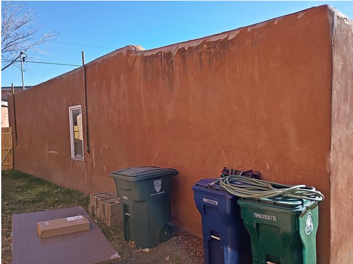
Photo 10: West elevation, including former garage and residence. Camera facing northeast.
