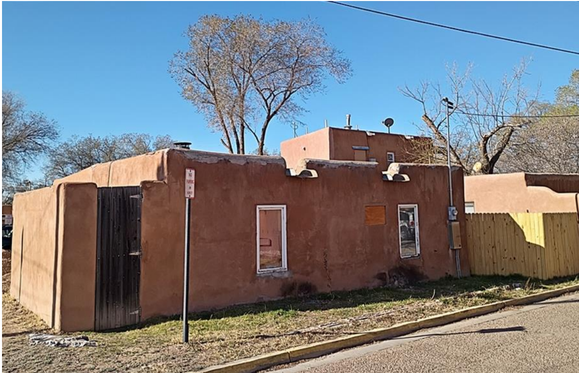
Photo 8: North elevation. Camera facing southwest.
