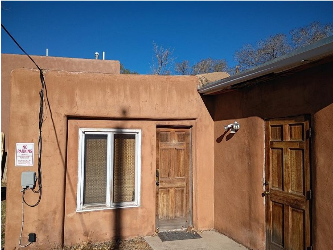
Photo 4: East elevation. Former garage infill fenestration. Camera facing northwest.
