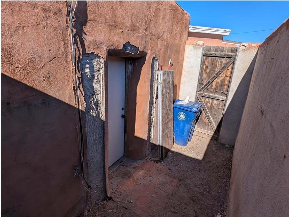
Photo 7: East elevation. Trash enclosure. Joey Ortiz, January 20, 2026.
