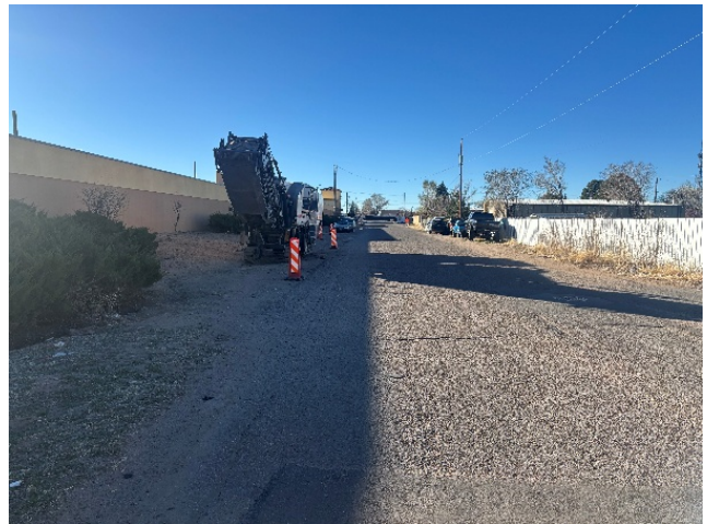
Figure 4 – View South on Cam. De Jacobo
