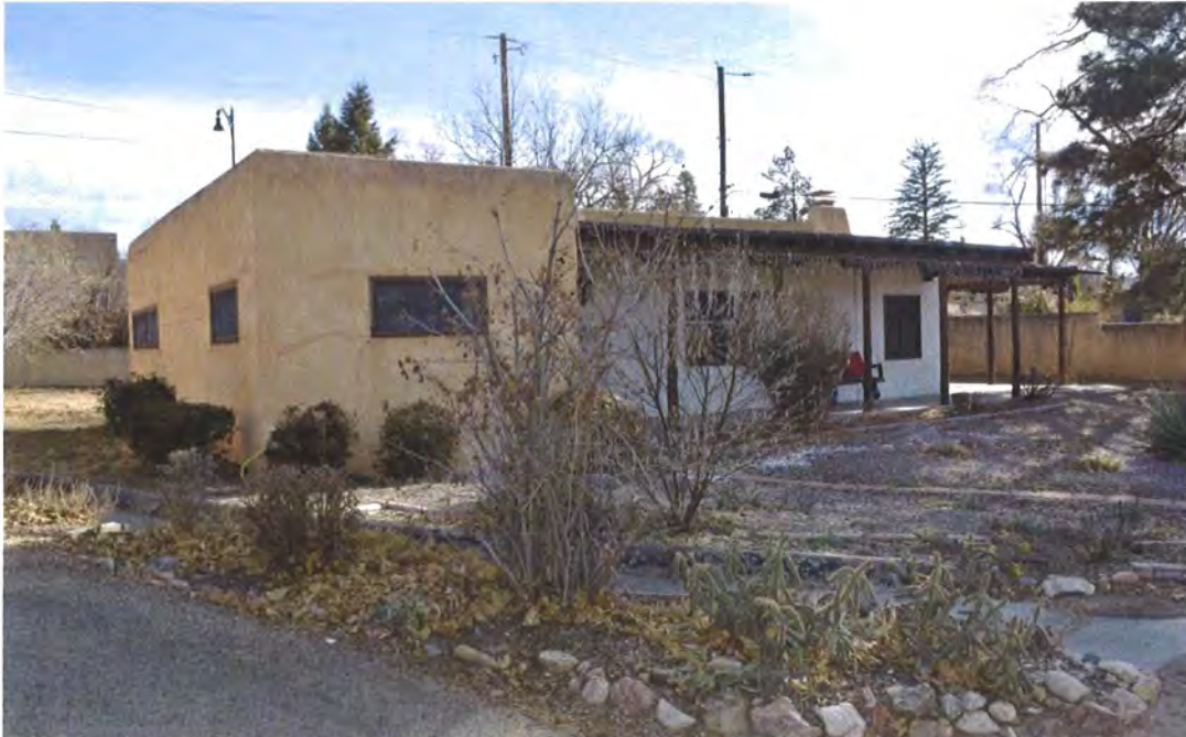
Photo 2: Street and north elevations, facing southeast.
