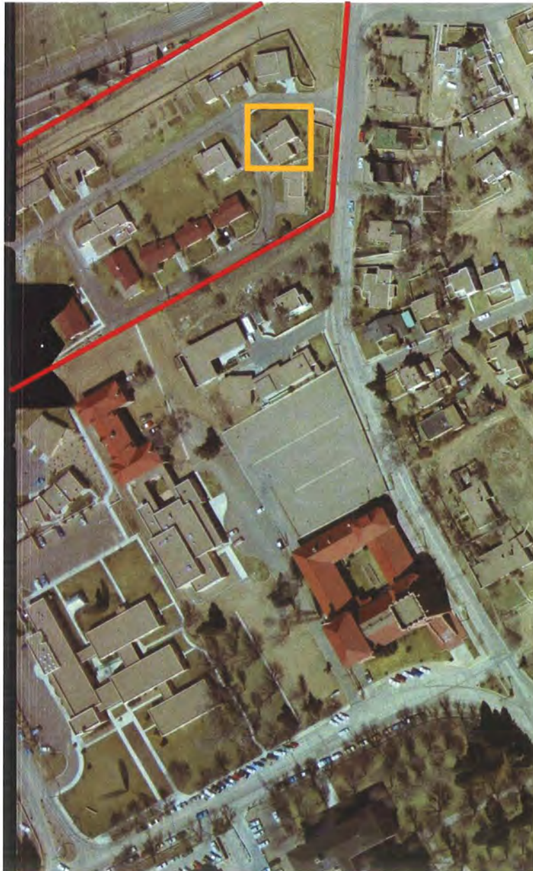
Figure 2: February 27, 1969 aerial photograph Building present, pre-addition. Courtesy NMDOT.
