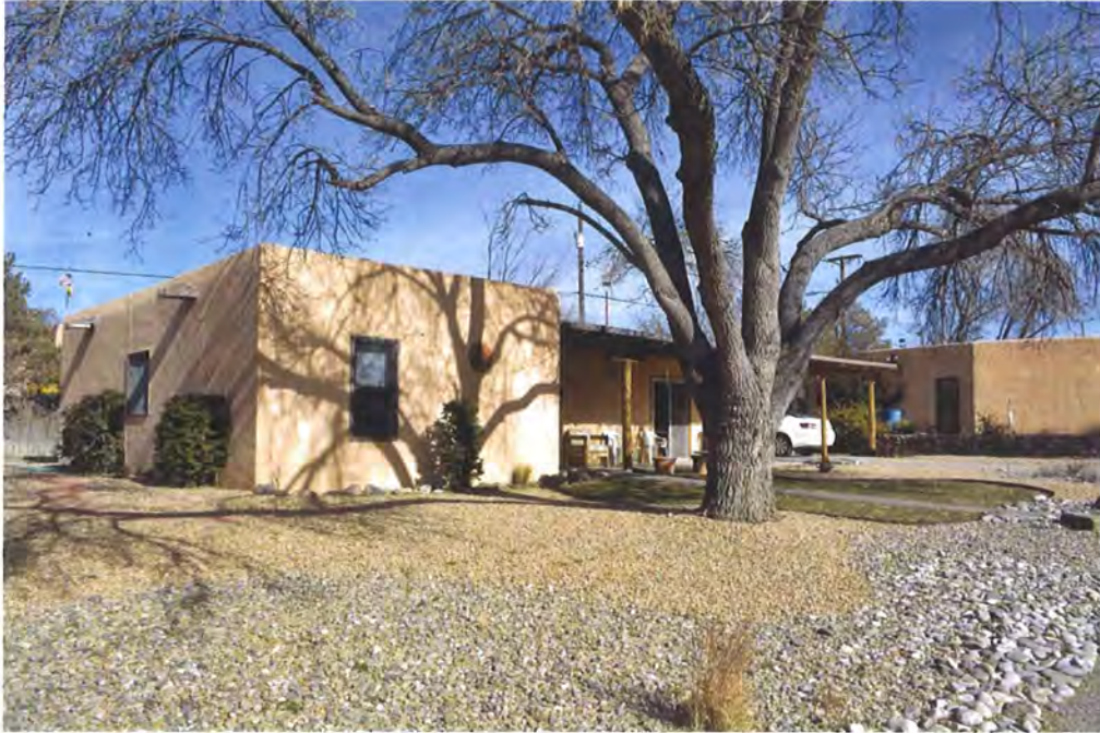
Photo 2: Street and west elevations, facing northeast.
