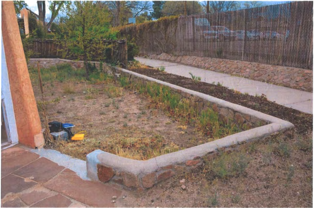
Figure 2: 124 Camino Santiago, rear retaining wall, May 3, 2018.
