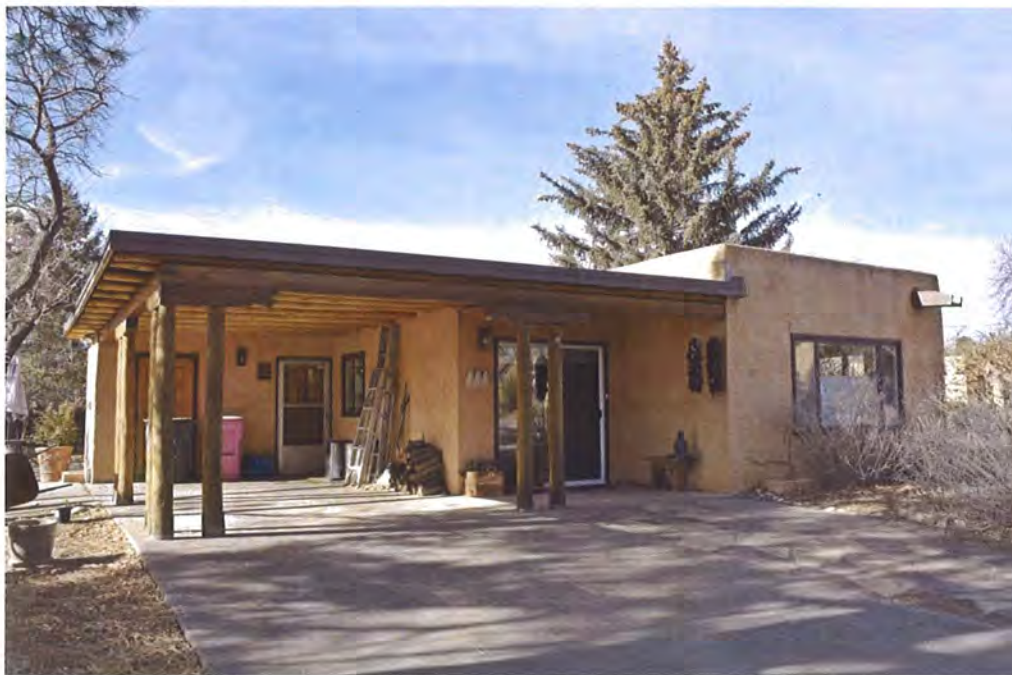
Photo 1: East and south elevations, facing northeast.
