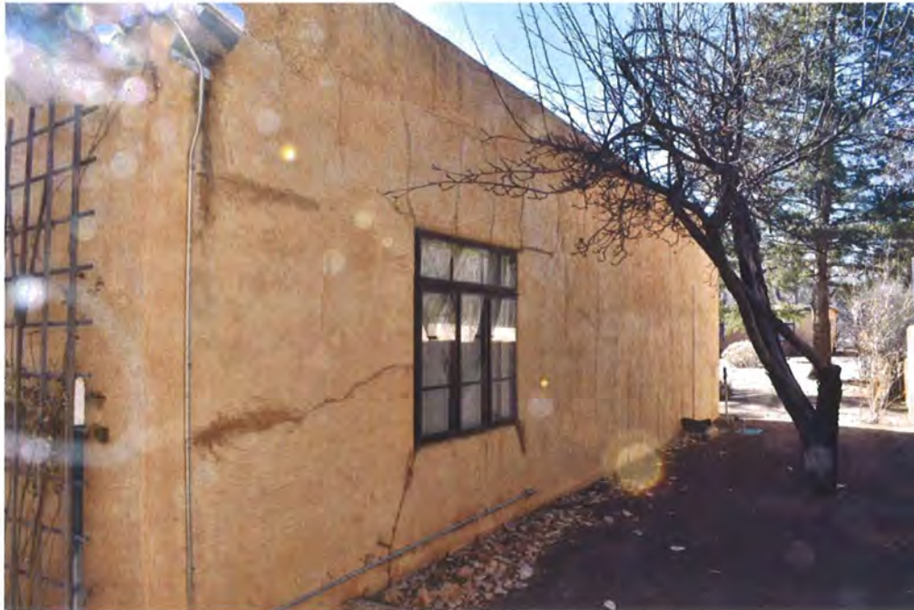
Photo 3: North elevation, facing southwest (Sharon Joyce, February 23, 2018).
