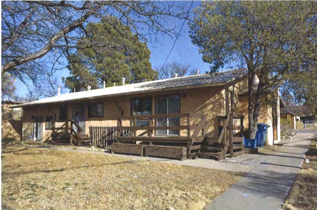
Photo 3: West elevation, facing northeast.
