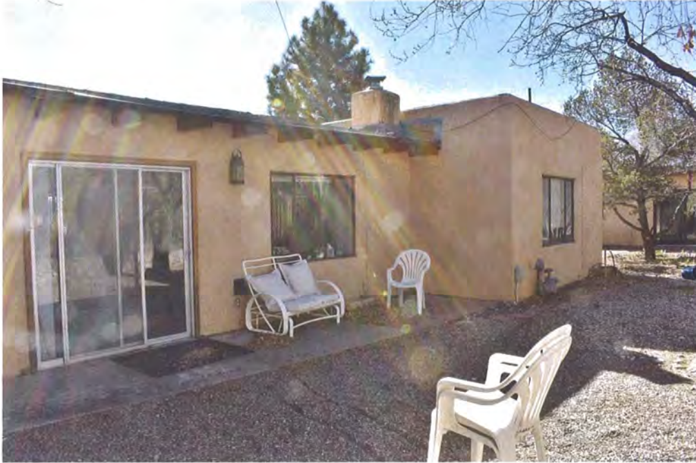
Photo 3: North elevation, facing southwest (Sharon Joyce, February 23, 2018).
