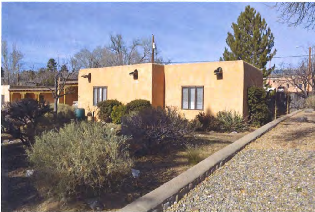
Photo 1: Street and east elevations, facing northwest.
