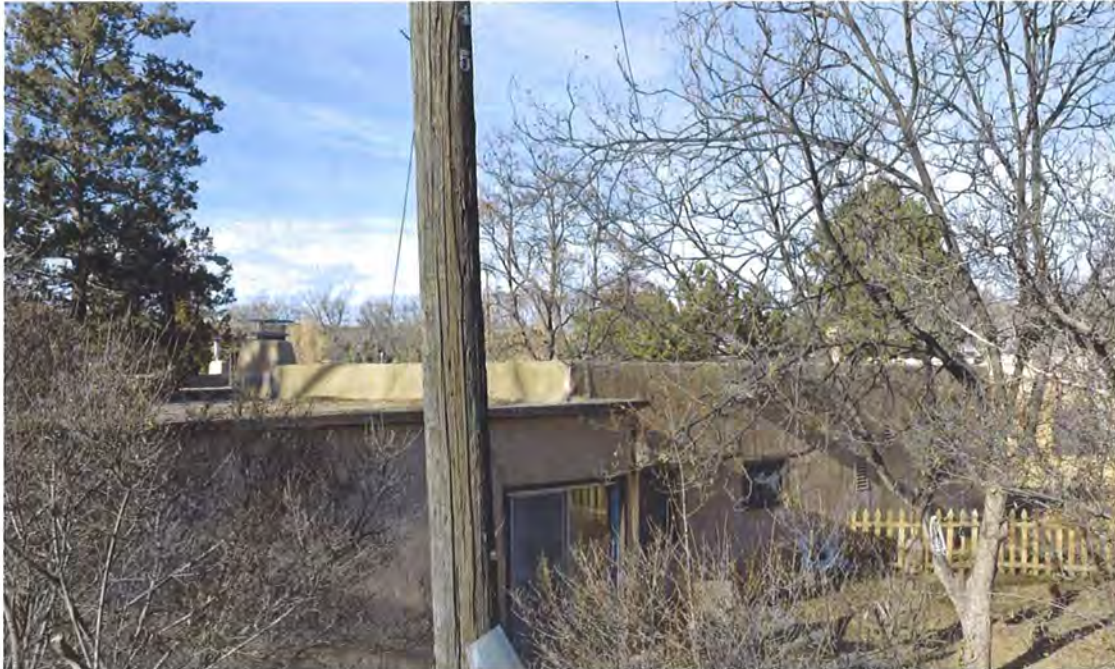
Photo 3: East elevation, facing northwest.
