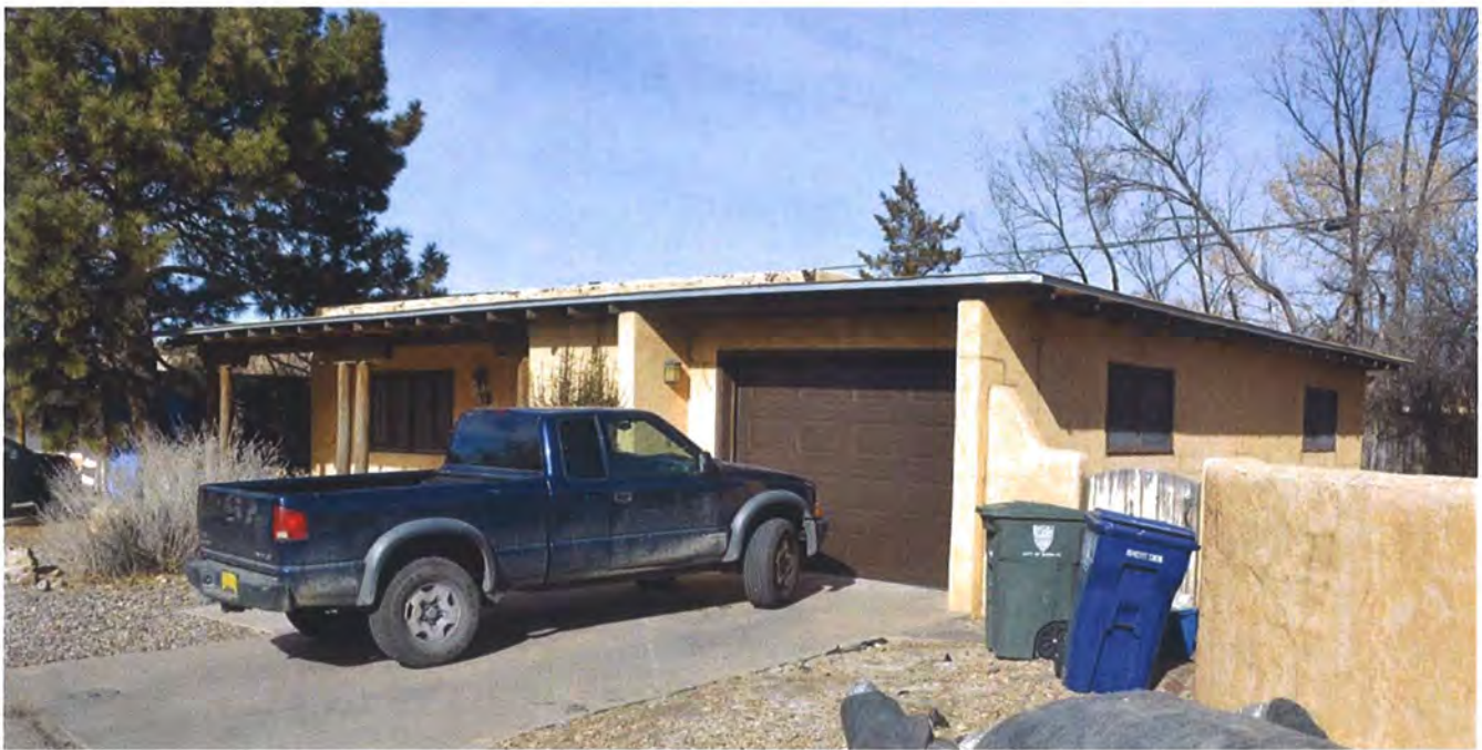
Photo 1: Street elevation and north elevations, facing northwest.
