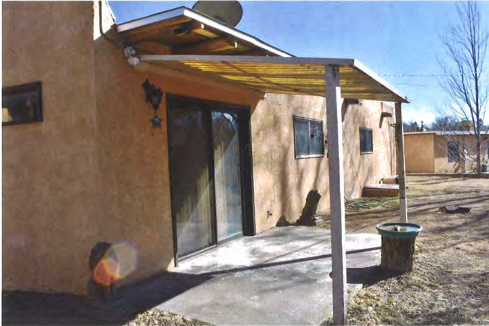
Photo 2: West elevation, facing south (Sharon Joyce, February 23, 2018).
