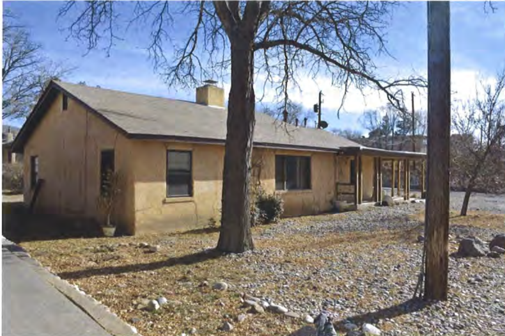
Photo 2: North and west elevations, facing southeast.
