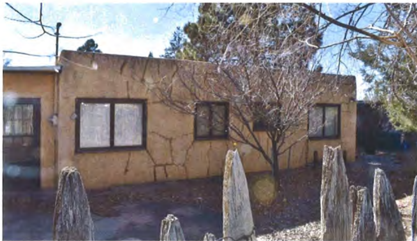
Photo 3: North elevation, facing south and southwest (Sharon Joyce, February 23, 2018).
