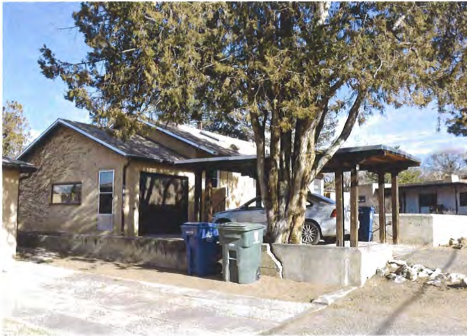
Photo 1: west elevation, facing northeast.
