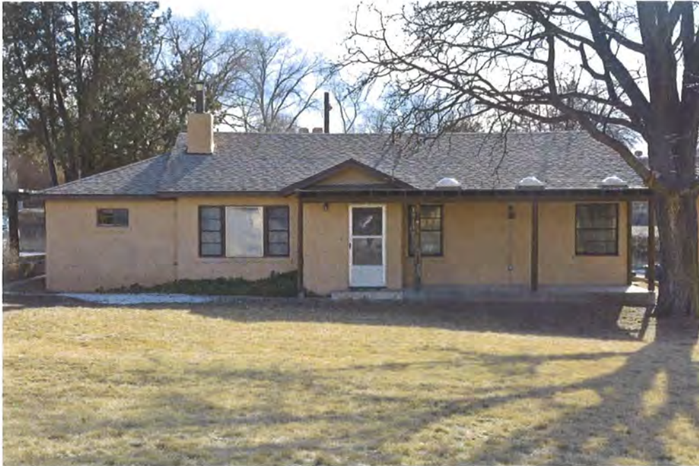
Photo 2: North elevation, facing south.
