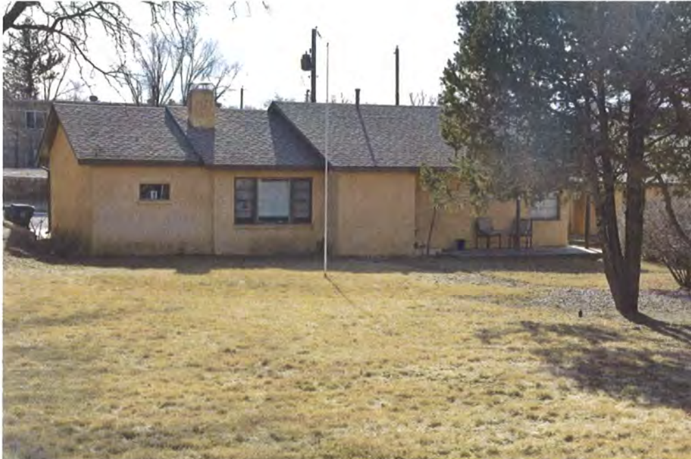
Photo 3: North elevation, facing southwest.
