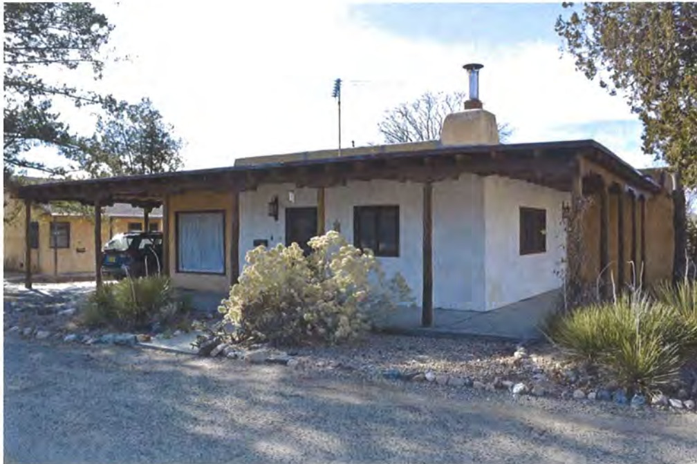
Photo 3: Street and west elevations, facing southeast.
