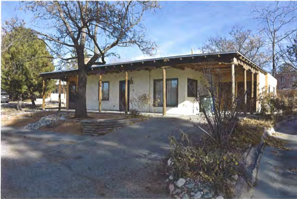
Photo 1: Street elevation and south elevations, facing northeast.
