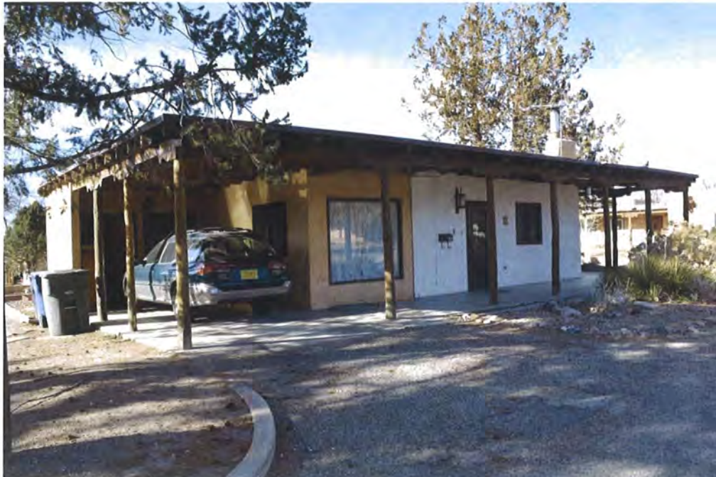
Photo 2: South and east elevations, facing northwest.
