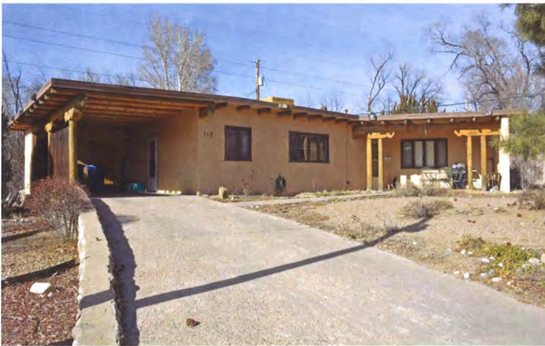
Photo 1: Street, west and south elevations, facing northeast.
