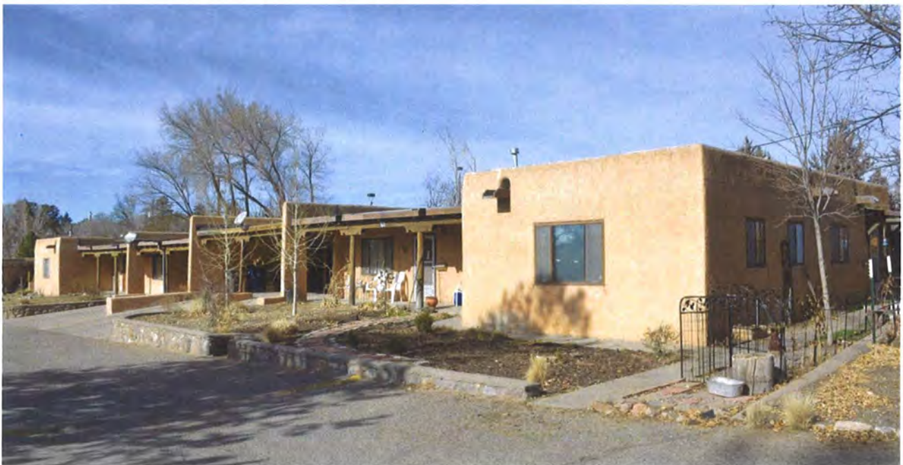
Photo 1: Street elevation and east elevations, facing northwest.
