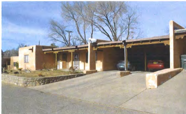
Photo 3: East Unit (top), facing northeast; West Unit (bottom), facing northwest.
