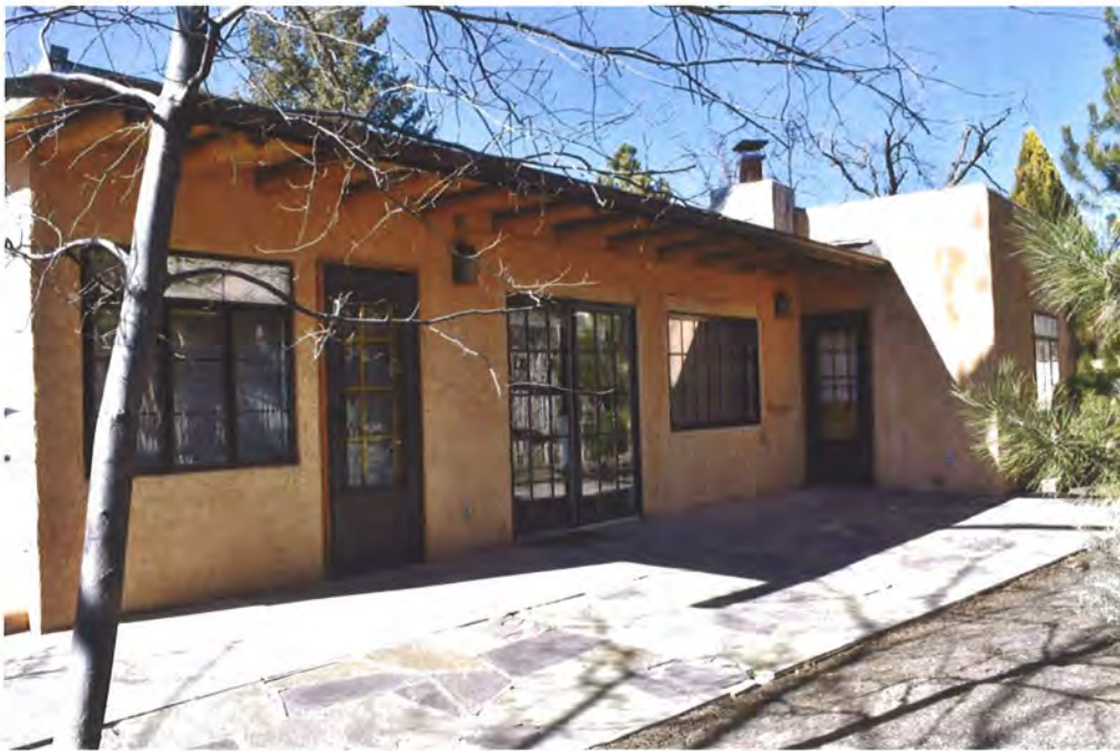
Photo 1: East elevation, facing north.
