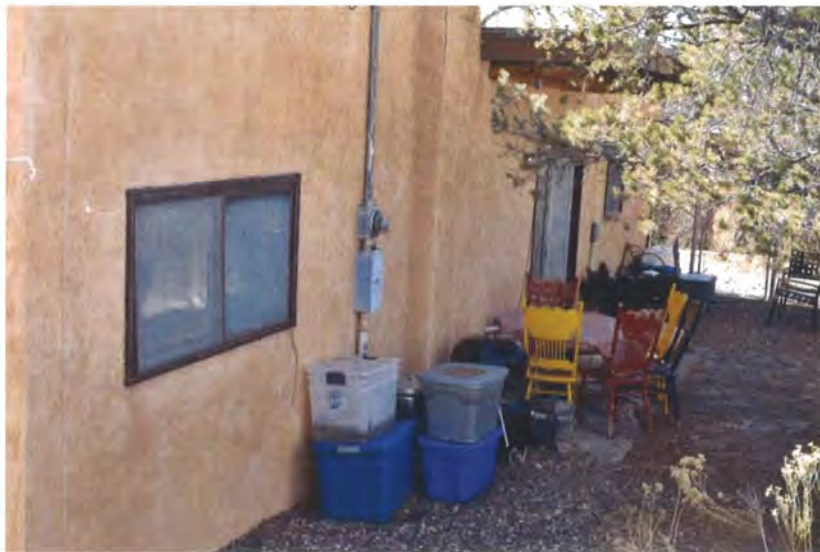
Photo 3: North elevation, facing southeast (top), west (bottom) (Sharon Joyce, February 23, 2018).
