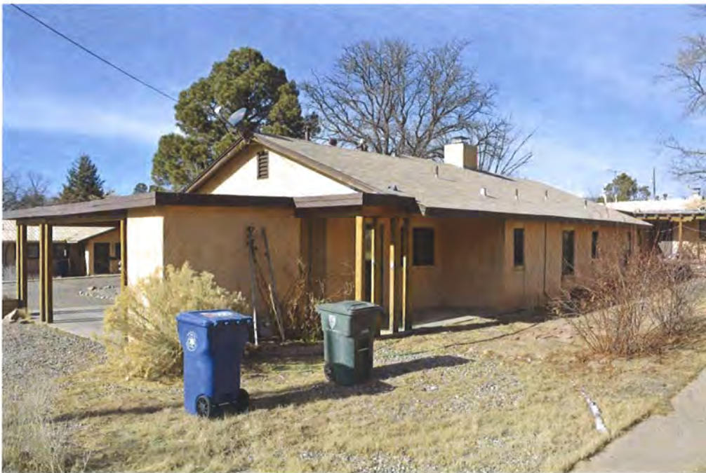
Photo 1: East elevation, facing northwest.
