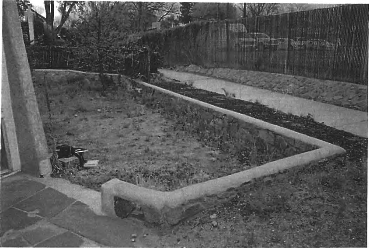
Figure 2: 124 Camino Santiago, rear retaining wall, May 3, 2018.
