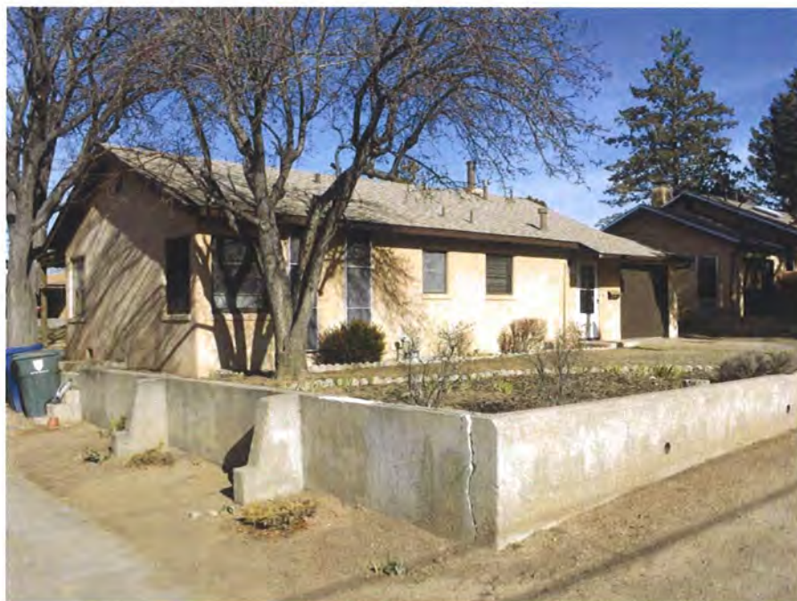
Photo 2: Street west elevations, facing northeast.
