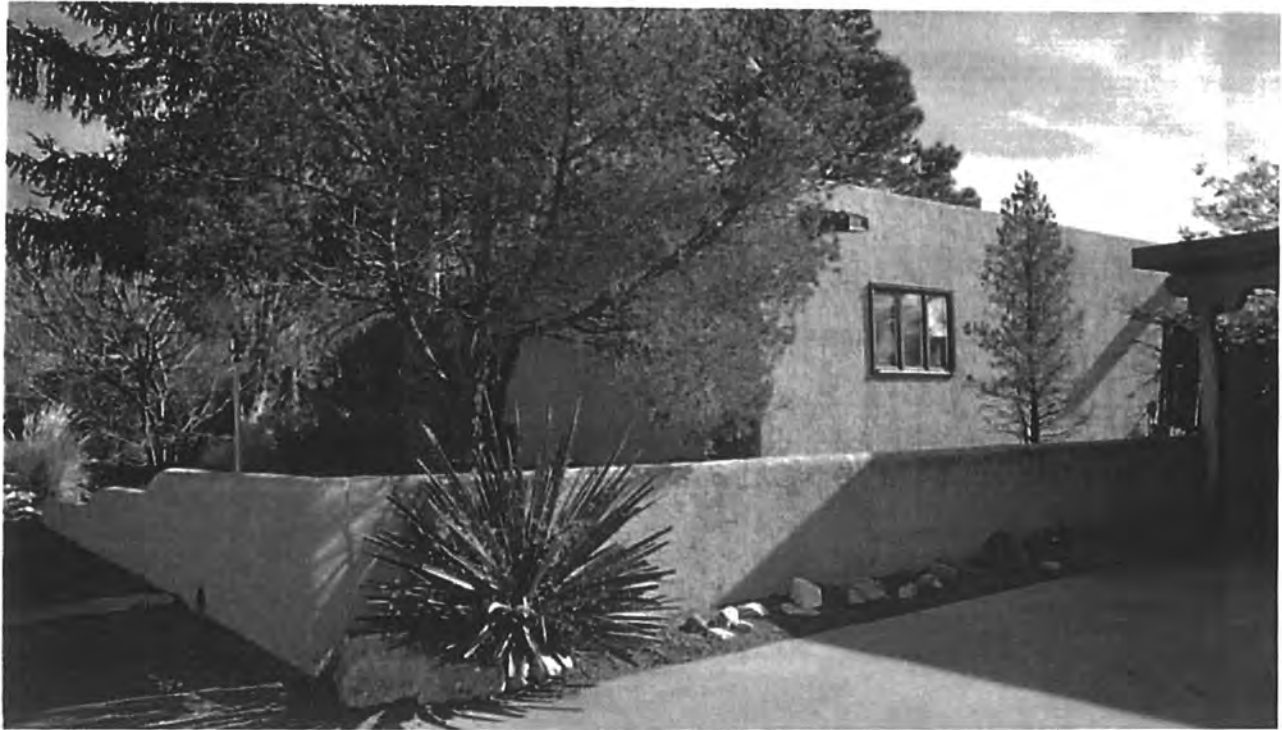
Figure 4: Stucco-on-block property wall between 114 and 118 Camino Santiago, January 18, 2018.
