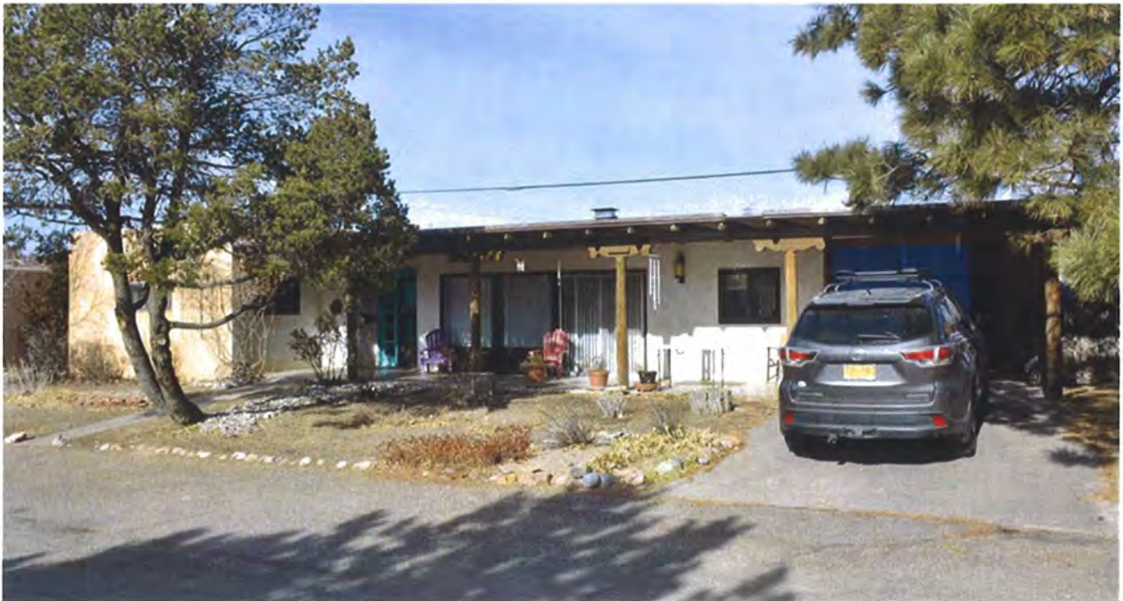
Photo 1: Street and east elevations, facing northwest.
