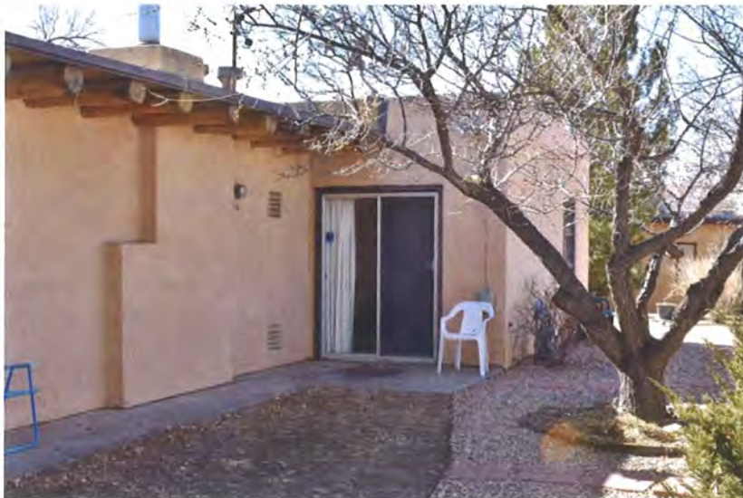
Photo 3: North elevation, facing southwest (Sharon Joyce, February 23, 2018).
