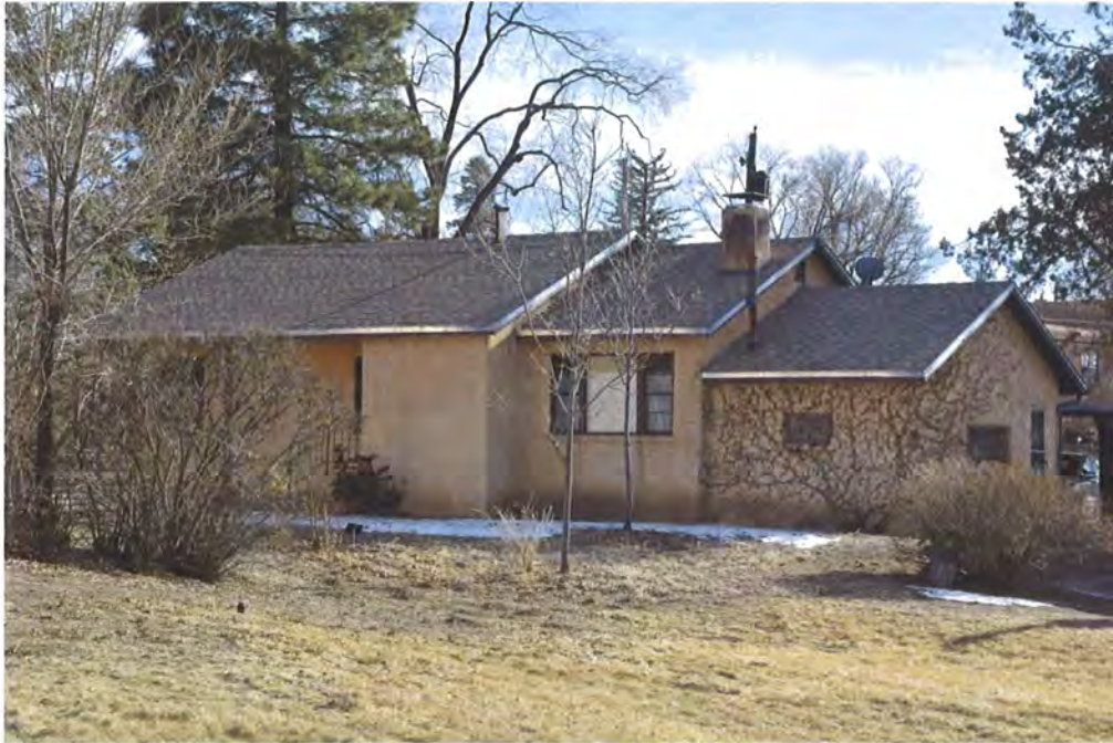
Photo 3: North elevation, facing southeast.
