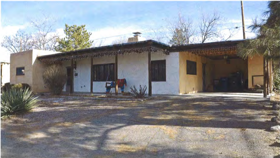
Photo 1: Street and south elevations, facing southeast.
