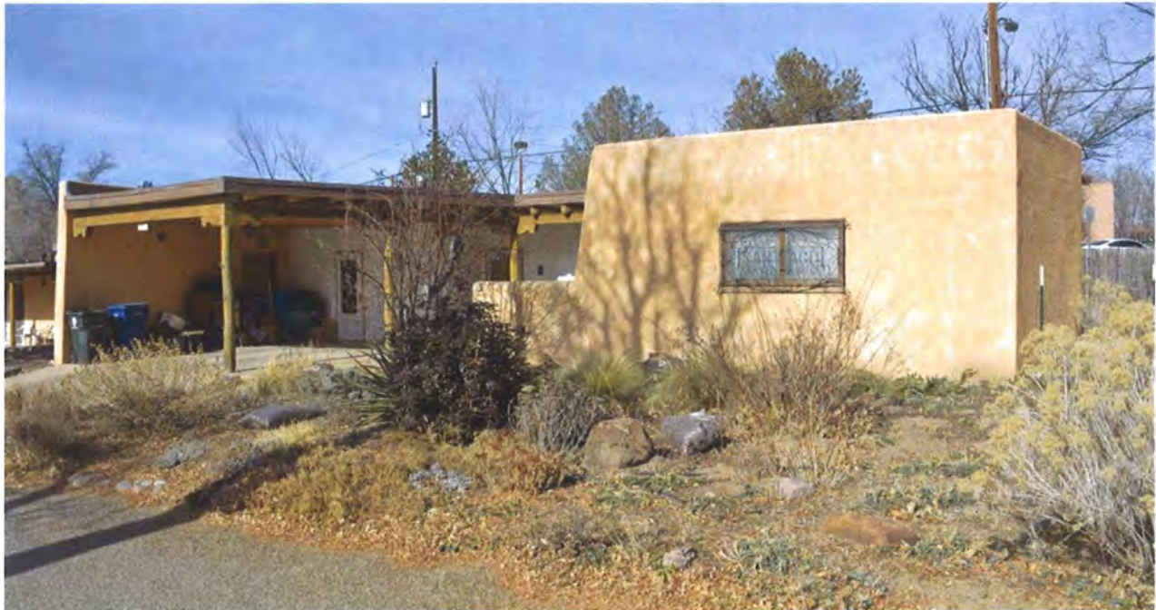
Photo 1: Street and east elevations, facing northwest.
