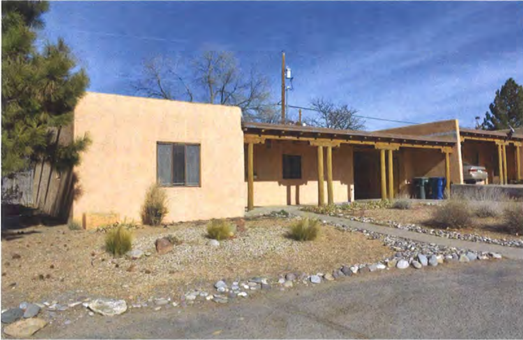
Photo 2: Street and west elevations, facing northeast.
