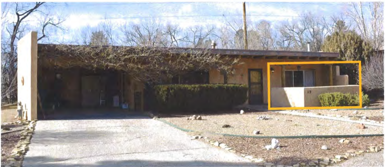
Photo 1: Street and south elevations, facing northwest. Box indicates removed portion of angled patio wall.
