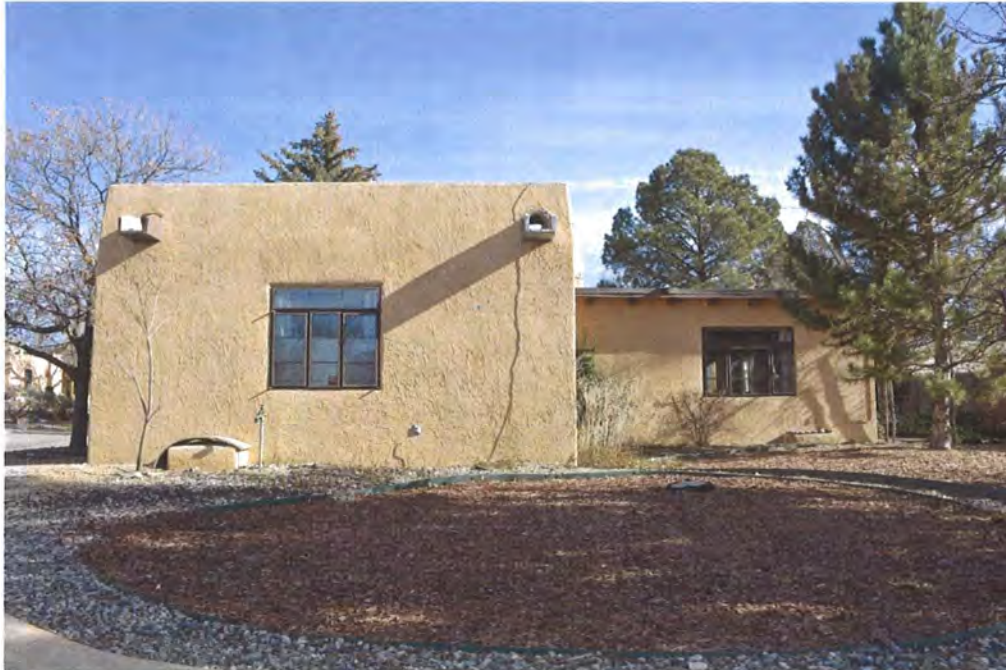
Photo 2: West elevation, facing east.
