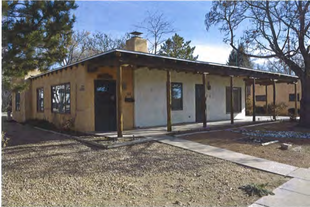
Photo 2: North and street elevations, facing southeast.
