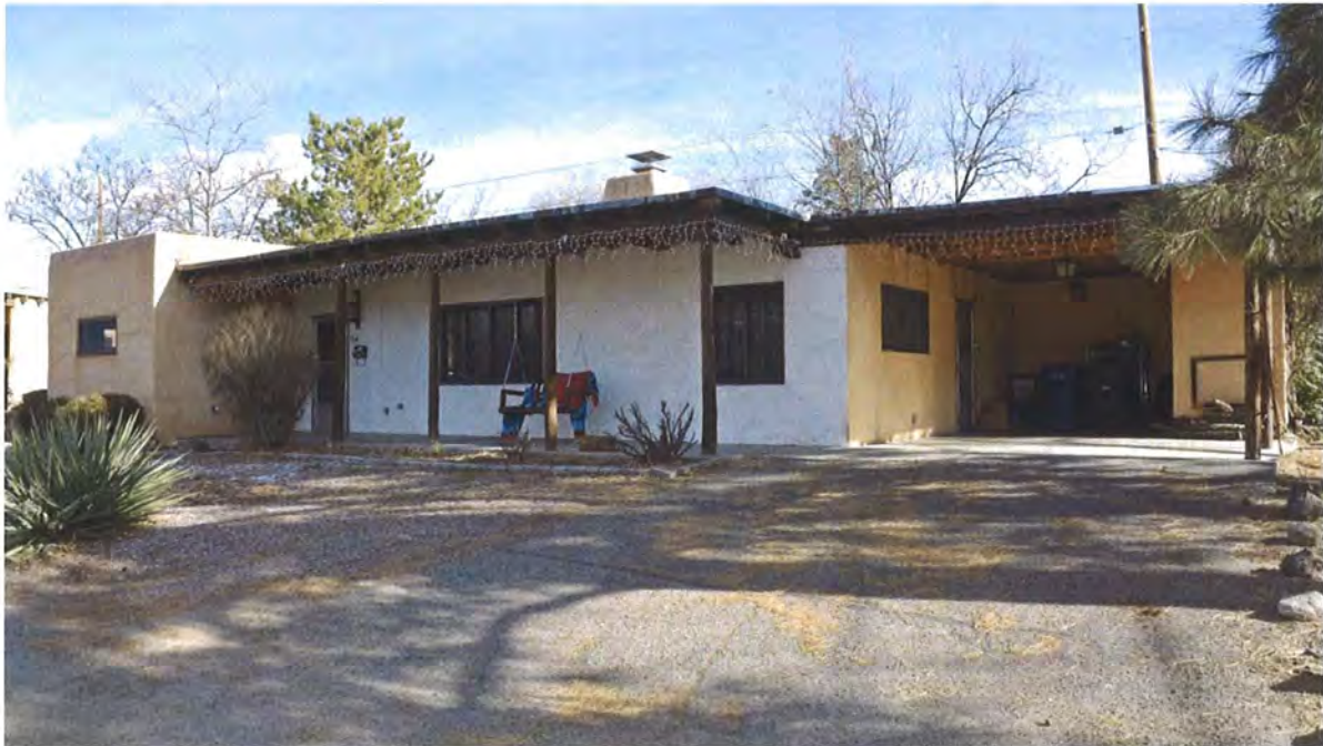
Photo 1: Street and south elevations, facing southeast.
