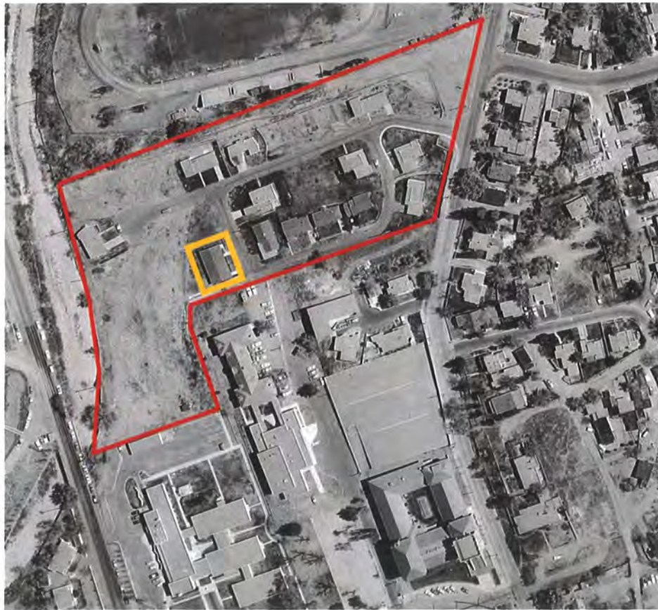
Figure 1: May 2, 1966 aerial photograph. Building present; pre-alteration. Courtesy NMDOT.
