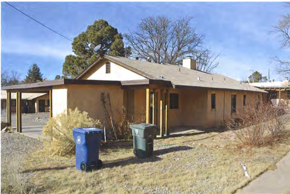
Photo 1: East elevation, facing northwest.
