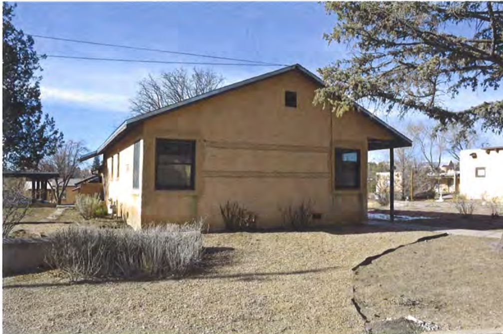
Photo 2: East elevation, facing northwest.
