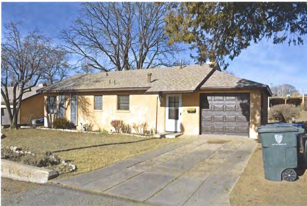
Photo 2: Street and east elevations, facing northeast.
