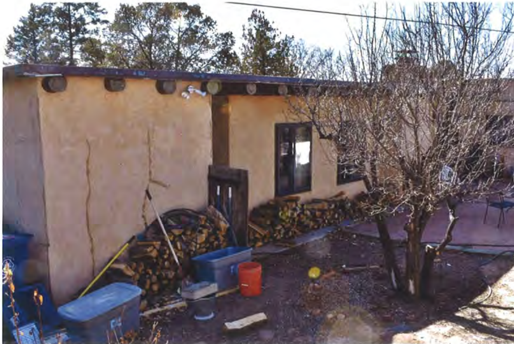
Photo 3: North elevation, facing southwest (Sharon Joyce, February 23, 2018).
