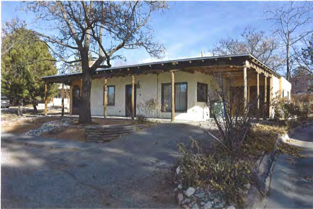
Photo 1: Street elevation and south elevations, facing northeast.
