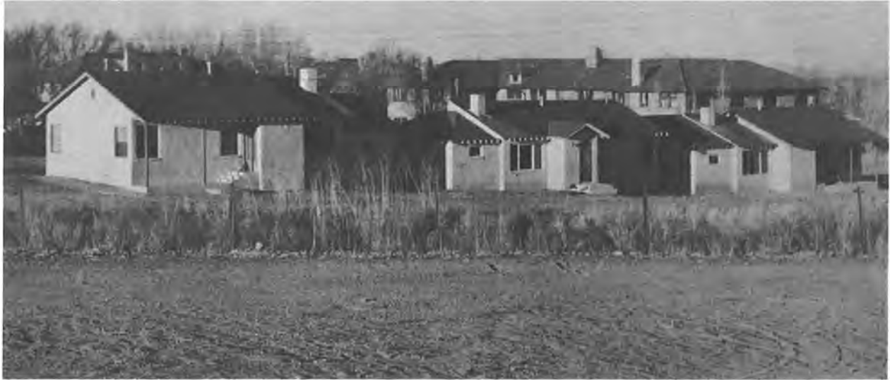
Figure 4: Rear (north) elevation of married faculty cottages, c. 1950s. Source: Atkins, 1983.
