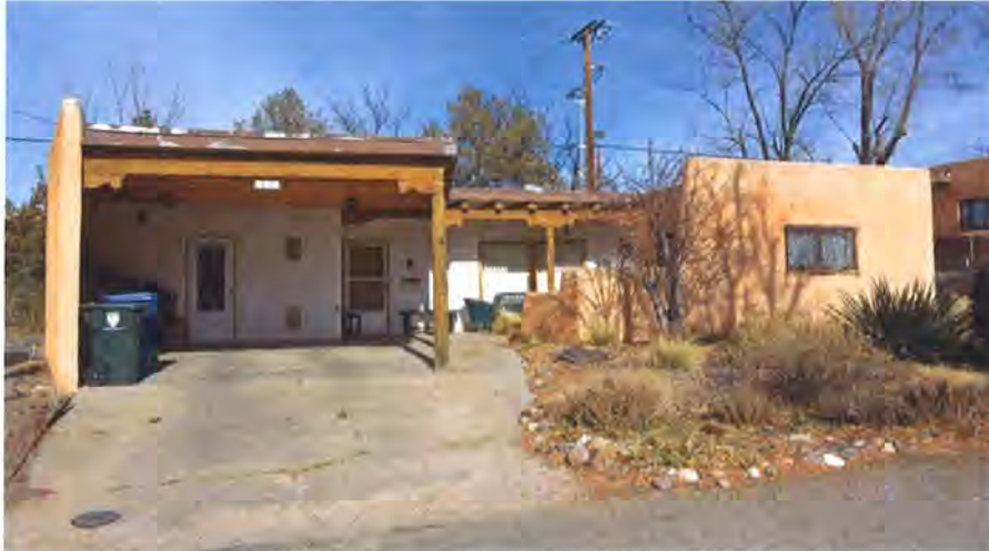
Figure 10: Example of carport dominated front façade, 109 Camino Santiago.
