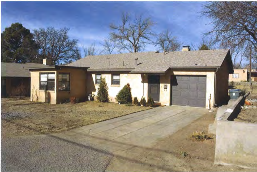
Photo 1: Street and east elevations, facing northwest.
