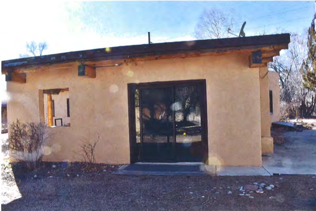
Photo 3: North elevation, facing south (Sharon Joyce, February 23, 2018).
