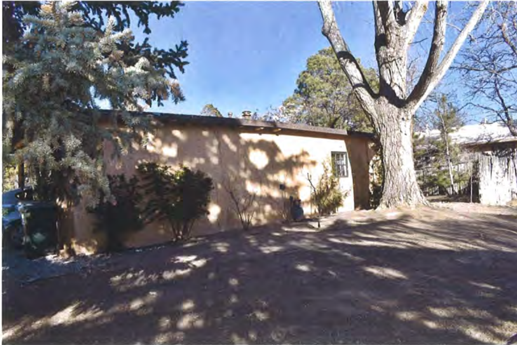
Photo 2: South elevation, facing northeast (Sharon Joyce, February 23, 2018).
