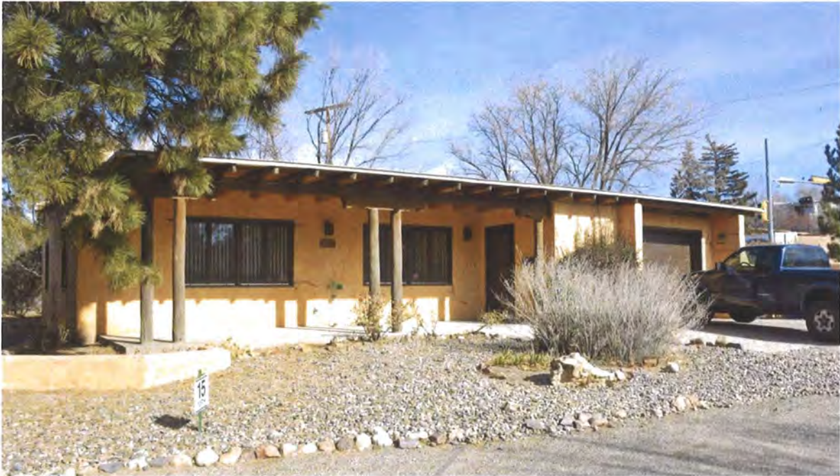
Photo 2: Street and west elevations, facing northeast.
