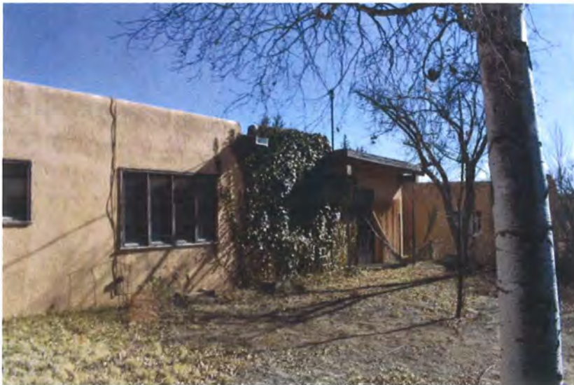
Photo 2: West elevation, facing southwest (Sharon Joyce, February 23, 2018).
