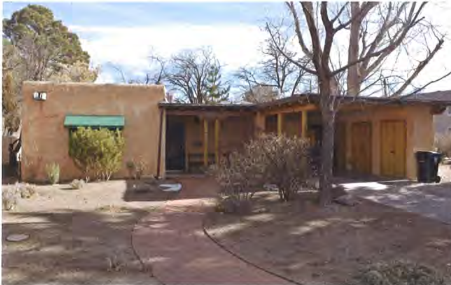
Figure 12: 120 Camino Santiago, constructed in c. 1971.
