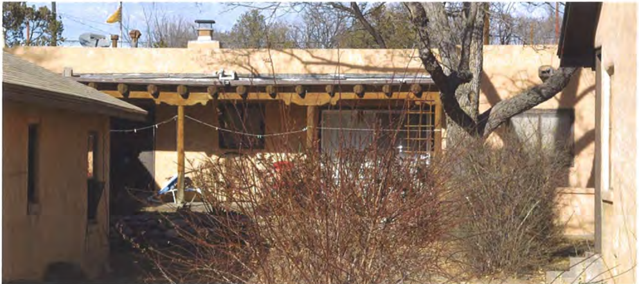
Photo 4: South elevation, facing north.
