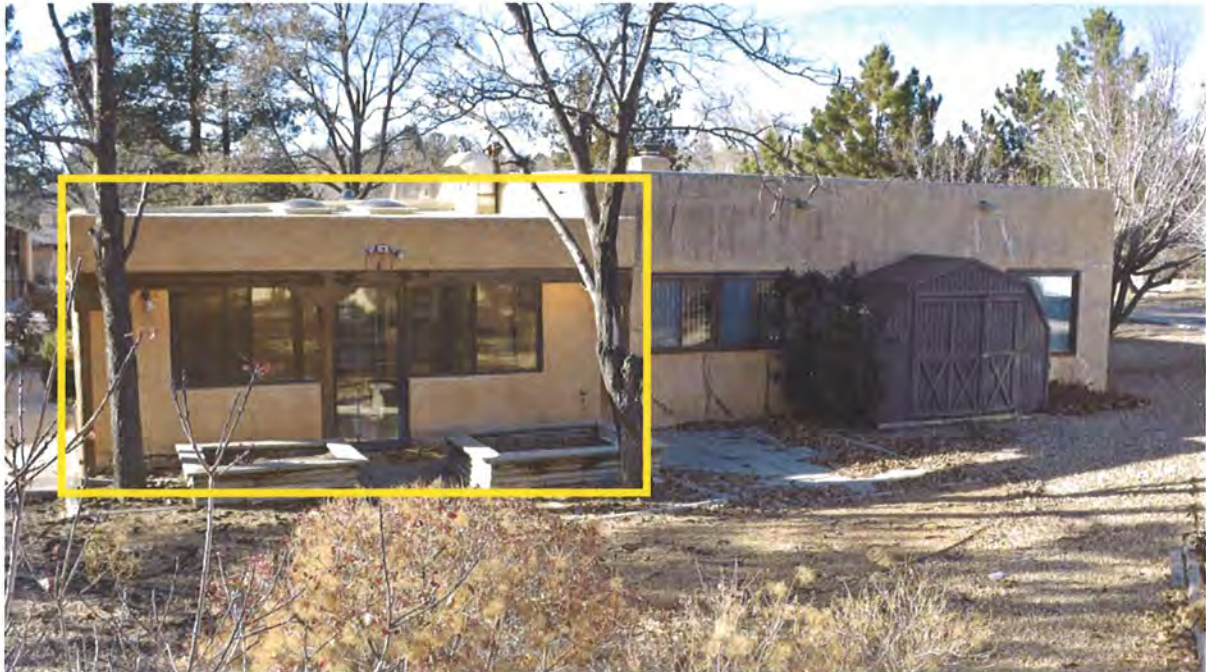
Photo 3: East elevation, facing northwest. Non-historic addition on left.
