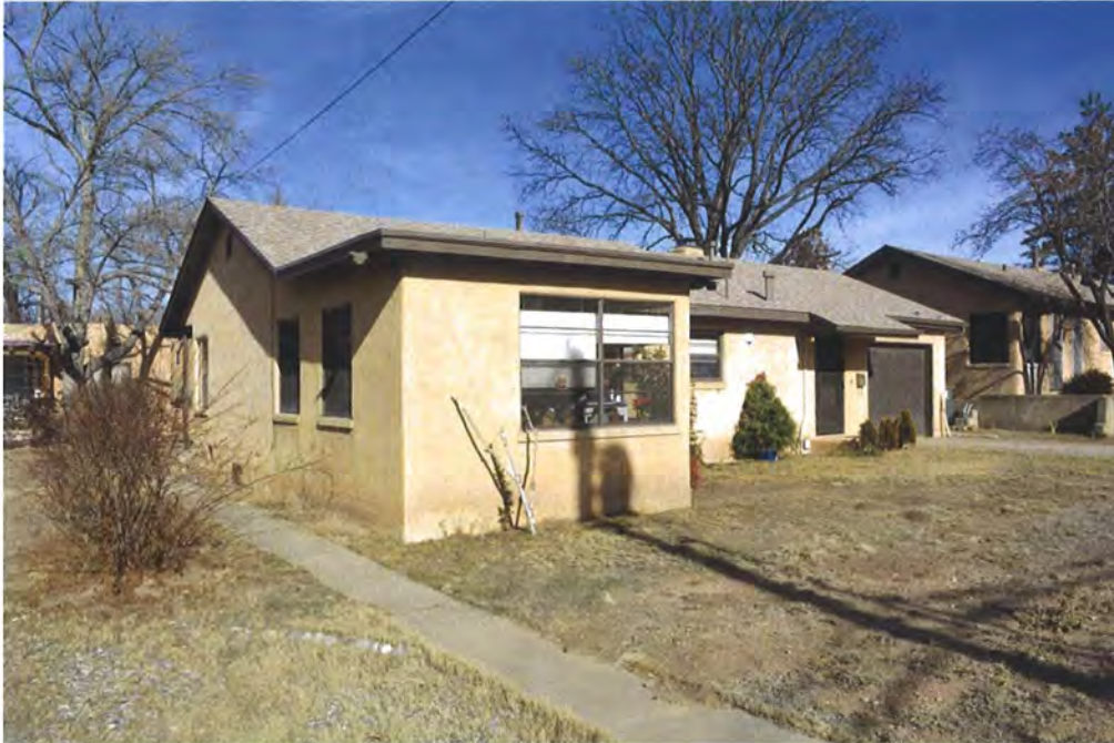
Photo 2: Street and west elevations, facing northeast.
