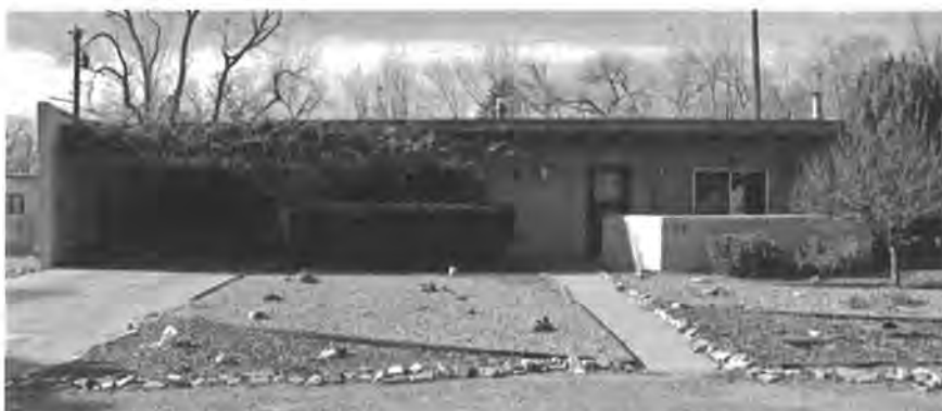
Figure 8: 119 Camino Santiago, an example of a Contemporary flat-roof form.
