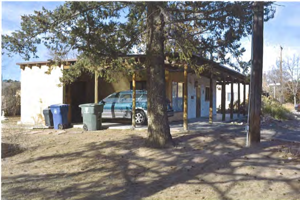
Photo 1: South and east elevations, facing northwest.
