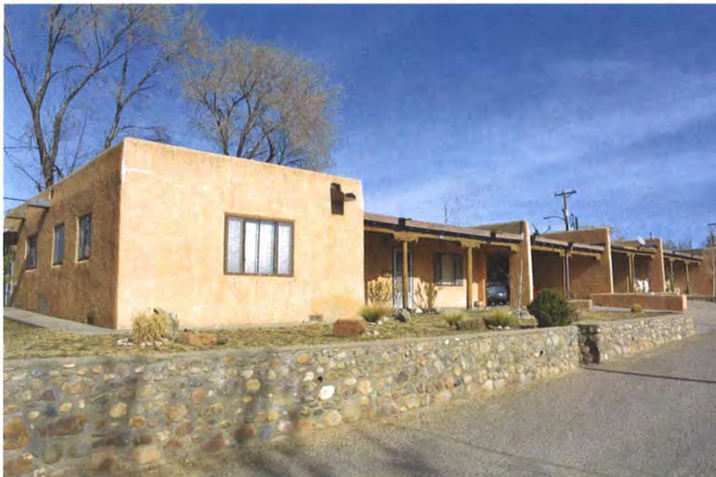
Photo 2: Street and west elevations, facing northeast.
