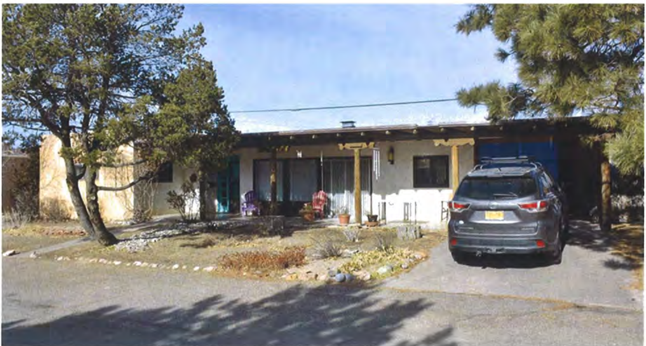
Photo 1: Street and east elevations, facing northwest.
