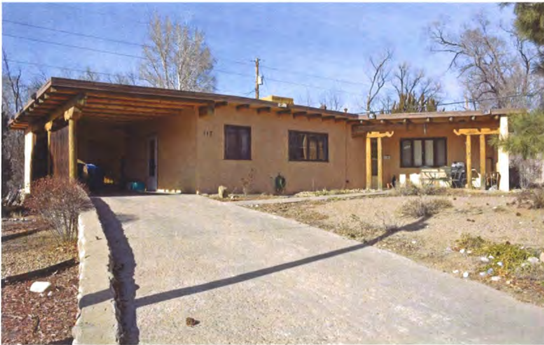
Photo 1: Street, west and south elevations, facing northeast.
