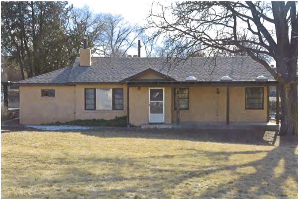
Photo 2: North elevation, facing south.
