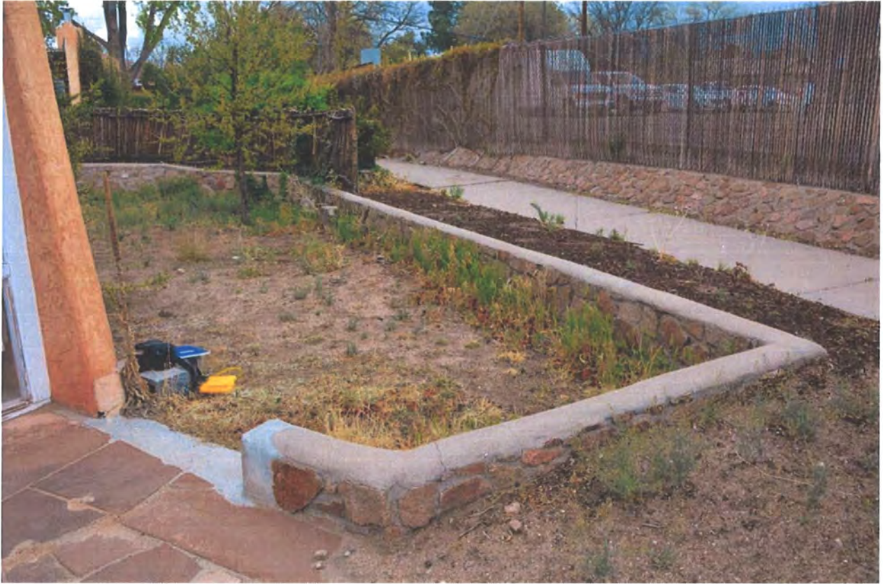
Figure 2: 124 Camino Santiago, rear retaining wall, May 3, 2018.
