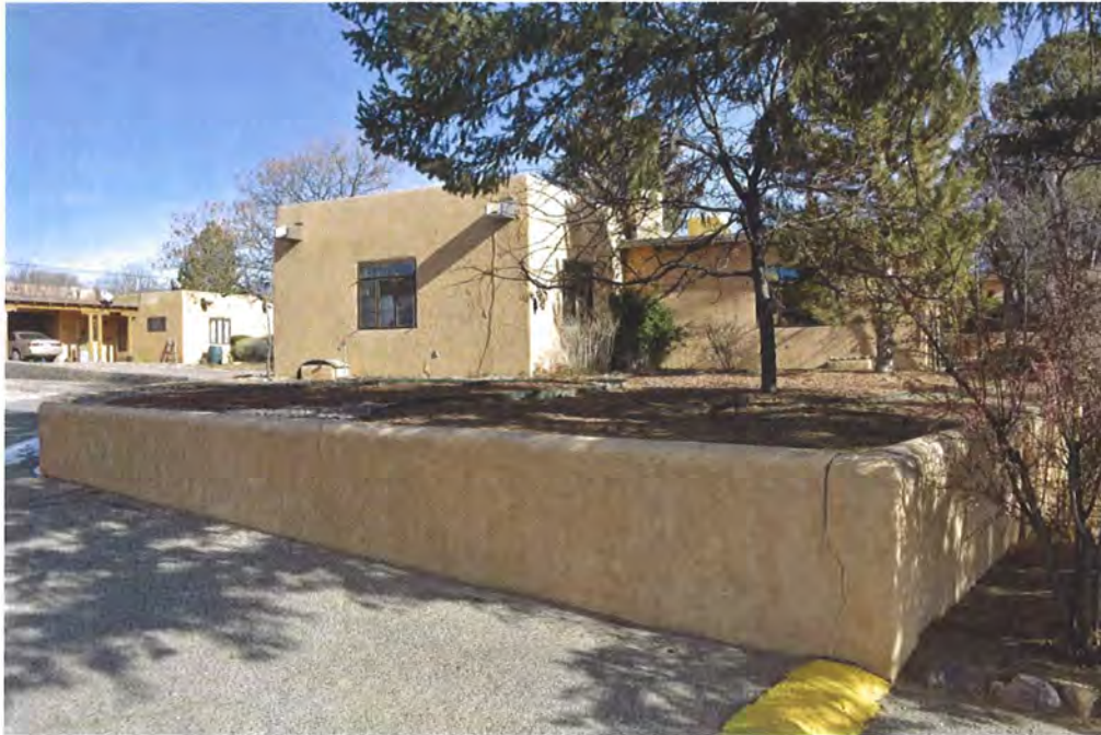
Photo 3: West and south elevations, facing northeast.
