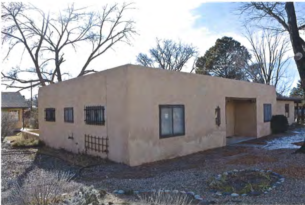
Photo 1: Street and north elevations, facing southeast.
