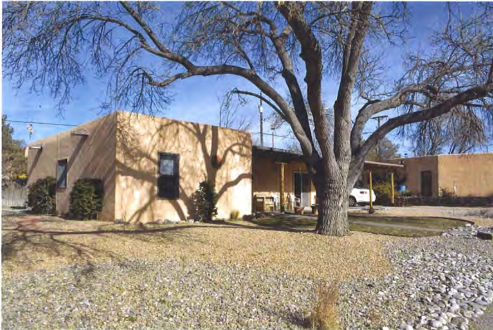
Photo 2: Street and west elevations, facing northeast.
