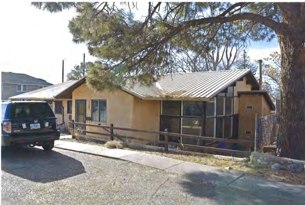
Photo 1: Street and north elevations, facing southwest.
