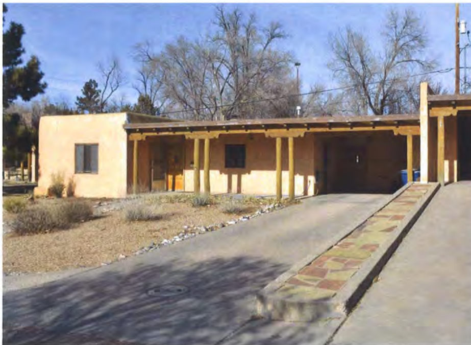
Photo 1: Street and east elevations, facing northwest.
