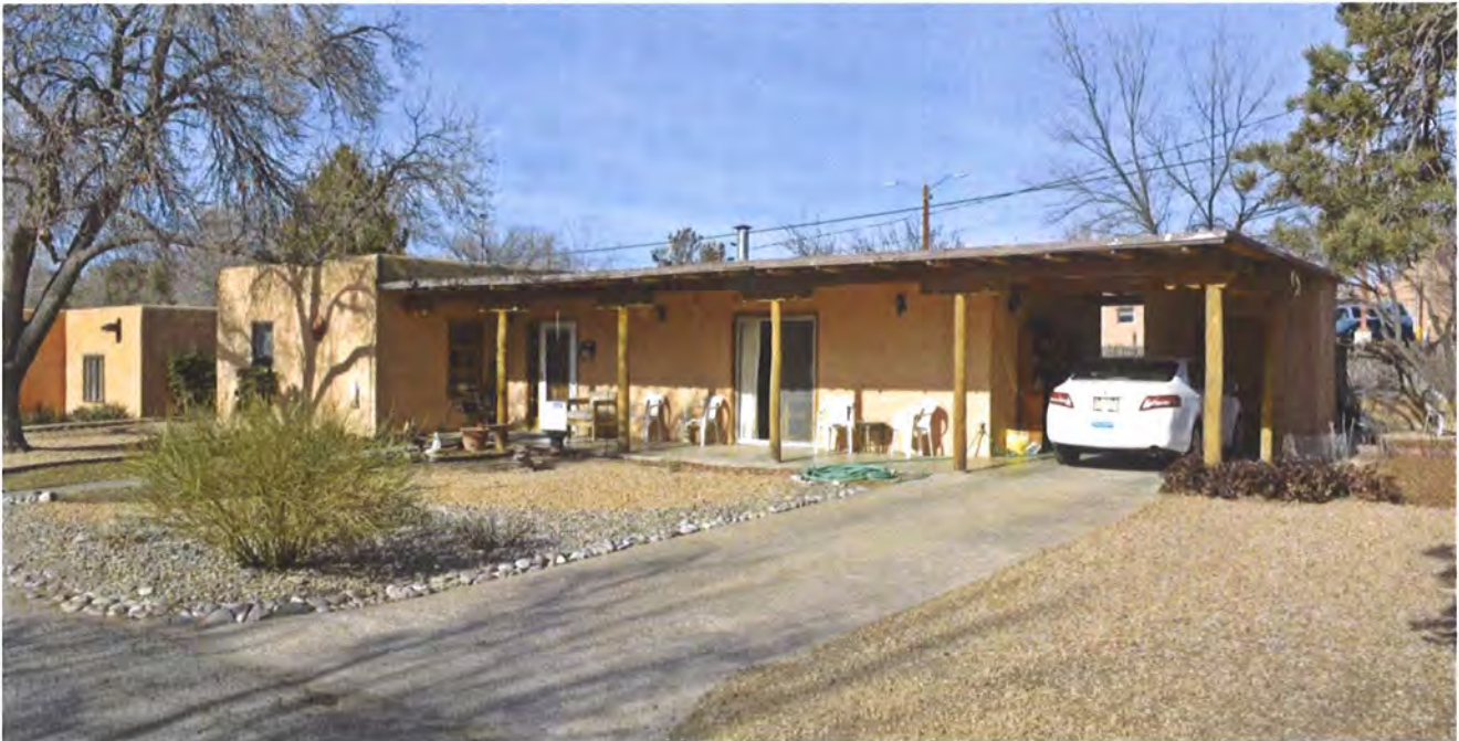
Photo 1: Street and east elevations, facing northwest.
