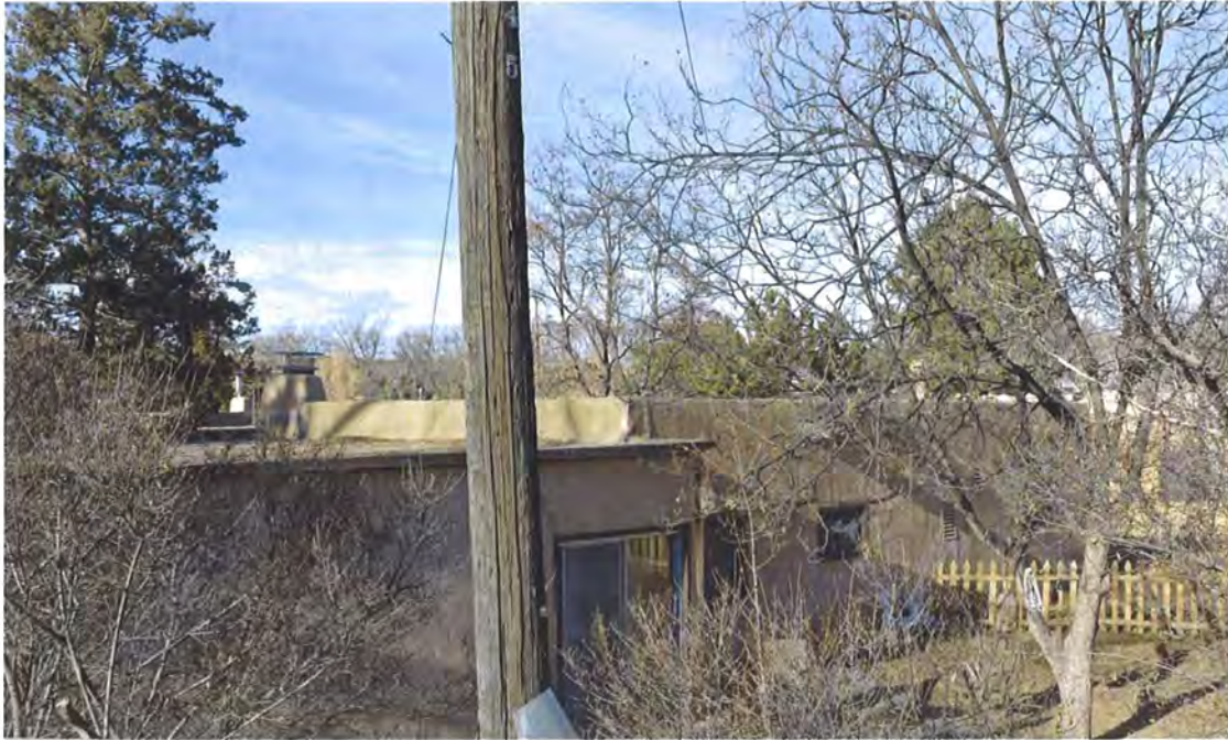
Photo 3: East elevation, facing northwest.
