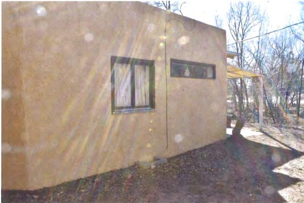
Photo 3: North elevation, facing southwest (Sharon Joyce, February 23, 2018).
