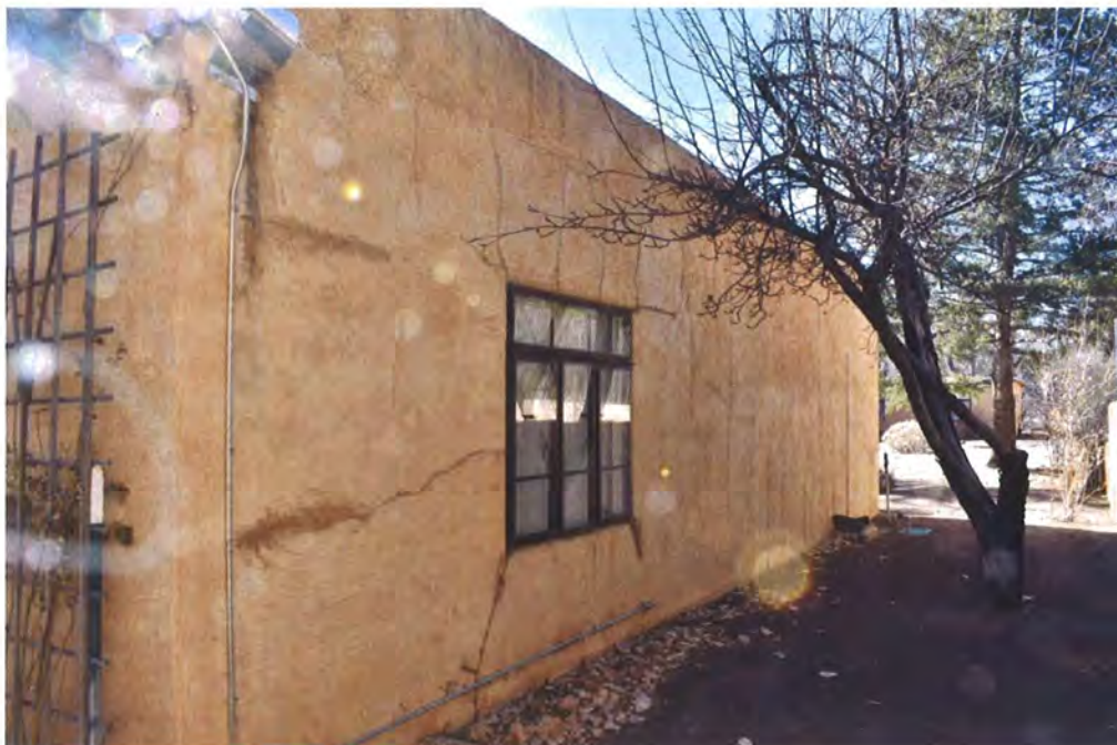
Photo 3: North elevation, facing southwest (Sharon Joyce, February 23, 2018).
