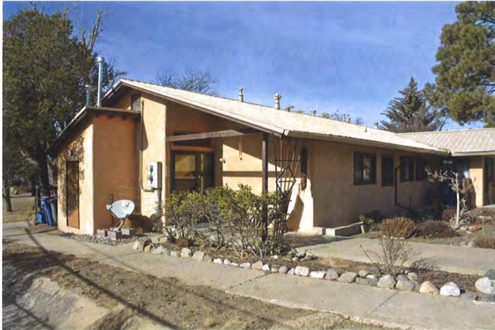
Photo 2: South elevation, facing northwest.
