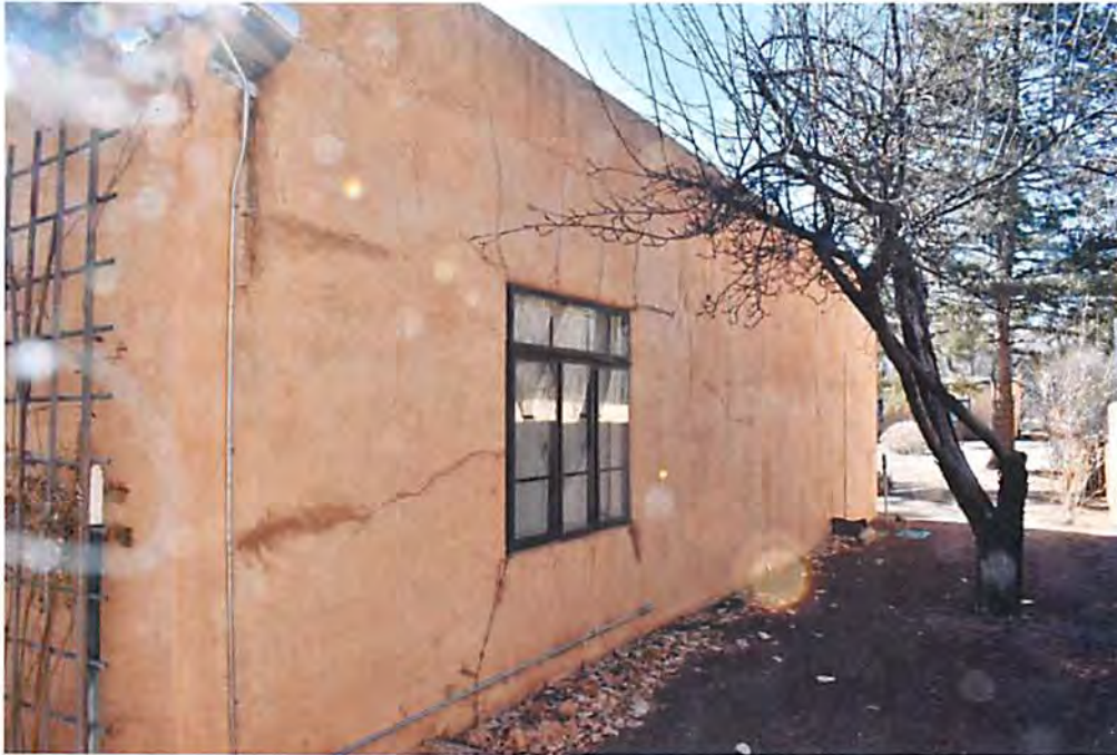
Photo 3: North elevation, facing southwest (Sharon Joyce, February 23, 2018).
