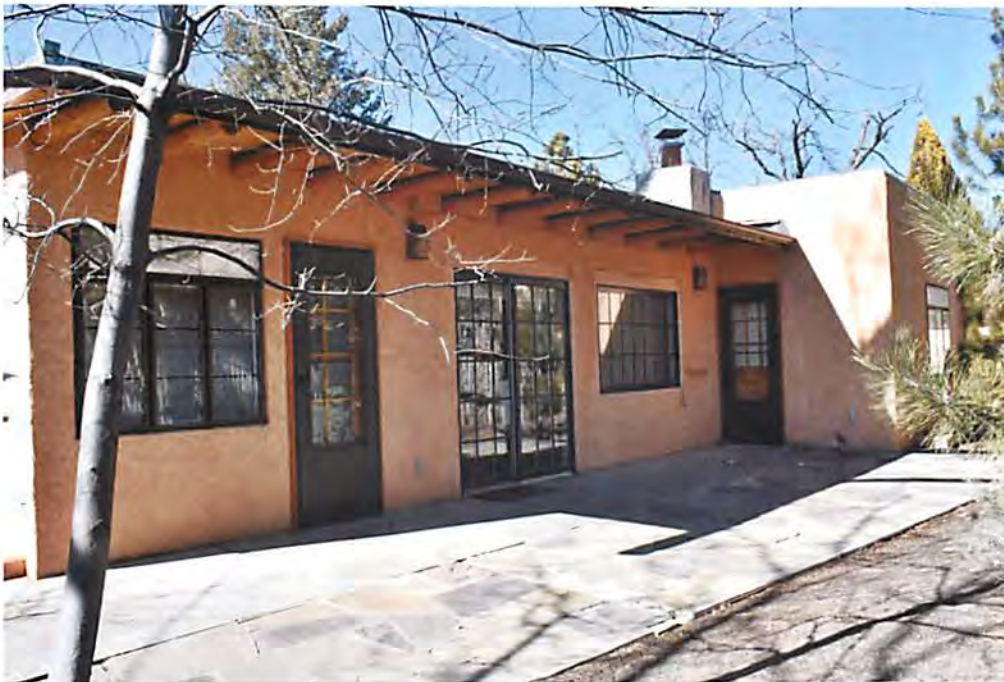
Photo 1: East elevation, facing north.
