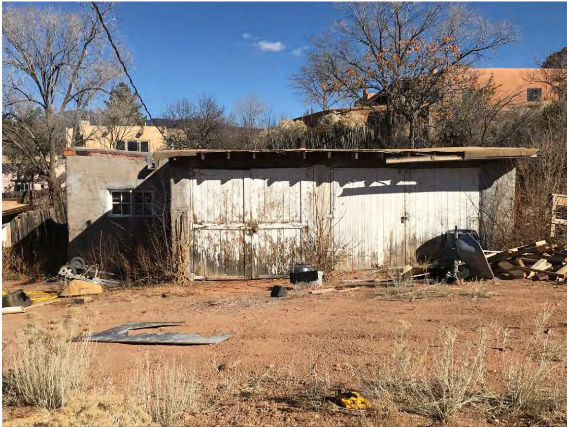
Photo 10: Upper Building, west elevation. Camera facing east.
