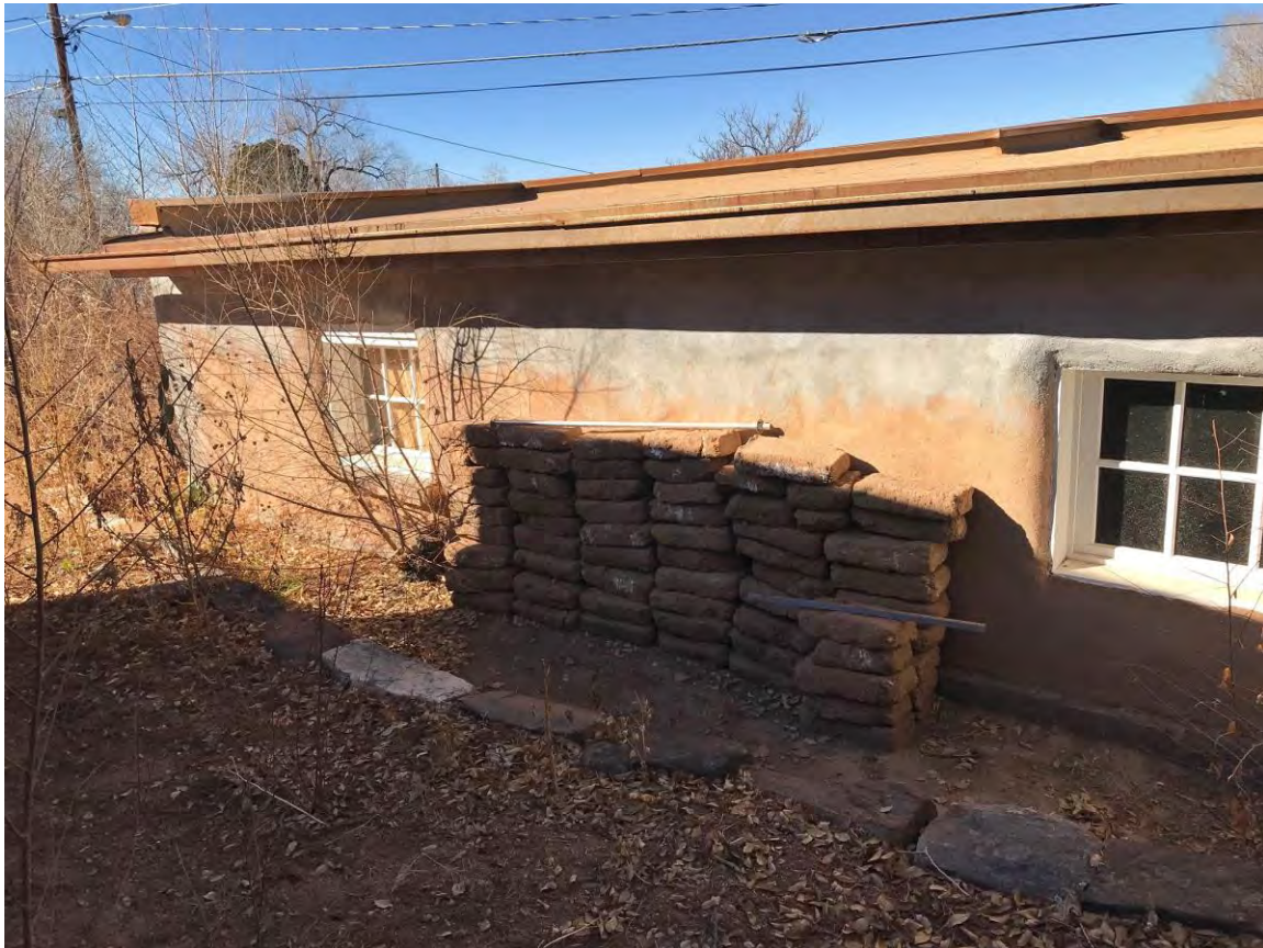
Photo 6: Lower Building, south elevation. Camera facing northwest.
