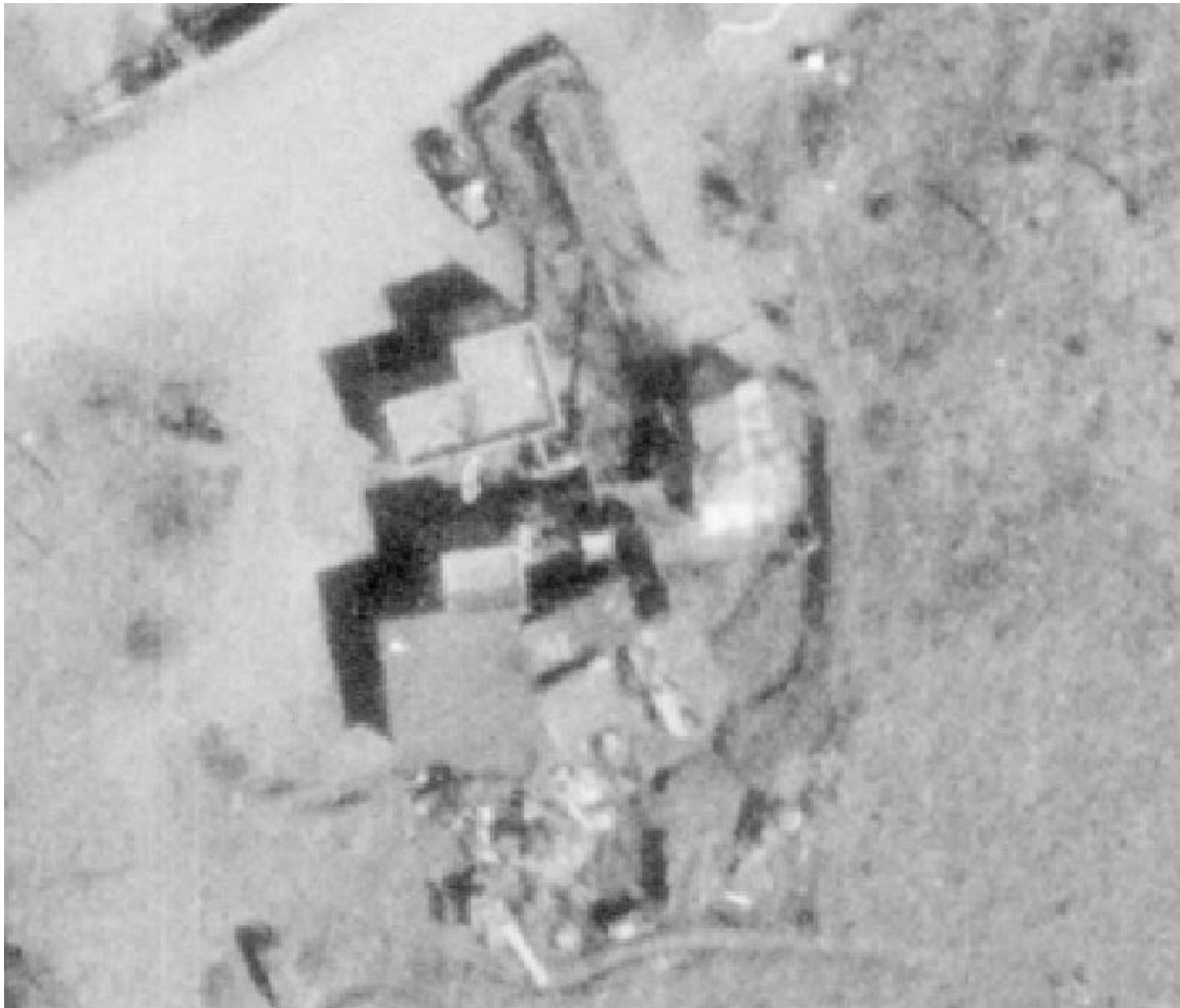
Figure 4: Subject buildings. May 2, 1966, aerial photograph. Courtesy New Mexico Department of Transportation.
