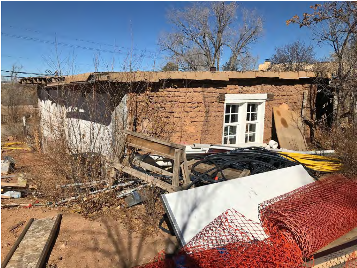
Photo 11: Upper Building, south elevation. Camera facing northeast.
