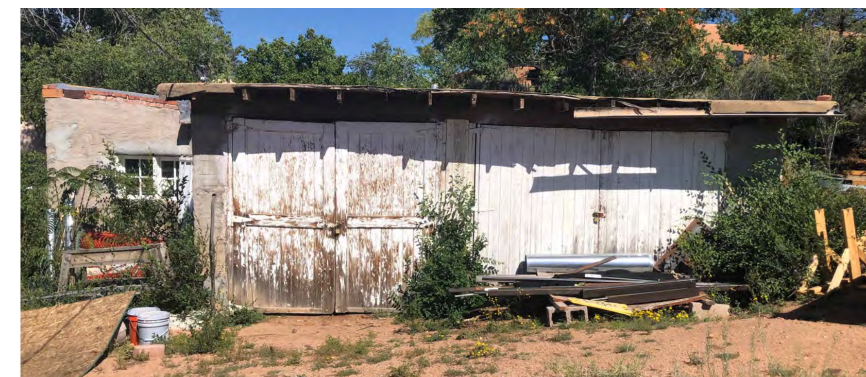
EXISTING REAR BUILDING WEST FACADE PHOTOGRAPH
