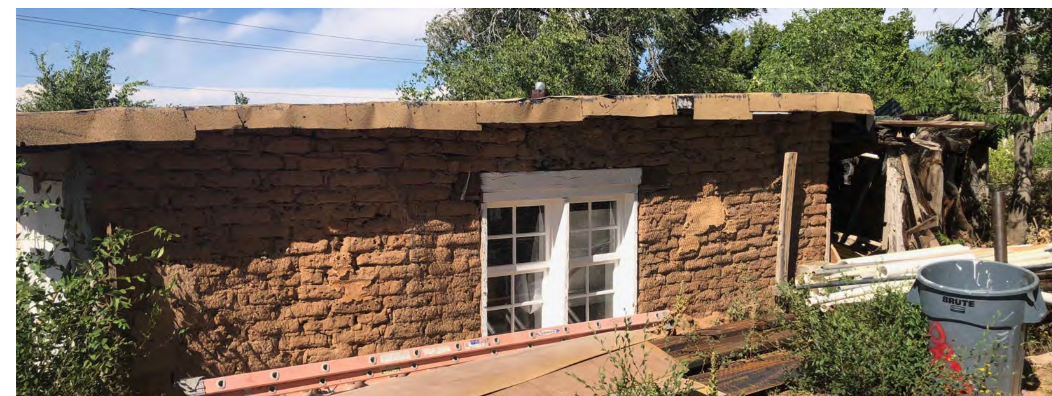
EXISTING REAR BUILDING SOUTH FACADE PHOTOGRAPH
