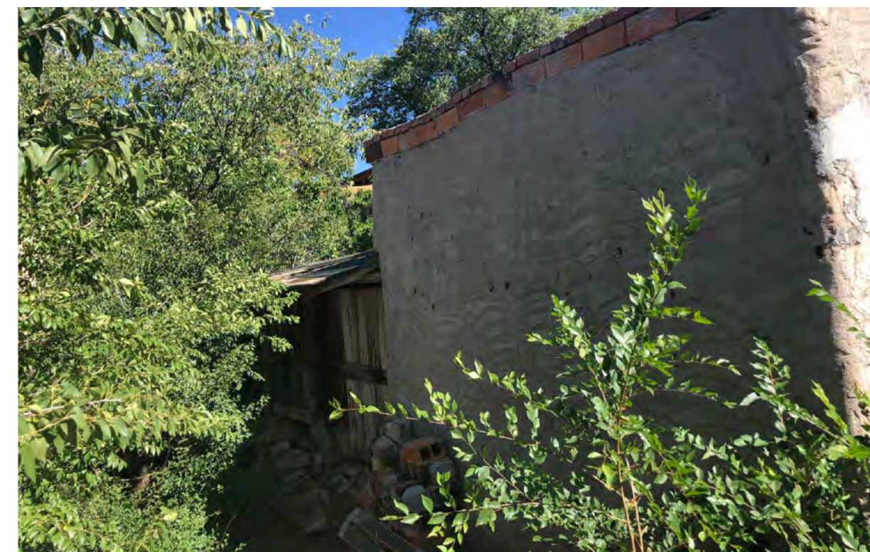
EXISTING REAR BUILDING NORTH FACADE PHOTOGRAPH
