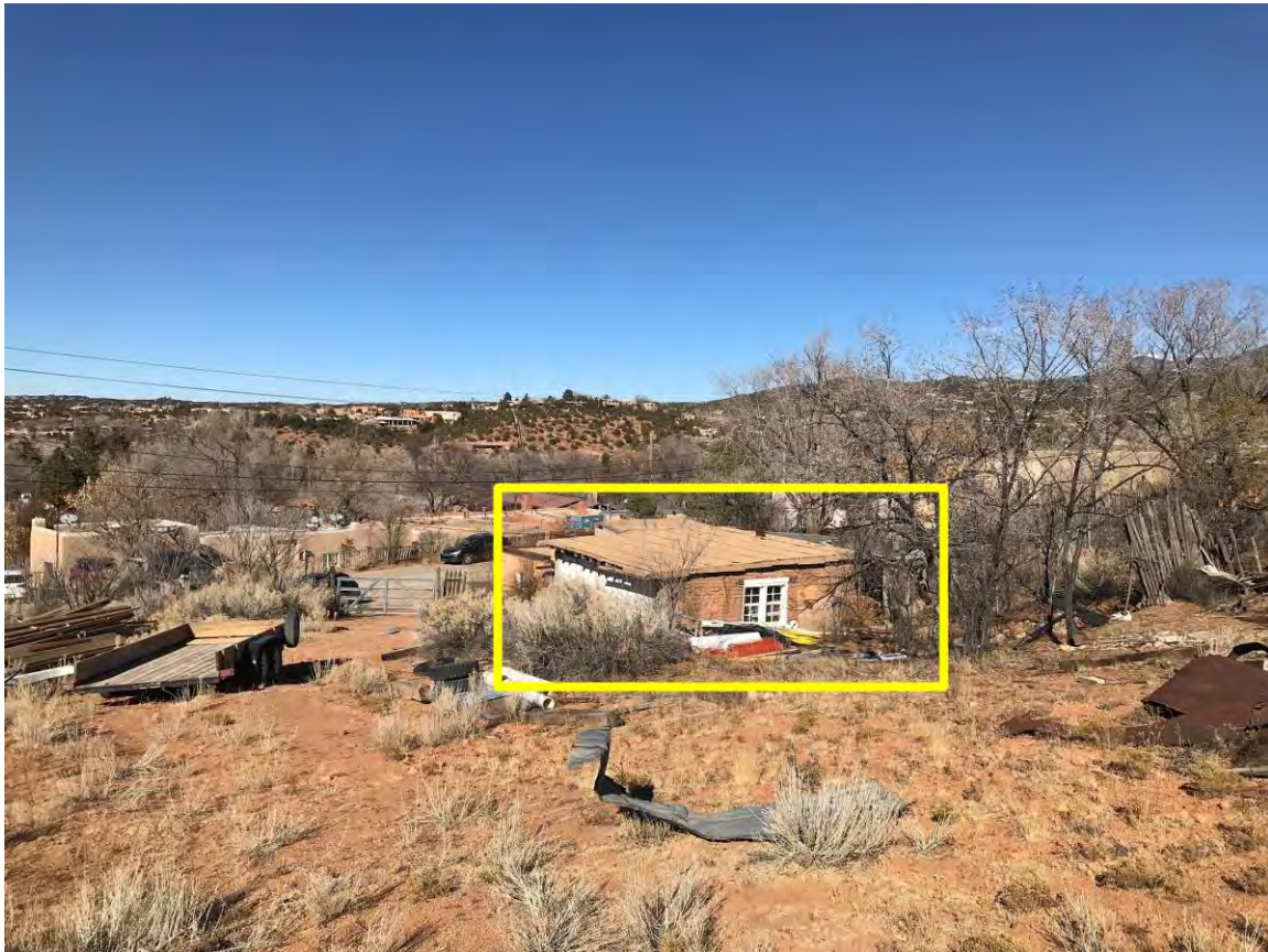
Photo 3: View of Upper Building from south edge of property. Camera facing northeast.
