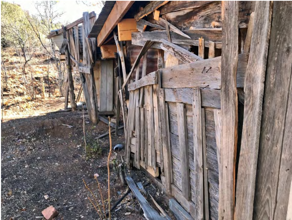
Photo 14: Shed, middle portion. Camera facing south.
