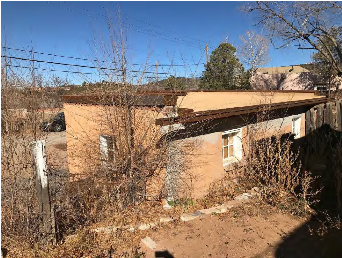
Photo 5: Lower Building, west and south elevations. Camera facing northeast.
