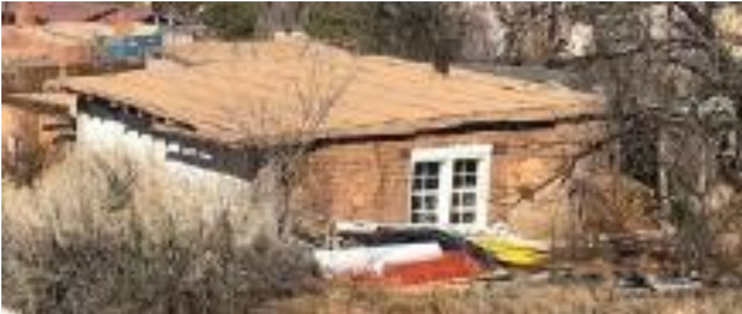
Figure 5: Southern Building South Elevation
