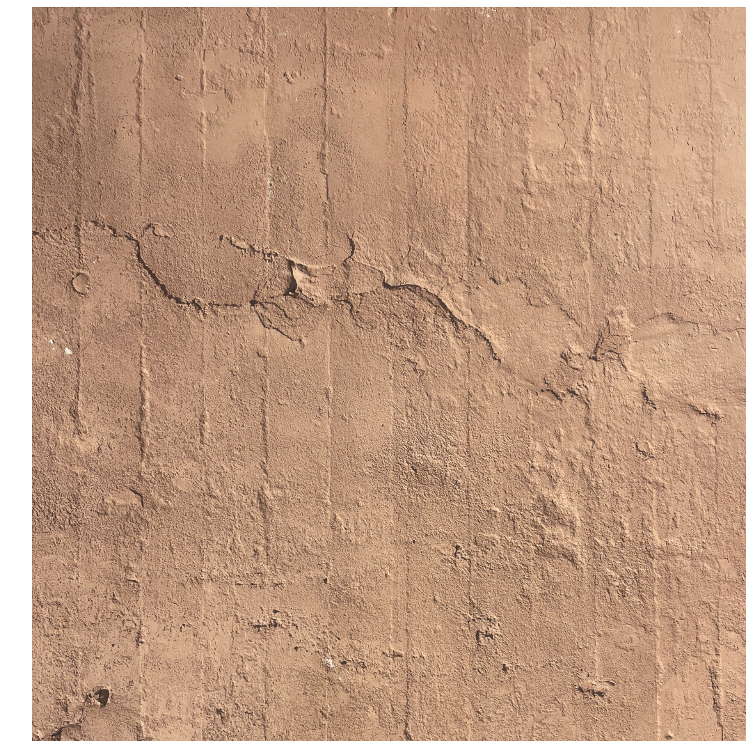
Existing Cast Concrete Retaining Wall
