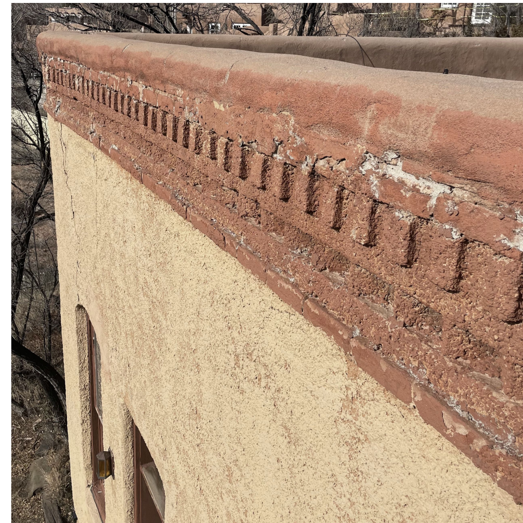
Historic House Existing Coping Repair
