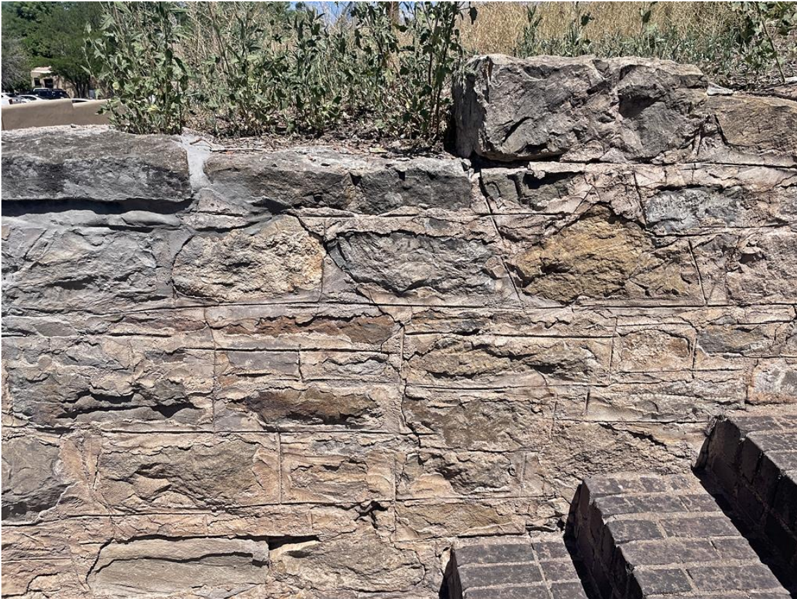
Photo 18: Masonry stairway wall of street entry. Camera facing southwest.
