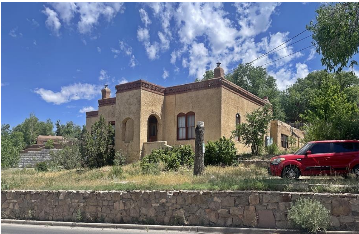
Photo 2: Setting. Camera facing northwest.
