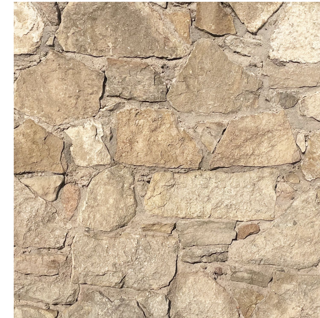
Historic Existing Stone Wall
