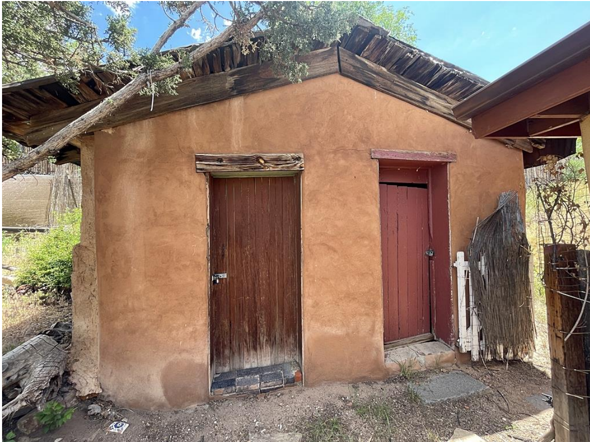
Photo 16: Shed. South elevation. Camera facing northeast.
