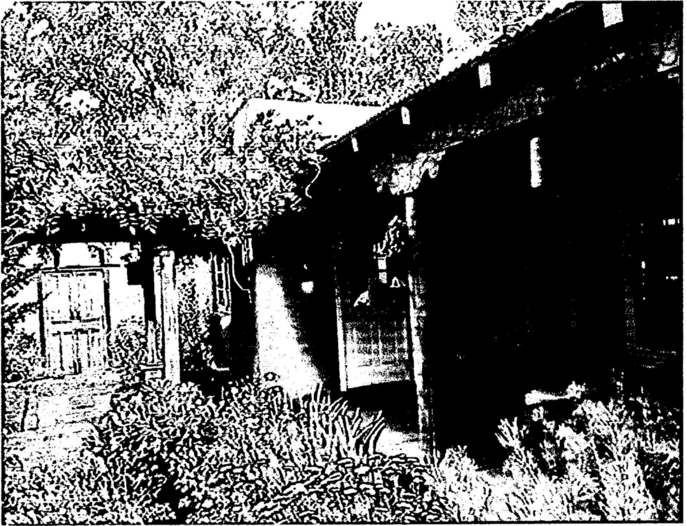
435 ARROYO TENORIO - MAIN HOUSE SOUTH ELEVATION
