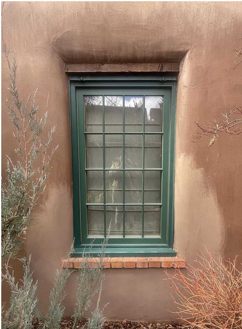
Photo 5: East elevation, window detail. Camera facing west.
