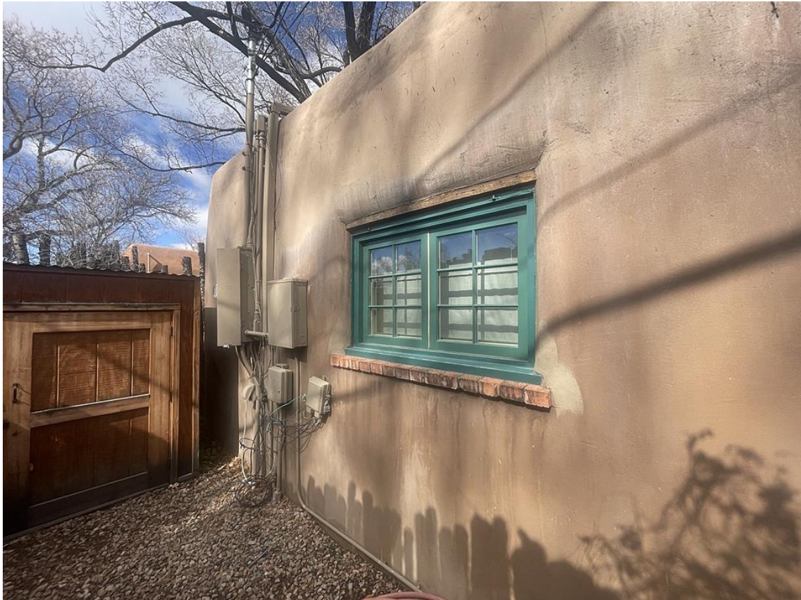
Photo 3: South elevation, oblique. Camera facing northwest.
