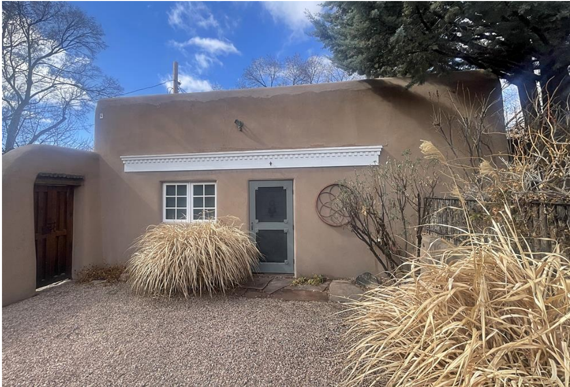
Photo 12: 435 Arroyo Tenorio A, east façade. Camera facing southwest.
