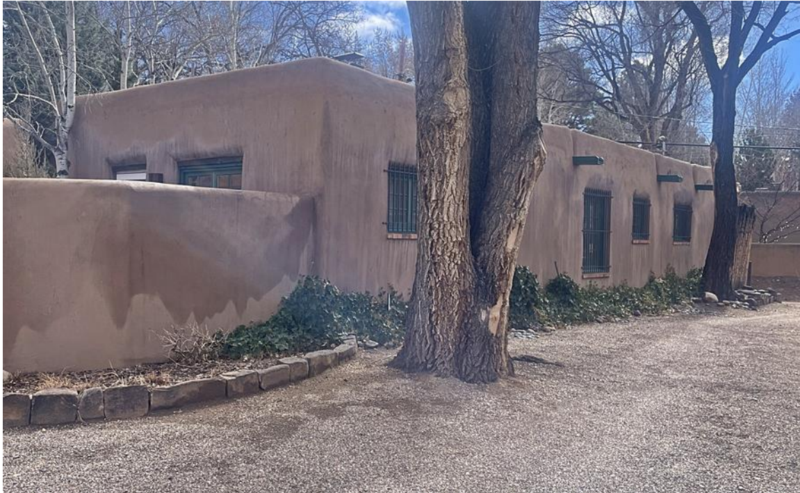
Photo 9: North and west elevations. Camera facing southeast.
