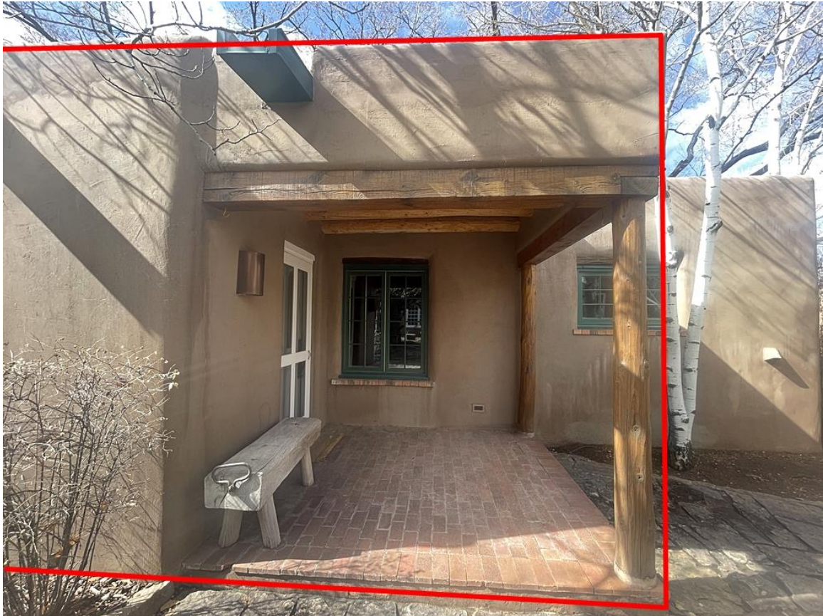
Photo 7: East elevation, c.1994 portal entry addition outlined in red. Camera facing west.
