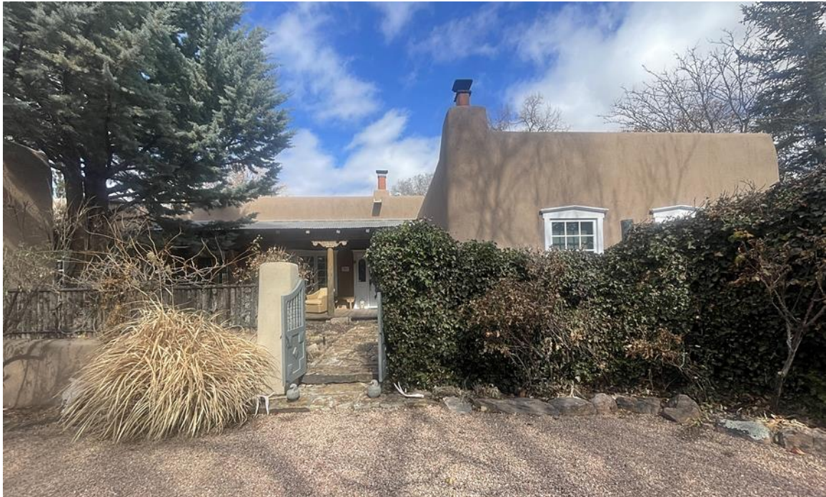
Photo 14: 435 Arroyo Tenorio, south façade. Camera facing north.
