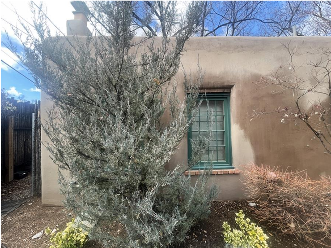
Photo 4: East elevation, south end. Camera facing west.
