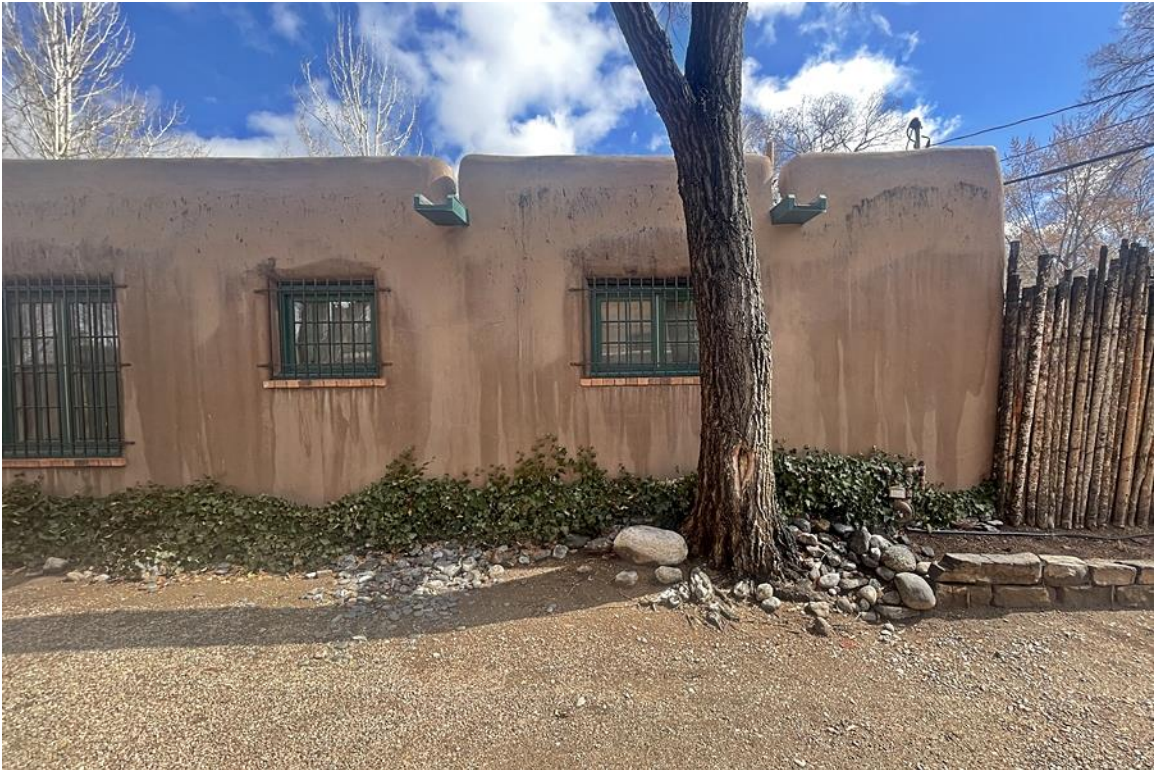
Photo 11: West elevation, south end. Camera facing east.
