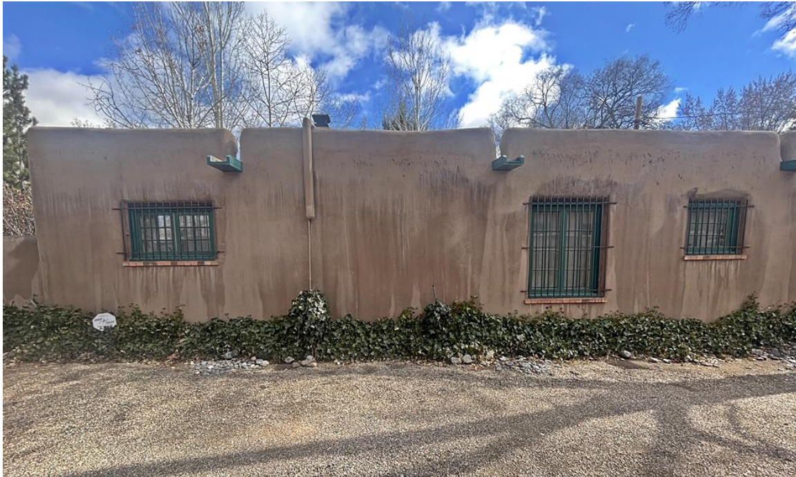
Photo 10: West elevation, north end. Camera facing east.
