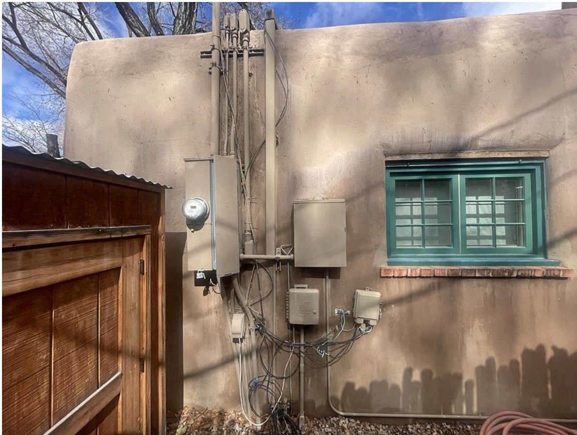
Photo 2: South, west end. Camera facing northwest.
