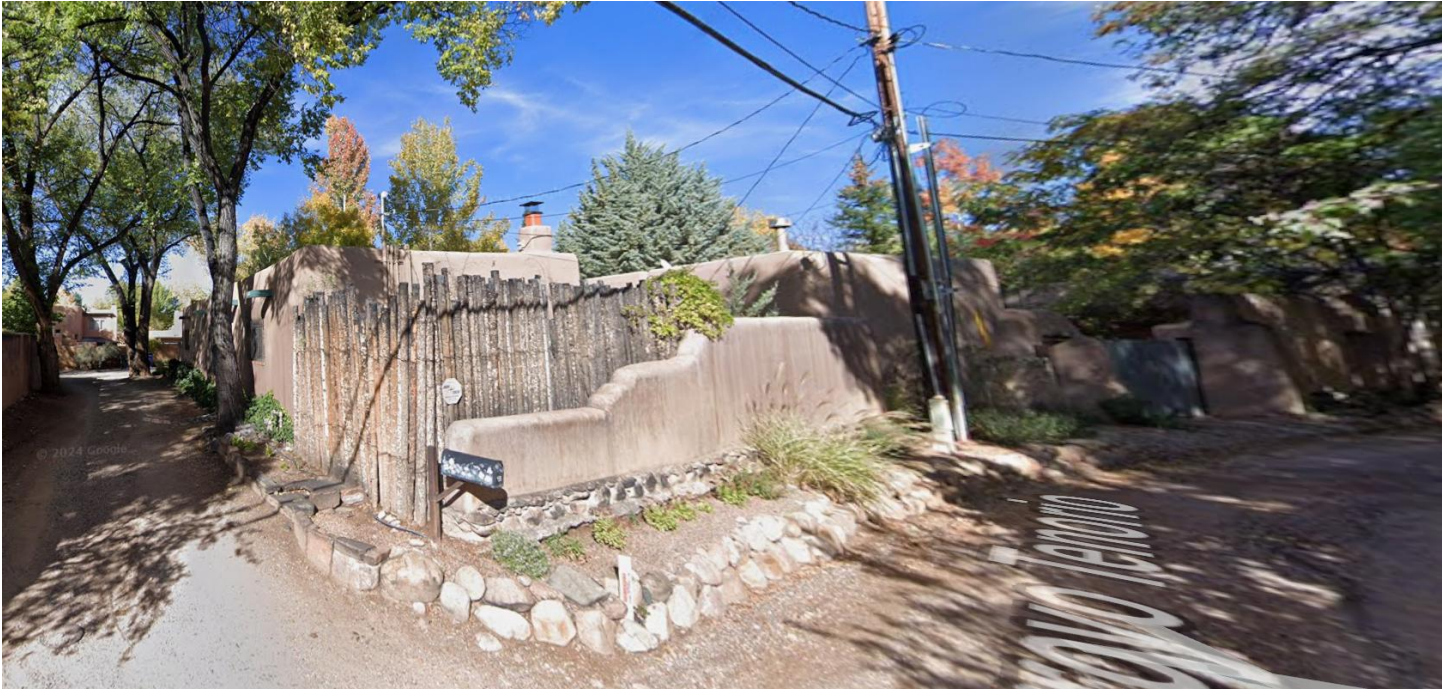
Figure 2: Street Frontage of Subject Property
