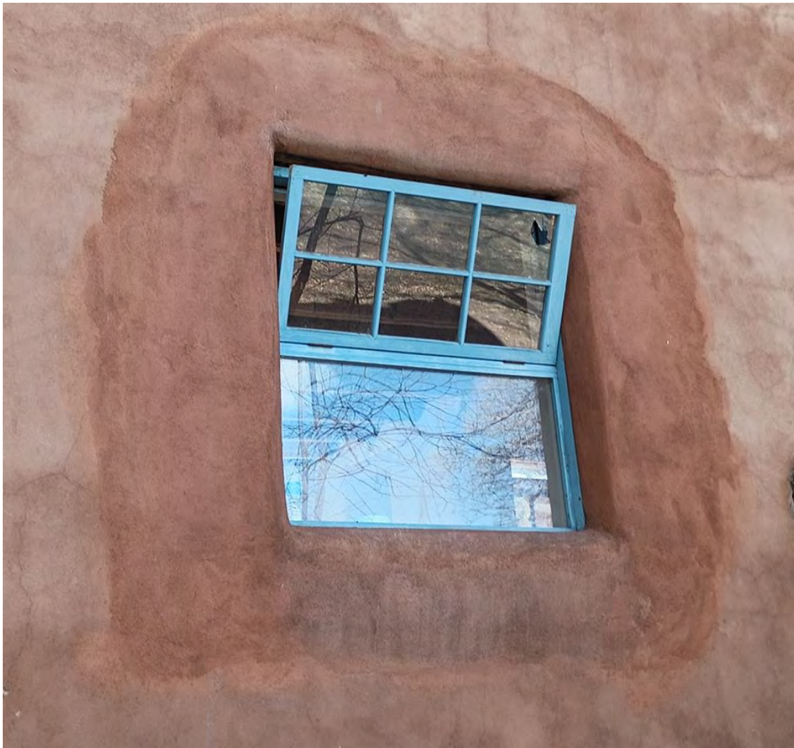
Photo 17: North elevation, typical window. Camera facing up.
