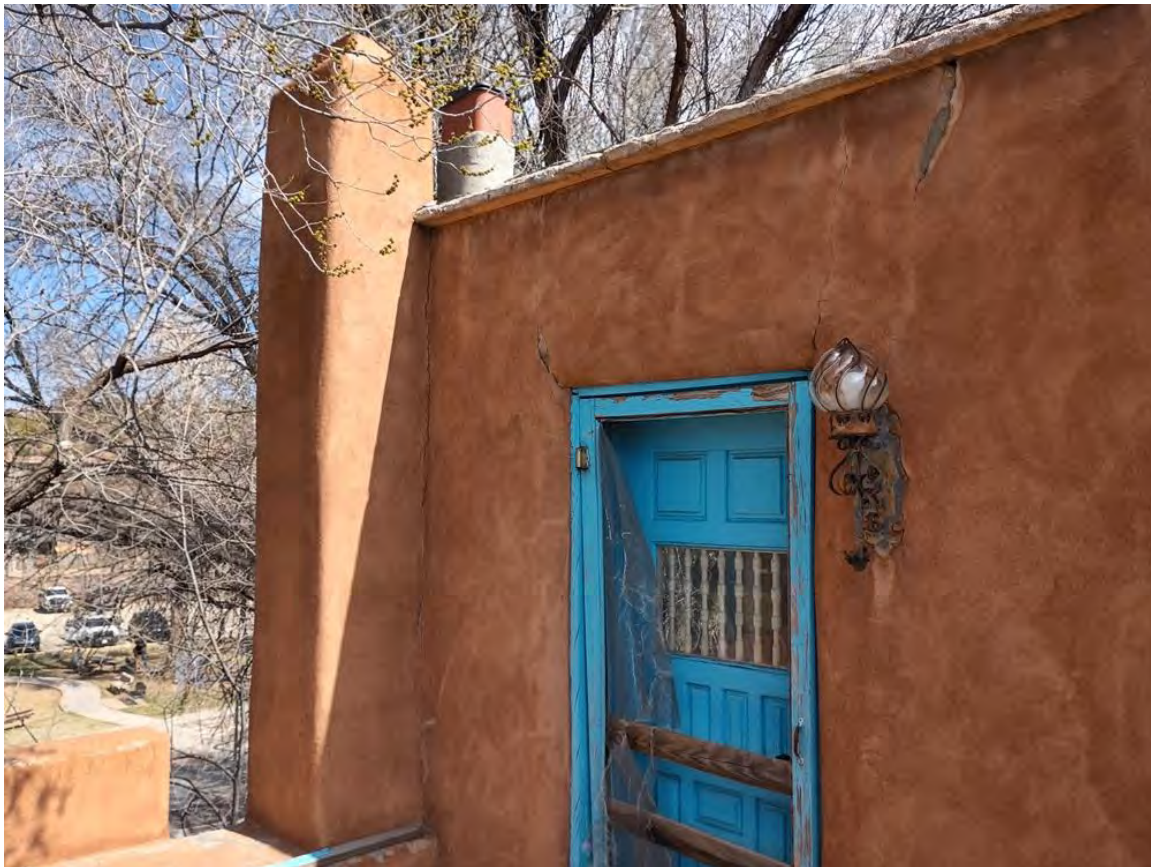
Photo 11: West elevation, second story roof deck entrance. Camera facing northeast.
