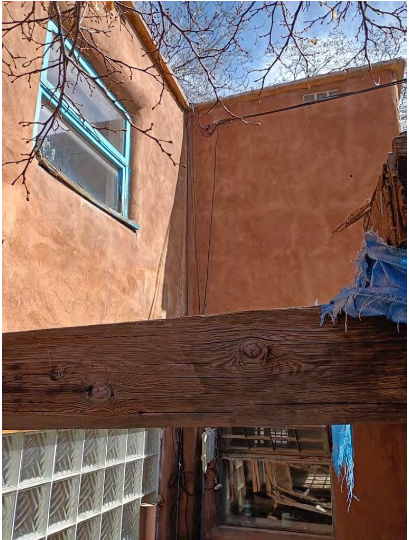
Photo 7: South elevation with stepped back volume. Camera facing up.
