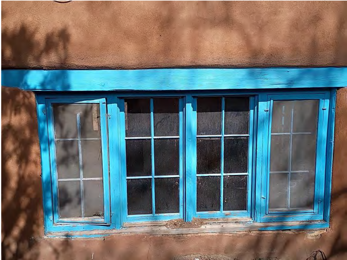
Photo 8: South elevation, ground floor window. Camera facing north.
