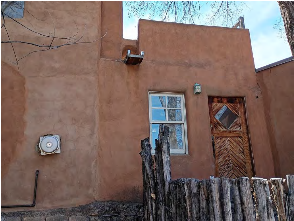
Photo 16: North elevation, addition at west end. Camera facing up.
