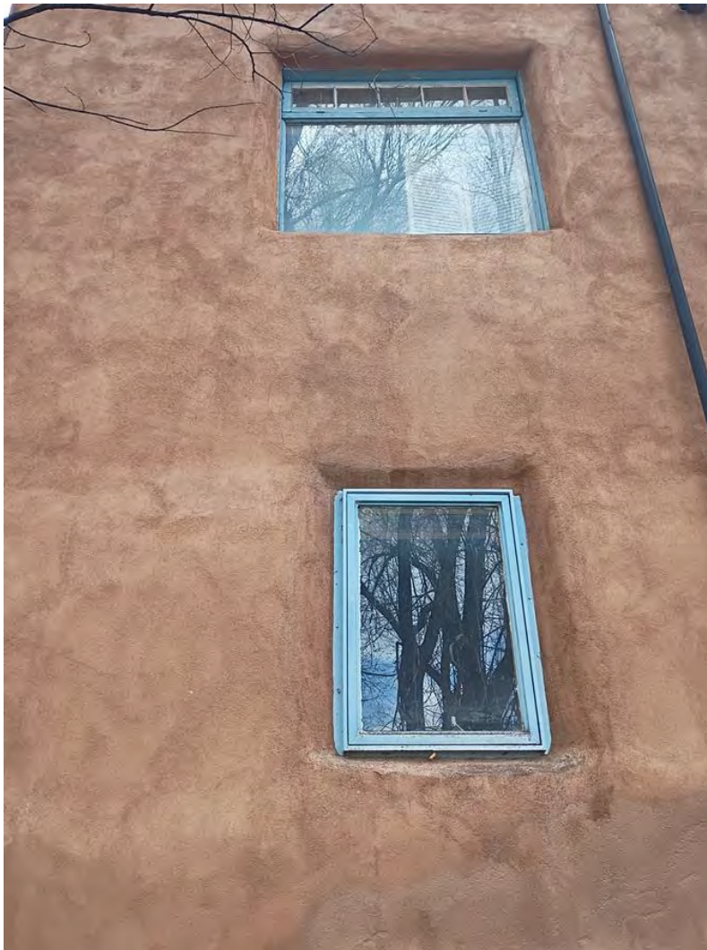
Photo 19: North elevation, east end. Camera facing up.
